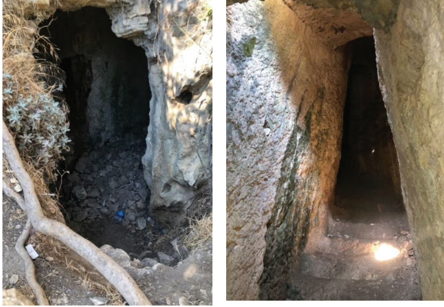
Figure 123. The entrance of the dark tunnel of Alara Castle, 2021
