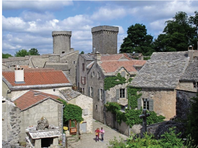
Figure 133. The relation and street pattern of the housing units of the La Couvertoirade (Source: wikimedia.org, 2023)
