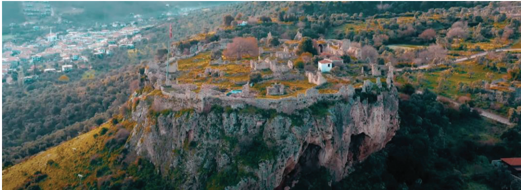
Figure 112. The aerial photo of the inner castle of Beçin (Source: ktb.gov.tr, 2022)
