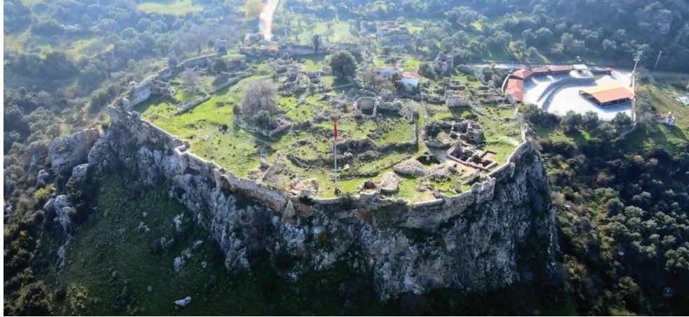
Figure 5. The view of Beçin Castle the plateau from the north direction (Source: Milas Municipality 2019)
