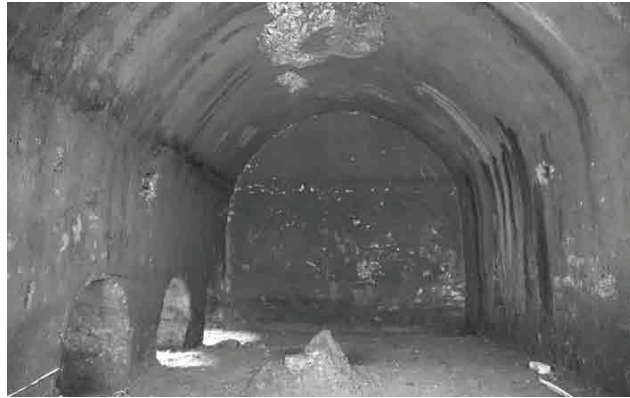
Figure 14. The cistern structure in the Kale Tavas (Source: Beyazıt 2016).
