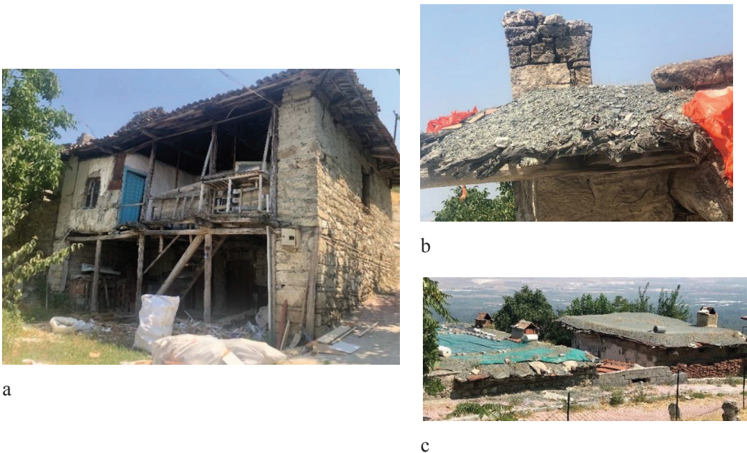
Figure 101. a. The housing units located at the skirt of Honaz Castle, 2020, b. The housing units have terrace roof with earth covering, 2020, c. The housing units with hipped roof located at the skirt of Honaz Castle 2020.
