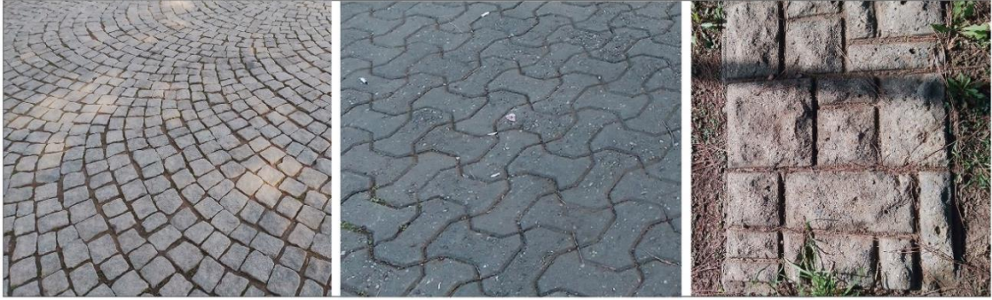
Figure 5. 20. Pavement materials in the Hıfzı Veldet Velidedeoğlu Park (Source: Prepared by the author)
