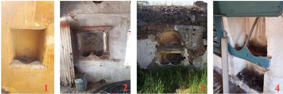
F. 12: 1: Single jug niche in H9. 2: Double jug niche in H6. 3: Double jug niche with another niche on top in H4. 4: Double jug niche with another niche under it in H5. (Photos by Saribekiroğlu, 2017)
