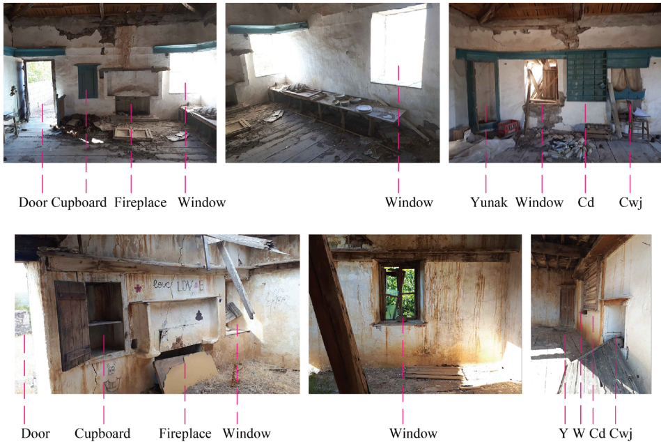
F. 4: Living spaces of H5 and H14 at first level. Above photos belong to H5 and below ones to H14. Left: West walls. Middle: North walls. Right: South walls. Y: yunak. W: window. Cd: cupboard for dishware. Cwj: cupboard for water jugs (Photos by Saribekiroğlu, 2017; prepared by Saribekiroğlu, 2022)
