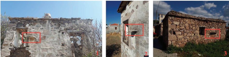
F. 15: 1: Exterior shelf in H3. 2: Exterior shelf in H5. 3: Exterior shelf in H13. (Photos by Sarıbekiroğlu, 2017)
