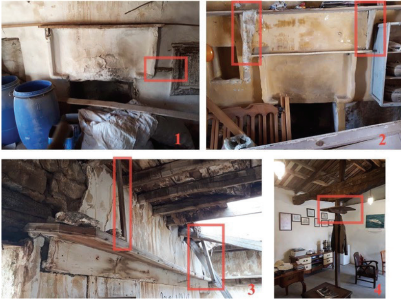
F. 14: 1: Small wooden shelf at ocak kulağı level in H6. 2: High level shelf supported below in H9. 3: High level shelf suspended to beams in H14. 4: Direk başı in H7. (Photos by Sarıbekiroğlu, 2017)
