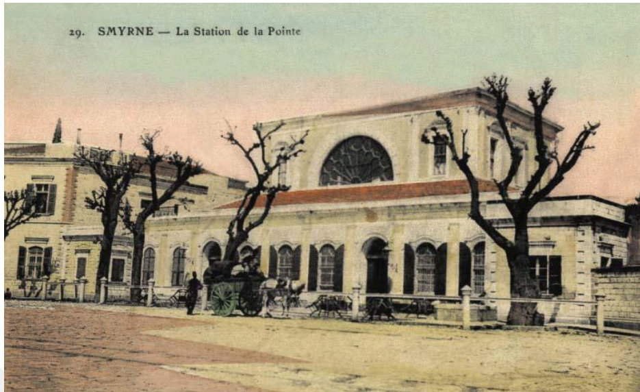
Figure 86. Photo of Alsancak Station (Source: SALT Rsearch)
