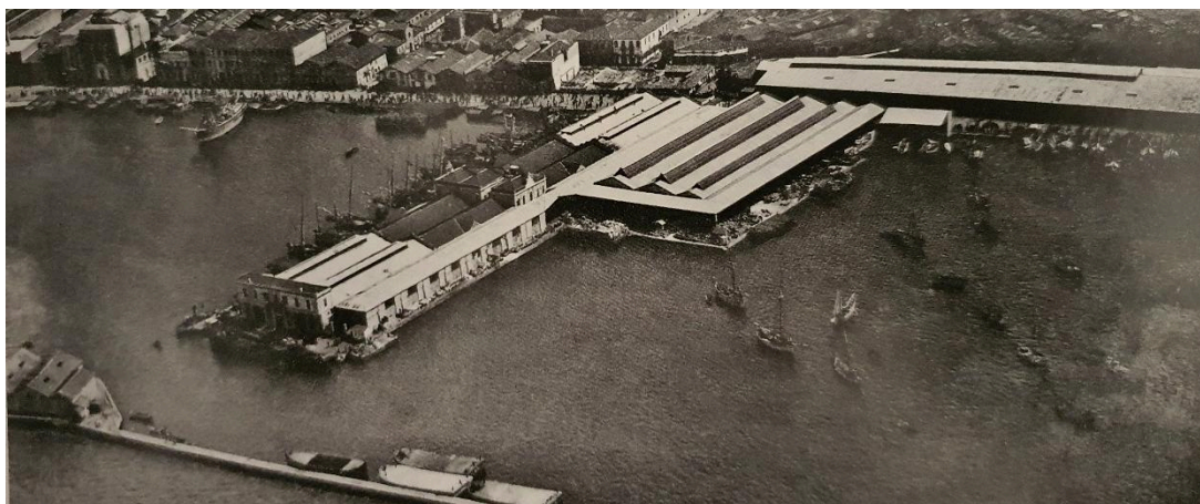
Figure 66. Aerial Photography of Pier (Source: Collection of Poulimenos)
