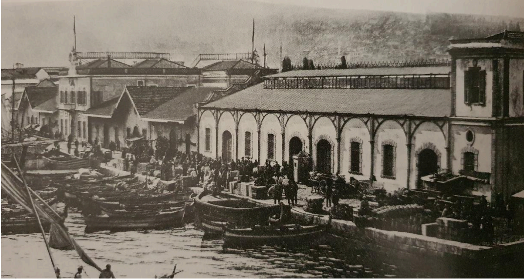
Figure 67. Photo of Pier (Source: APİKAM)
