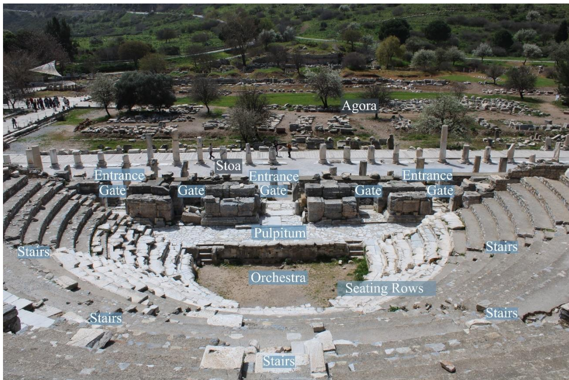
Figure 4.8. Parts of the Ephesus Bouleuterion/Odeion seen when looking from the north direction to the south direction (Photograph: T. Tekin, 03.04.2022).
