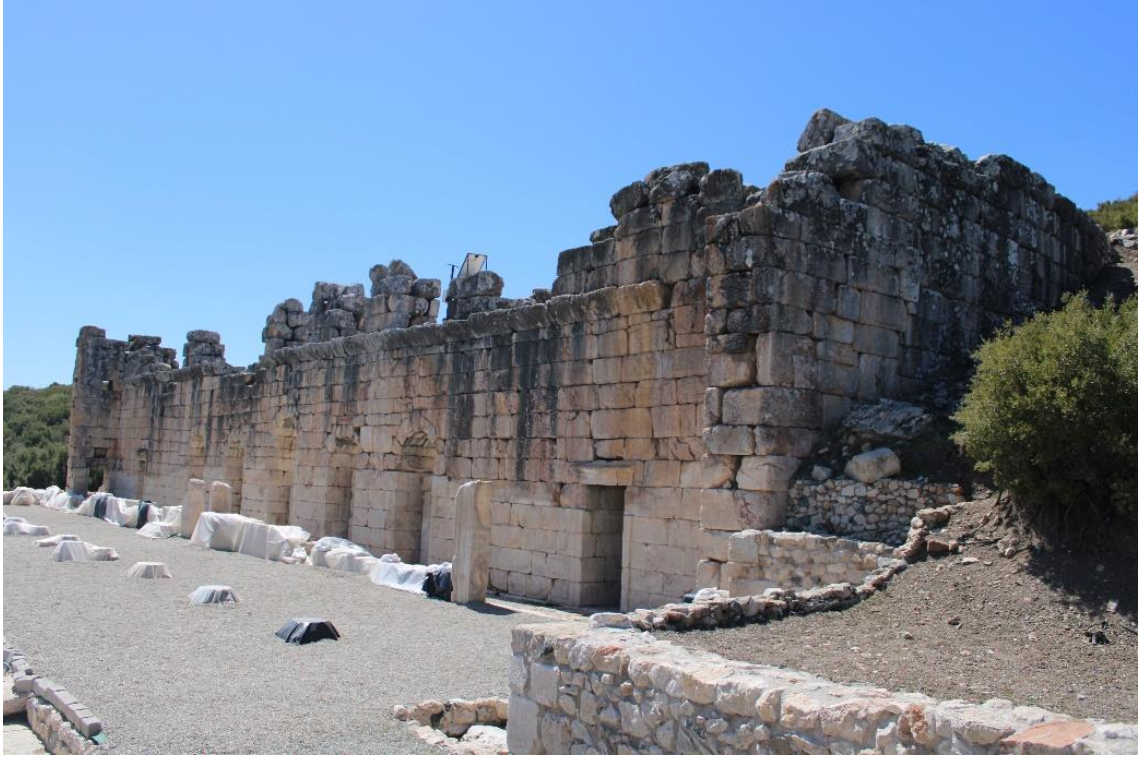
Figure 2.13. View of the Kibyra Bouleuterion from the northeast direction (Photograph: T. Tekin, 09.04.2022).
