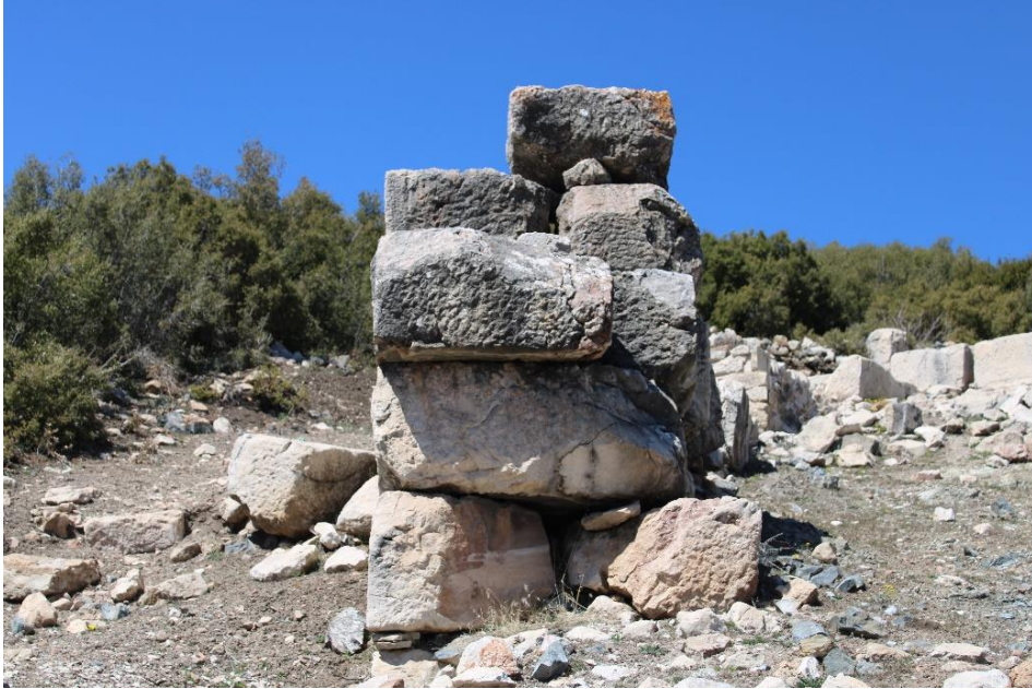
Figure 4.88. Retaining wall masonry in the southwest section of the bouleterion which is surrounding the cavea with curvilinear form (Photograph: T. Tekin, 09.04.2022).
