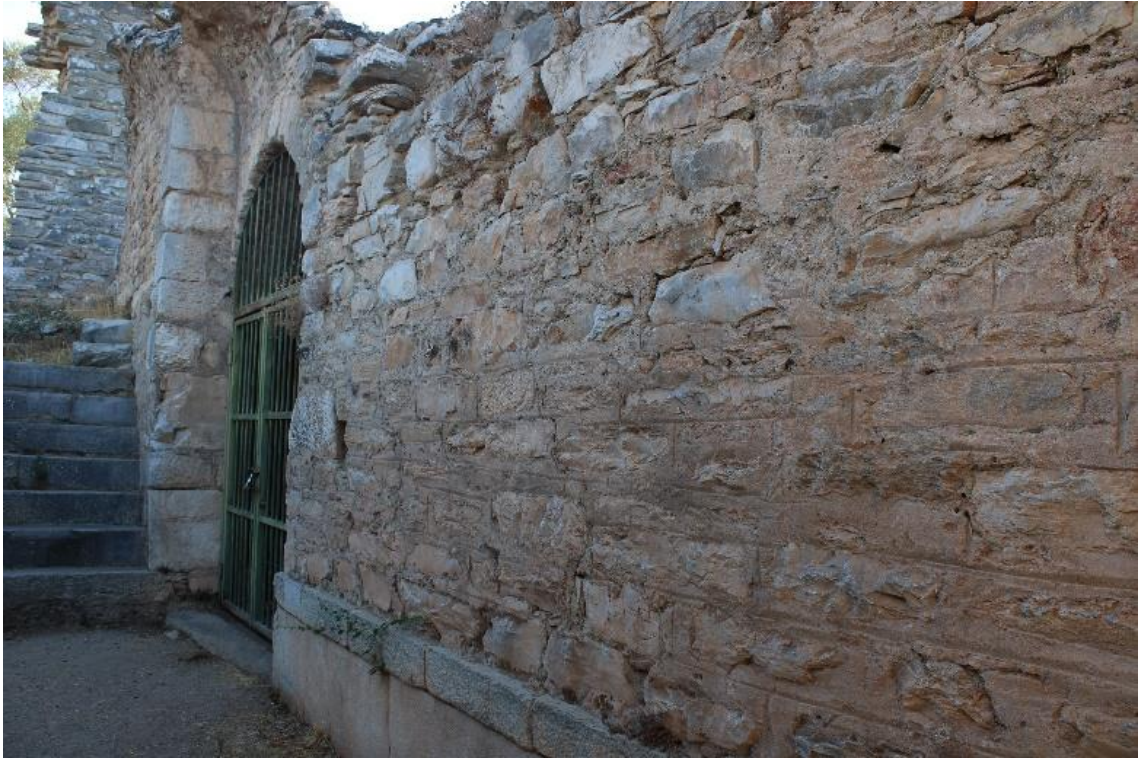
Figure 4.53. Consolidated east inner wall of the west corridor (Photograph: T. Tekin, 05.09.2021).
