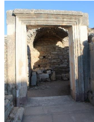
Figure 4.48. Completed door opening with using materials which are different from the original stone block material. After implementation(a) and today's state(b) (Source of a: Levi 1986, Figure 37, 1986; Photograph of b: T. Tekin, 05.09.2021).
