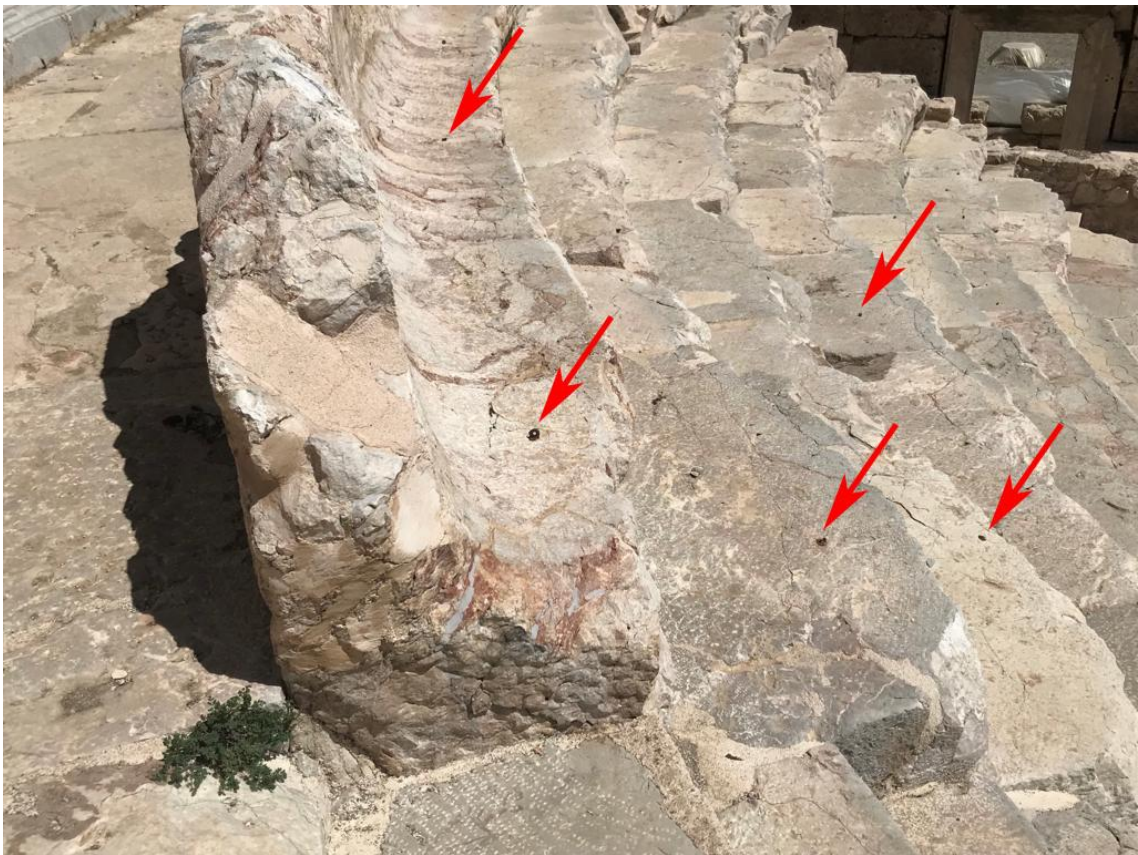
Figure 2.20. Fastener ruins on the seating rows of Kibyra Bouleuterion (Photograph: T. Tekin, 09.04.2022).
