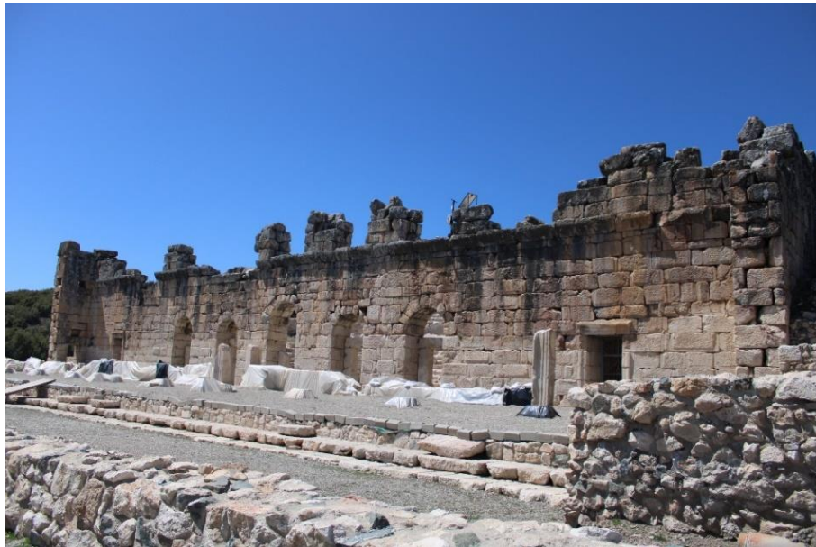
Figure 4.108. The east side of the scene wall of the Kibyra Bouleuterion (Photograph: T. Tekin, 09.04.2022).
