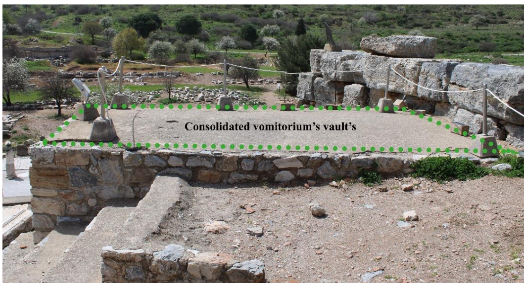
Figure 4.22. Concrete implementation on the western vomitorium vault (Photograph: T. Tekin, 03.04.2022).
