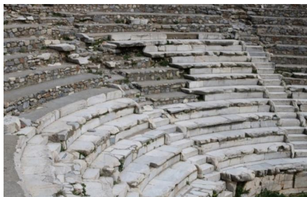
Figure 2.17. Ima cavea section of the Ephesus Bouleuterion/Odeion built of stone blocks and the reconstructed rubble filling under the seating rows (Photograph: T. Tekin, 03.04.2022).
