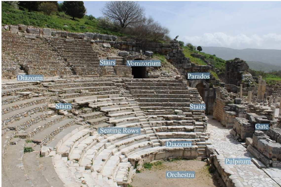
Figure 4.9. A portion of the parts of the Ephesus Bouleuterion/Odeion seen when looking from the west direction to the east direction (Photograph: T. Tekin, 03.04.2022).
