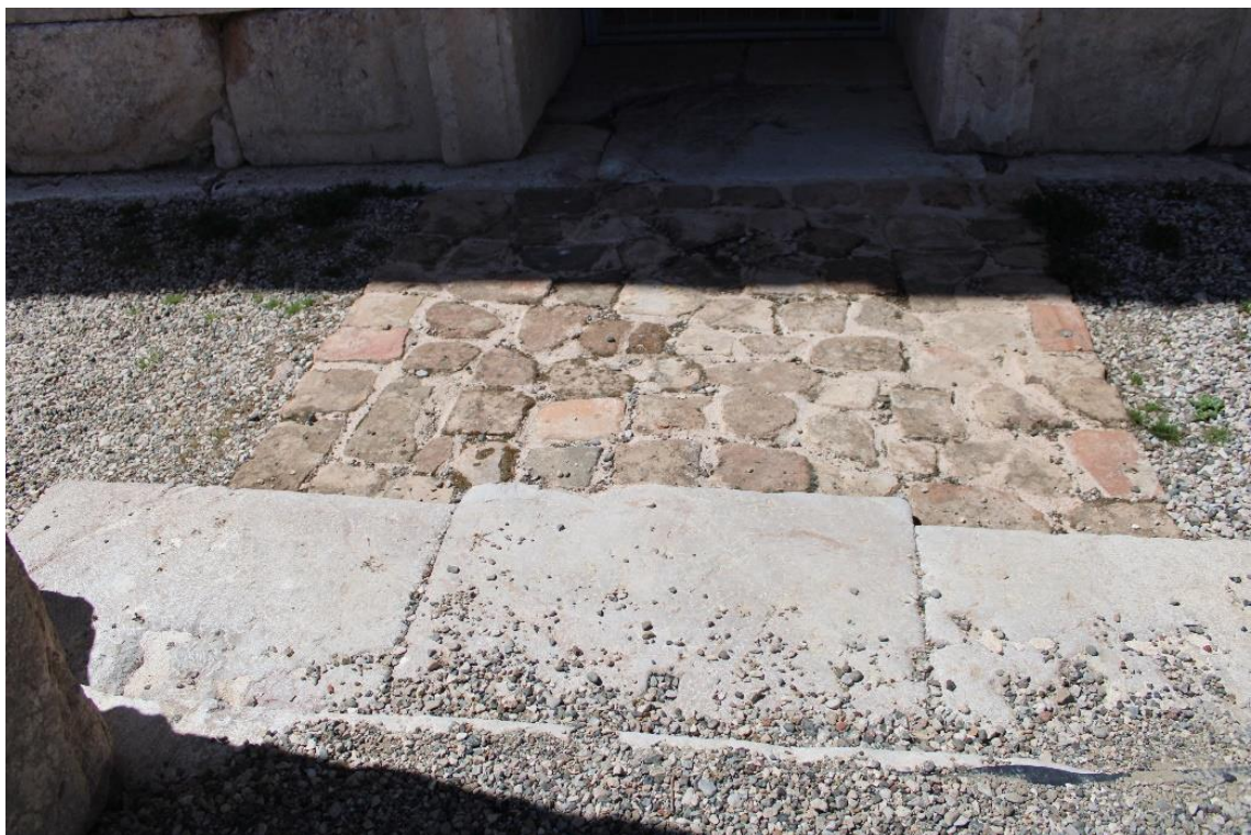
Figure 4.105. Reconstructed part using rubble stone and mortar between the scene wall and stoa (Photograph: T. Tekin, 09.04.2022).
