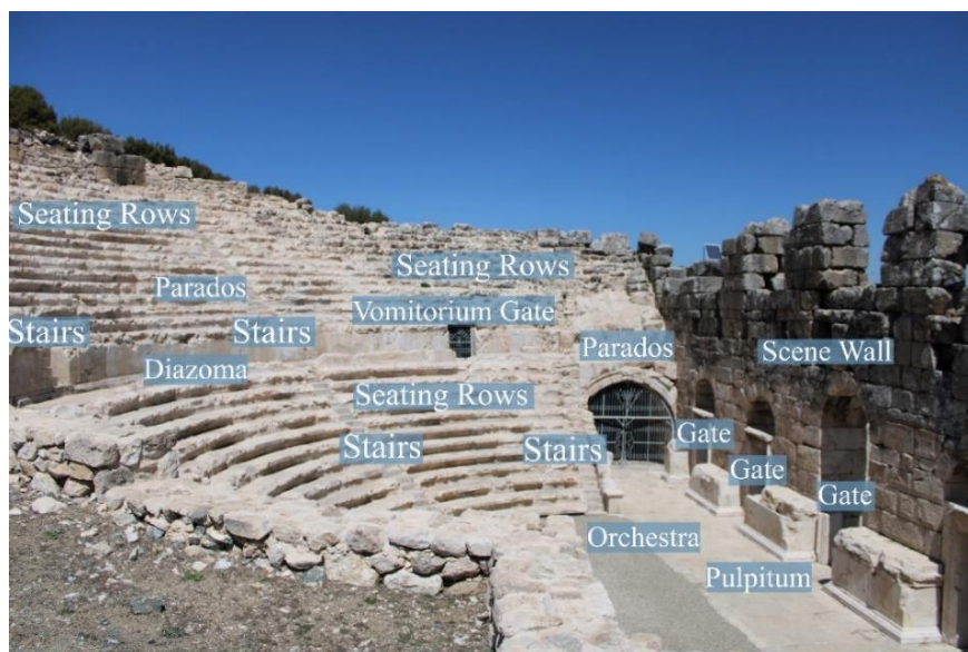
Figure 4.86. The view of some parts of the Kibyra Bouleuterion/Odeion from south (Photograph: T. Tekin, 09.04.2022).
