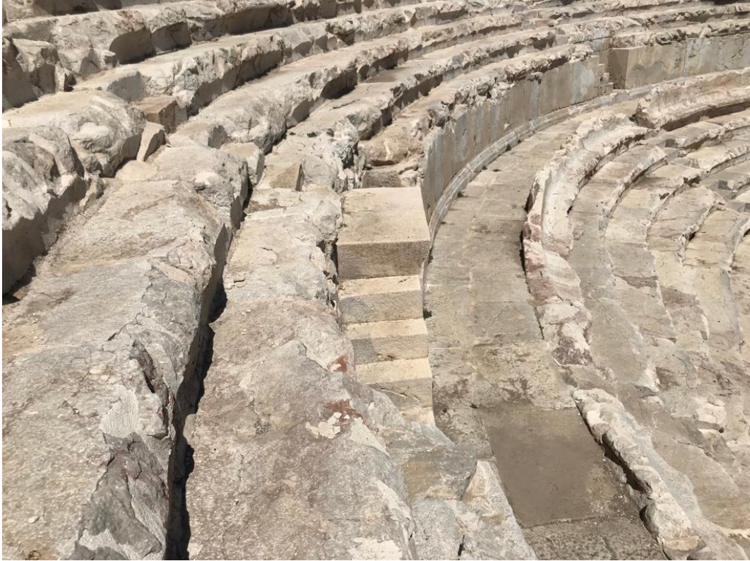
Figure 4.97. Completed and partially reconstructed stairs and seating rows (Photograph: T. Tekin, 09.04.2022).
