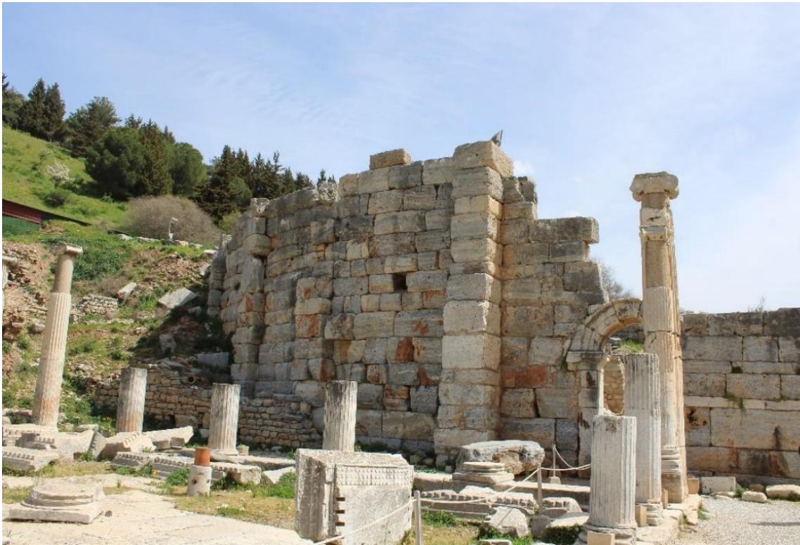
Figure 4.10. View of the curvilinear exterior wall on the west side of the Ephesus Bouleuterion/Odeion, the buttresses supporting the wall, and the arched gateway (Photograph: T. Tekin, 03.04.2022).
