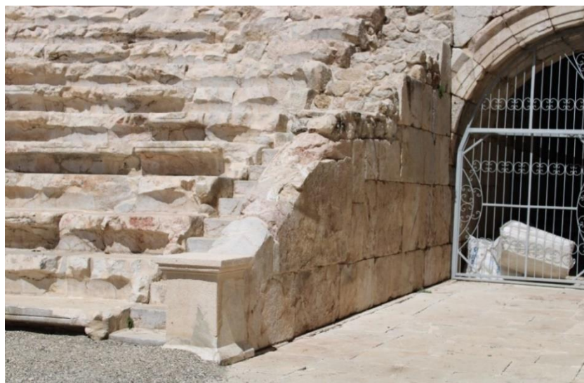
Figure 4.100. Reconstructed part at the beginning of the north analemma wall (Photograph: T. Tekin, 09.04.2022).
