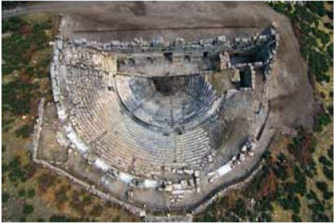
Figure 4.94. Aerial photograph of the bouleuterion after excavation (Source: Özüdoğru and Dökü 2010, p.39 Figure:4).
