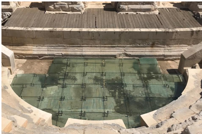
Figure 4.78. Orchestra flooring with added glass platform (Photograph: T. Tekin, 08.04.2021).
