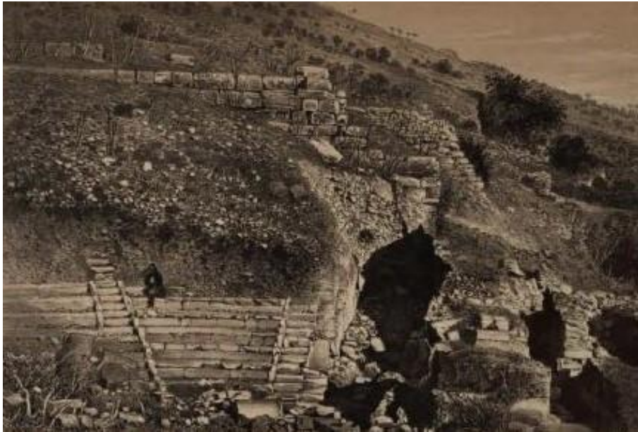
Figure 4.13. View from west to east of the structure before the excavation and conservation works (Source: Wood 1877).
