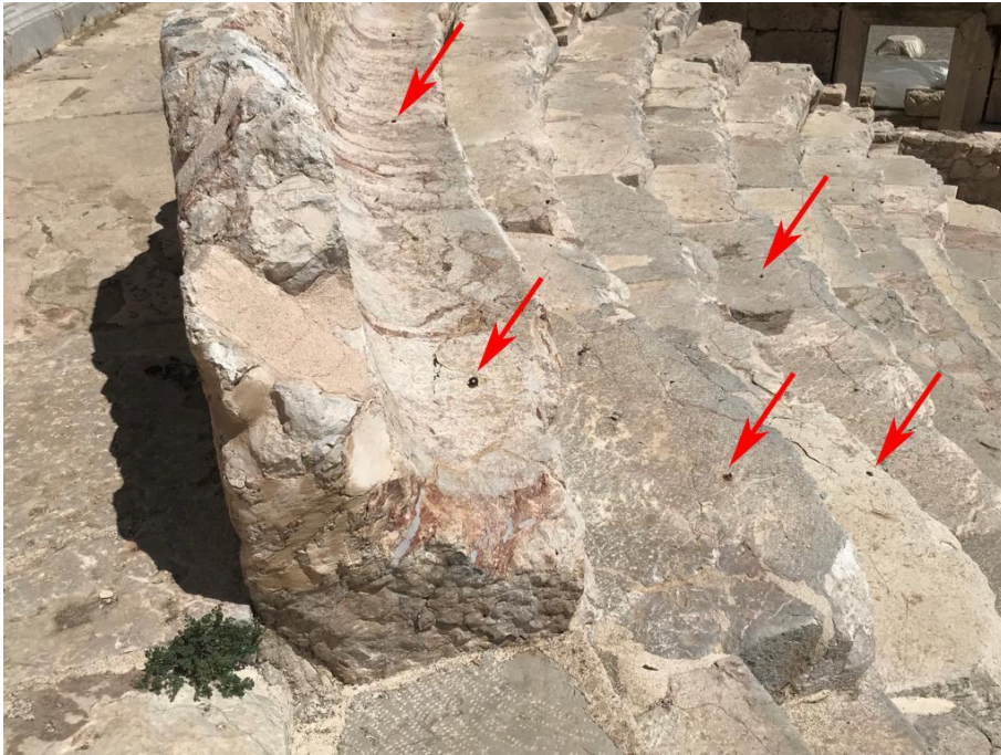
Figure 4.90. Fastener remains on the seating rows (Photograph: T. Tekin, 09.04.2022).
