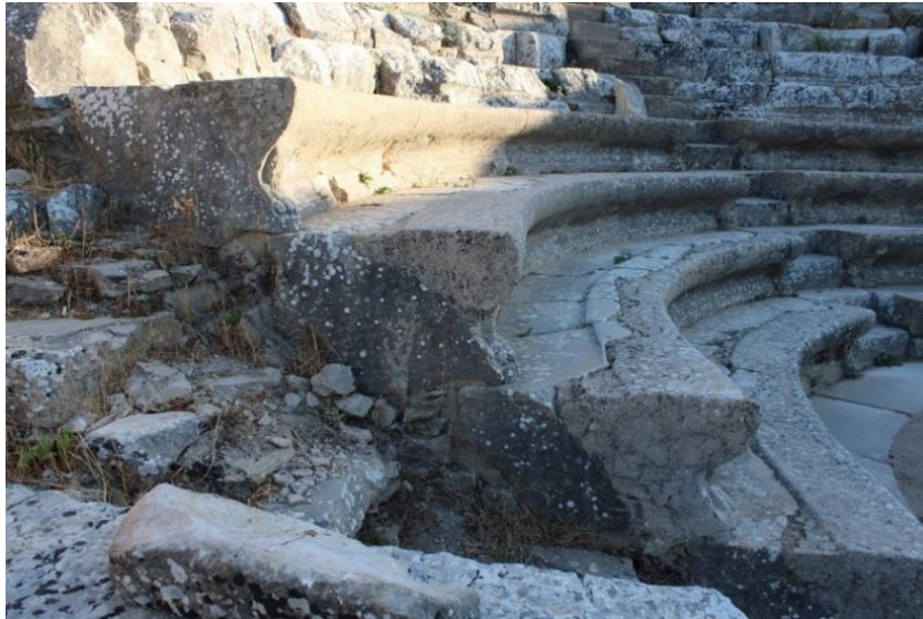
Figure 4.50. Completed seating rows by using concrete (Photograph: T. Tekin, 05.09.2021).
