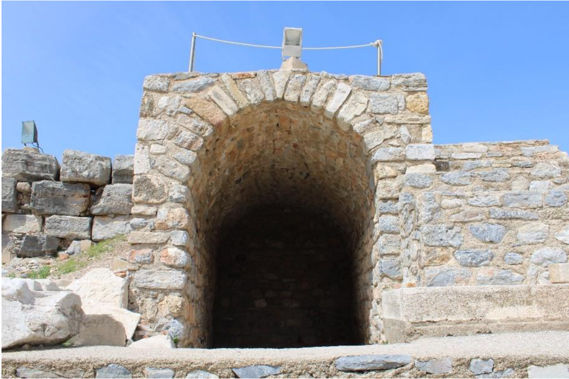
Figure 4.29. Reconstructed and completed vault of the western vomitorium (Photograph: T. Tekin, 03.04.2022).
