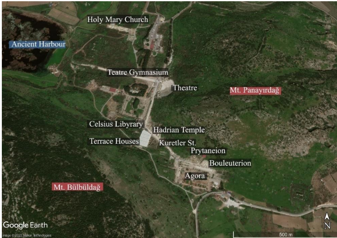
Figure 4.3. Aerial photograph showing the Ephesus Bouleuterion/Odeion and the surrounding structures (Revised from Google Earth, date of image: 21.02.2021 date of editing: 29.09.2022).
