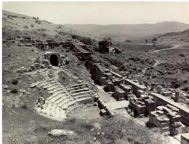
Figure 4.15. Reconstruction of the vomitorium, completion of the pulpitum and capping on the masonry on the south direction, 1964 (Source: Salt Research, 2022, Photograph: Laroche 1964).
