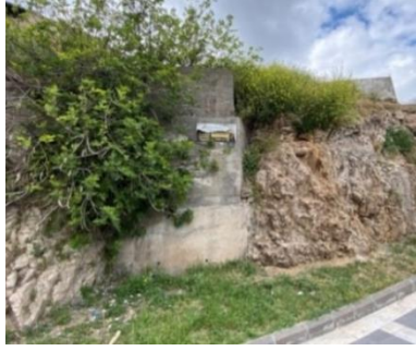
Figure 4.77. The retaining wall adjacent to Yeni Mahalle Tell (2021, April 11).
