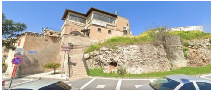
Figure 4.79. The stairs constructed on the tell and connected two streets each other. (Source: Google Earth, 2021)
