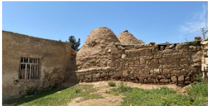
Figure 4.38. The traditional and dome of vernacular house which are plastered with adobe (2021, April 16).
