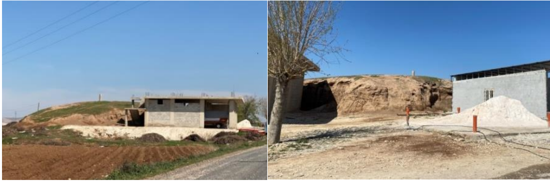
Figure 5.3. The modern buildings constructed in violation of registration decision (2021, 14 April).
