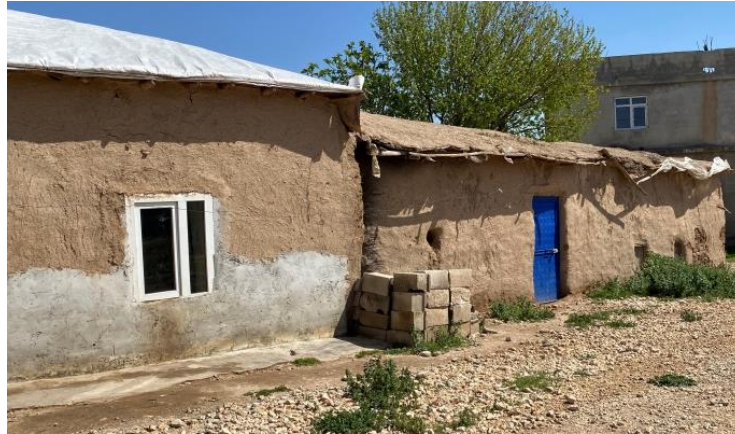
Figure 4.22. The traditional houses repaired with modern materials (2021, April 14).
