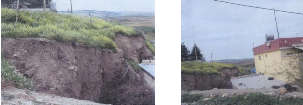
Figure 4.69. An excavation work conducted on Yaylak Tell for the construction of a modern house.
