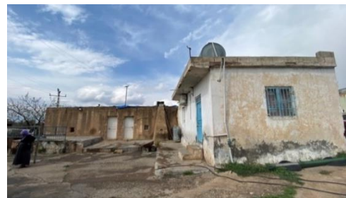
Figure 4.13. A traditional dwelling plastered with cement (right), and an original traditional building used as a warehouse (left) (2021, April 12).
