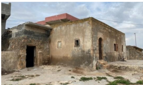
Figure 4.12. A modern addition to a traditional building (left), and a traditional building plastered with cement (right) (2021, April 12).
