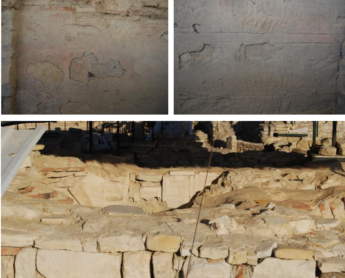
Figure 3.13. Horizontal and vertical ornaments on brick-lime plaster
