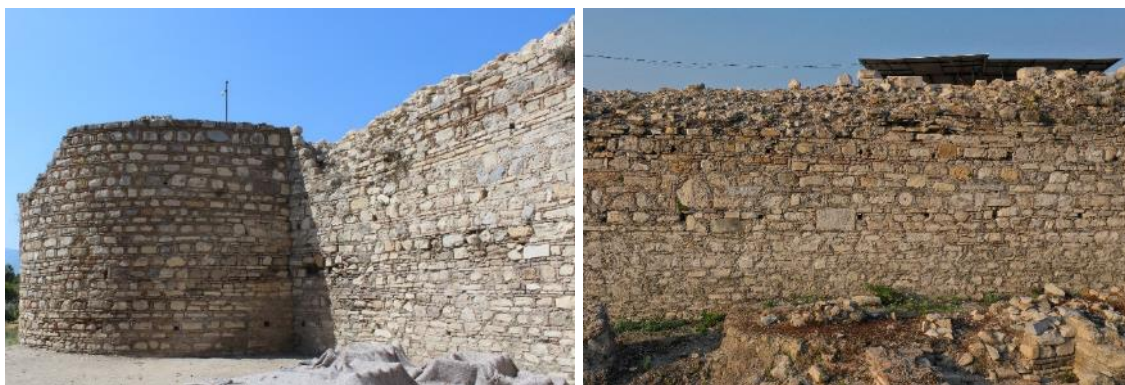
Figure 3.12. Kadıkalesi fortification wall
