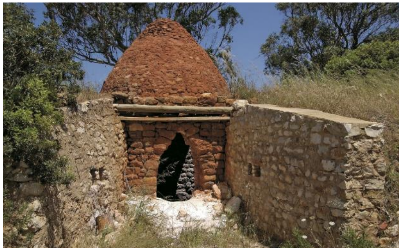
Figure 2.1. Restorated lime kiln in AlmaVerde (Source: Tranmer 2015)
