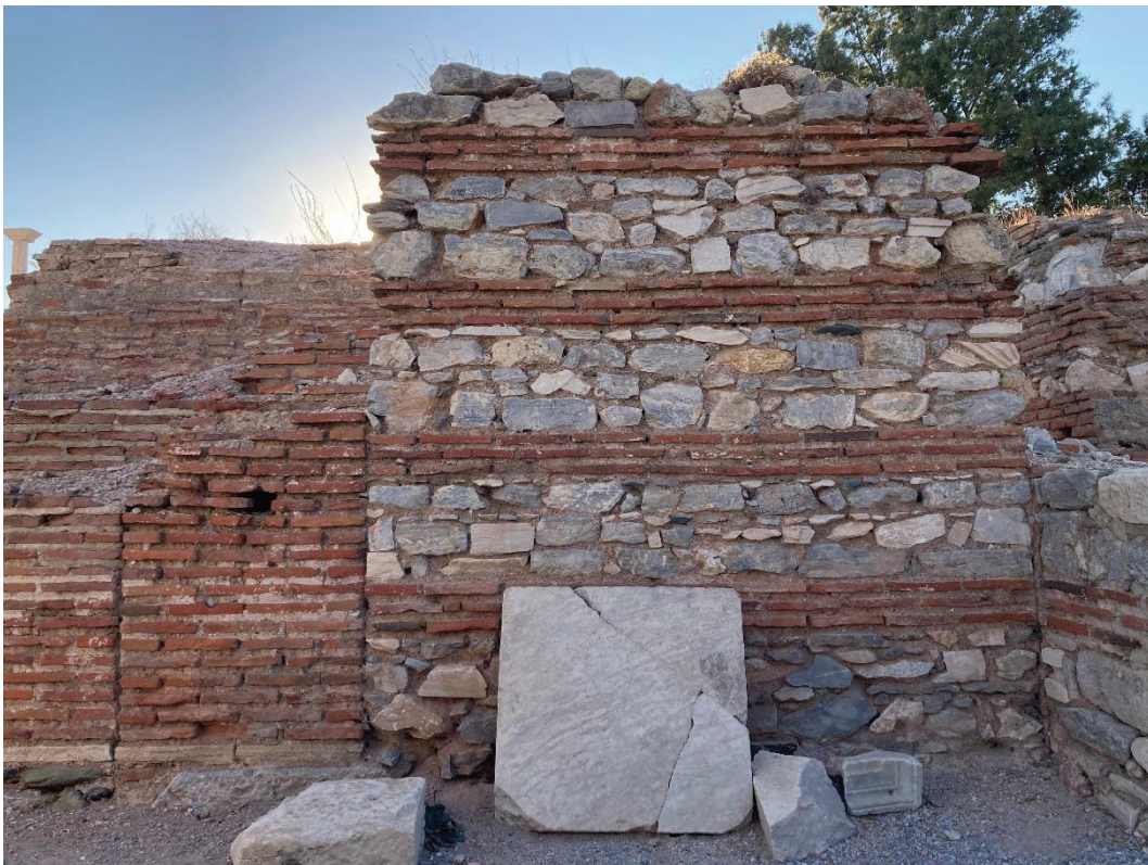
Figure 3.9. Different wall bonding types from the northern transept (Right side of the wall was a part of 1 st phase, and the left side was built in later periods)
