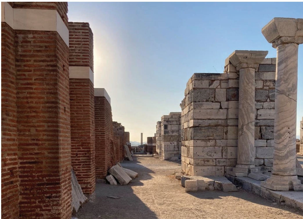
Figure 3.7. Photo of southern nave with outer brick wall on the left and stone columns and pillars on the right
