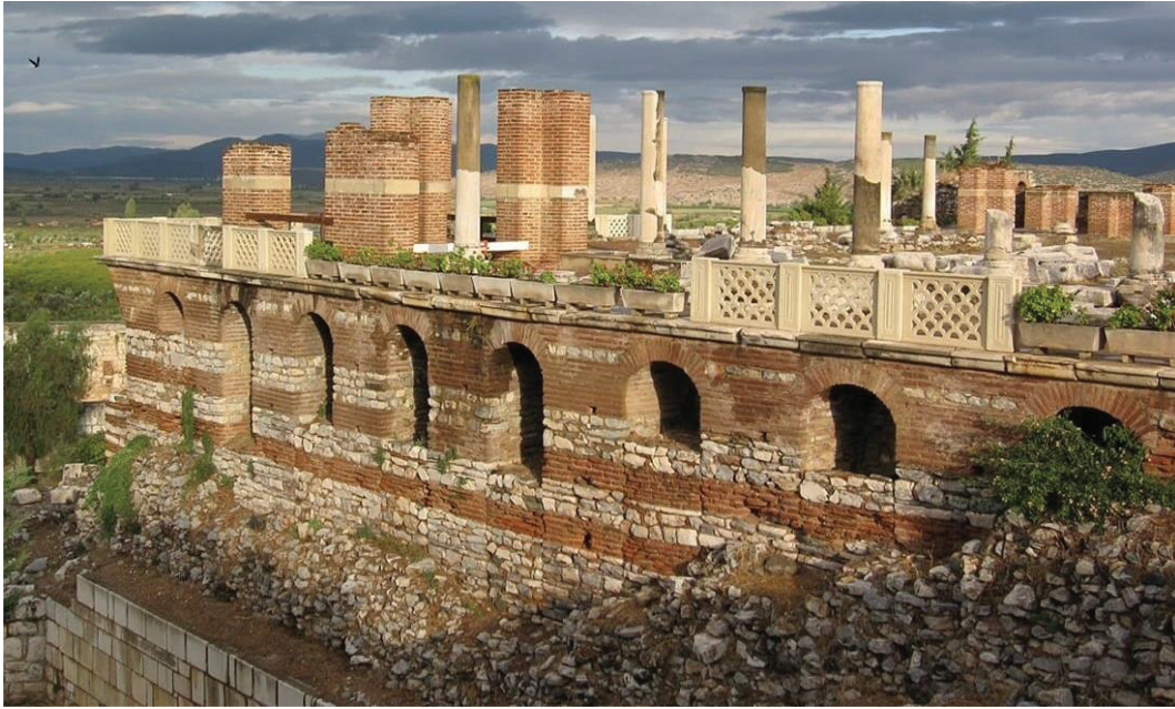
Figure 3.8. Photo of the exterior walls of substructure and the atrium built on top of it (Source: Büyükkolancı 2018, 24–25)
