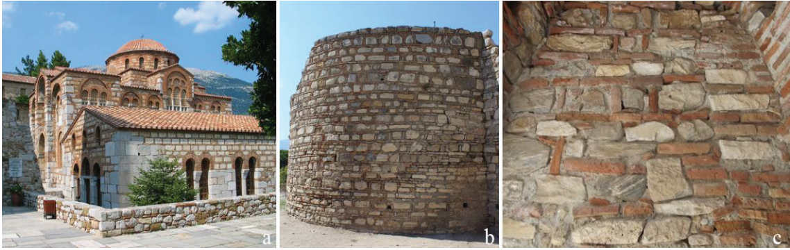
Figure 2.3. Examples of cloisonne technique, a: Monasteries of Daphni, Greece (Source: “Monasteries of Daphni, Hosios Loukas and Nea Moni of Chios - Gallery - UNESCO World Heritage Centre” n.d.) b: A bastion of Kadıkalesi (Photo: E. Çam, 2021), c: Fortification wall of Ayasuluk Hill (Photo: E. Çam, 2020)
