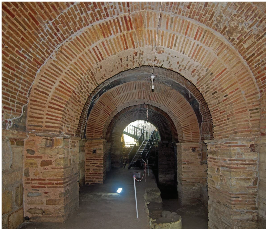
Figure 3.13. Substructure from 1 st phase with brick vault and arches
