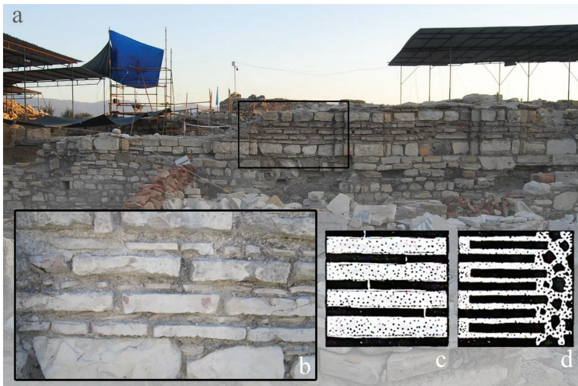
Figure 2.2. Recessed brick technique, a: Northern façade of Anaia Church (Photo: E. Çam, 2020), b: Detail of squared area shows recessed bricks (Source: Kanmaz 2015), c: Elevation sketch of the technique (Source: Ousterhout 1999, 174), d: Section sketch of the technique (Source: Ousterhout 1999, 174)
