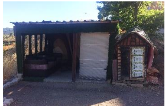
Figure 48. Sitting Areas created in Open Area of Uzundere TOKI Housings – II (Source: Diclehan Bekir 2019)
