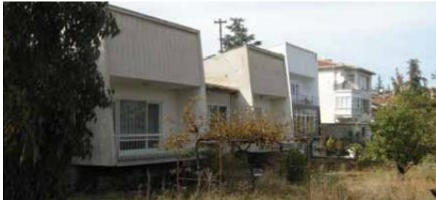
Figure 20. Merbank Housing (Merbank Mensupları Building Cooperative Housing) (Source: Sivil Mimarlık Tarihi Ankara 1930-1980 2014, 125)
