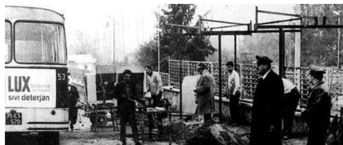
Figure 4.34. Sirinyer, Front Of The Prison During In 1970's.
