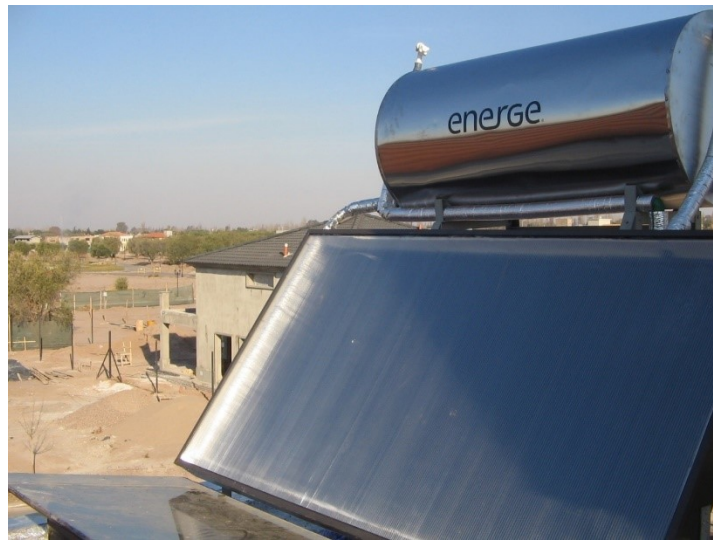
Figure 7: Thermosiphon uses sunlight to heat water (Source: URL4)
