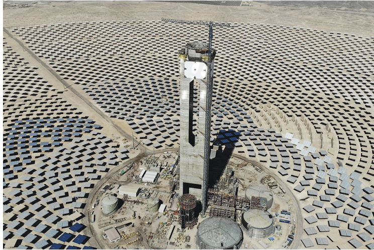
Figure 6: Concentrated solar power plant (Source: URL3)
