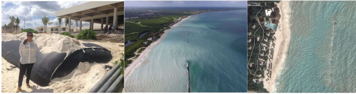
Figures 13. On shore breakwater Figure 14. Installation 2016 Figure 15. Situation 2017
