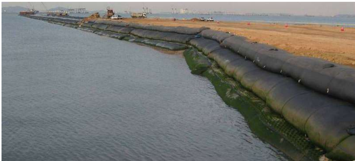
Figure 5. Installed Geotube system as perimeter bund
