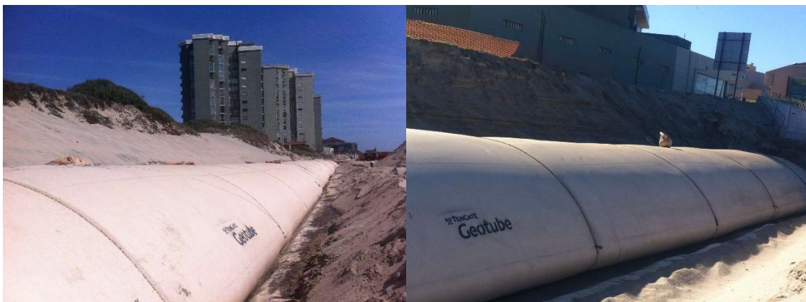
Figure 26 & 27. Installed geotextile tubes before covering with sand
