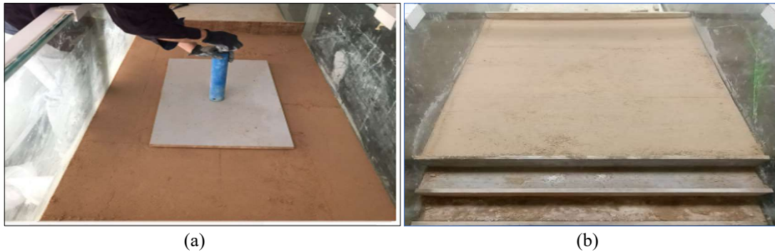
Figure 4. Some construction stages: a) Compacting by proctor hammer, b) After compaction of the first layer
