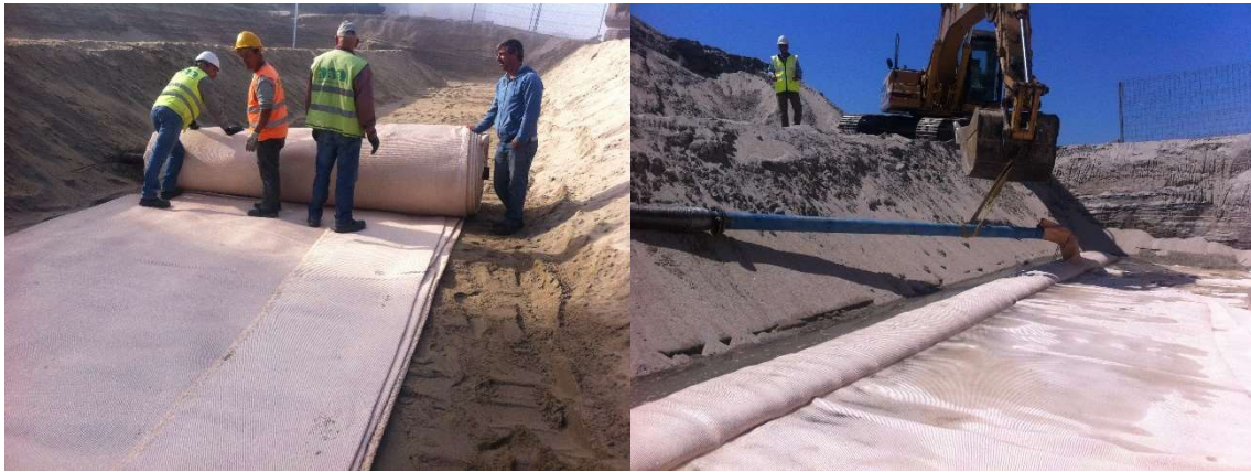
Figure 22 & 23. Installation scour apron and filling anchor tube
