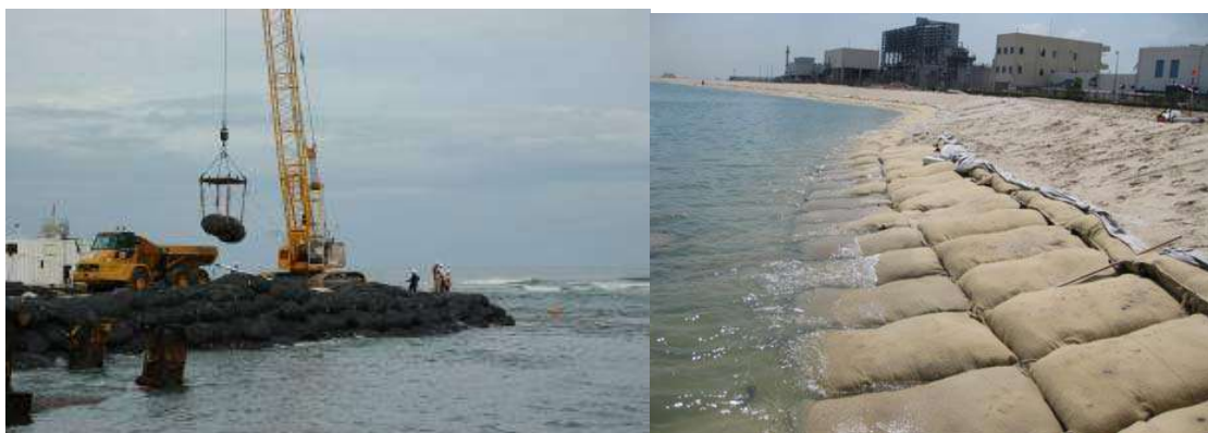
Figure 1 & 2. Installation of Geobags
