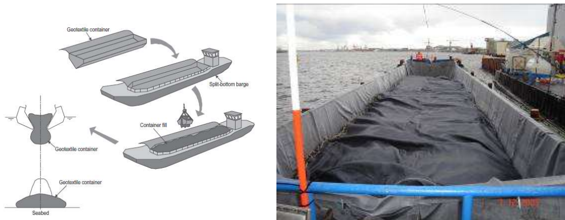
Figure 3 & 4. Deployment and installation of Geocontainer systems.
