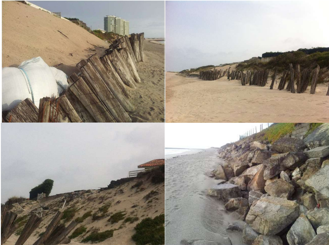
Figures 16-19. Situation before installation of geotextile tubes
