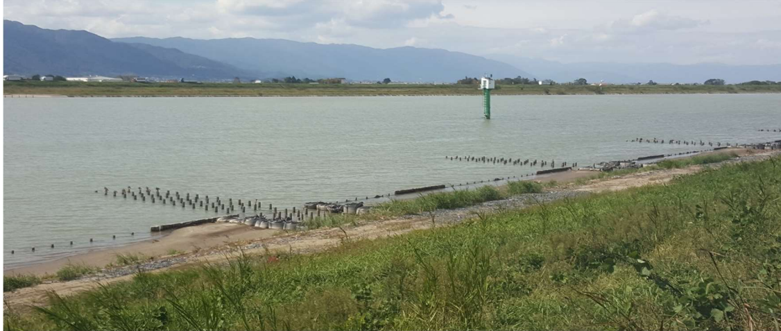
Figure 1. A series of pile-group groynes along the Kiso River, Japan
