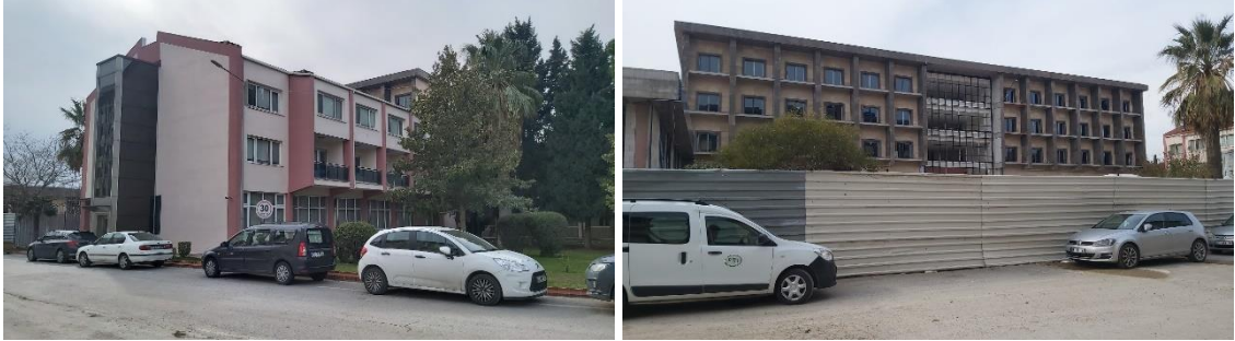
Figure 3.19. The guesthouse structure in the DSİ Campus (Source: The photo taken by the author.)
