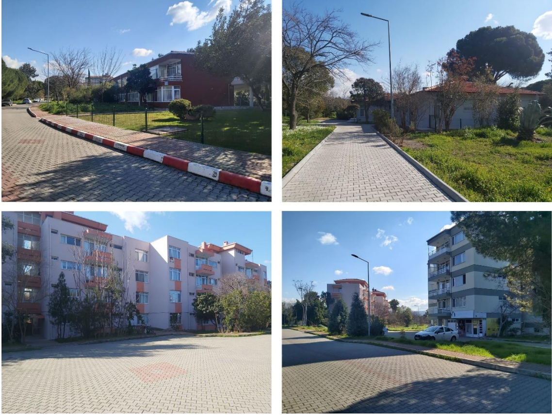
Figure 4.13. The collage shows the structure typologies in Ege University lodging area (Source: The photos taken by the author.)
