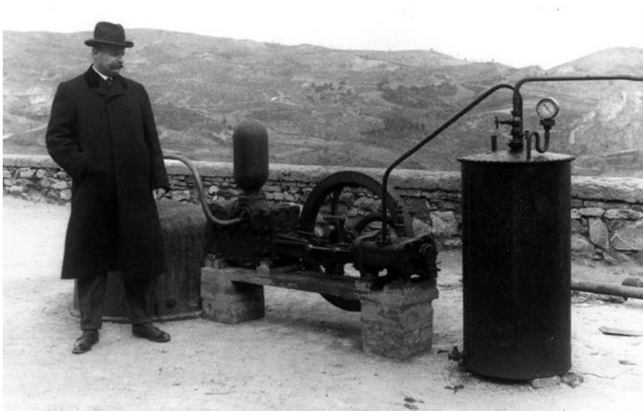
Figure 3.1. First machine to generate geothermal to electricity
