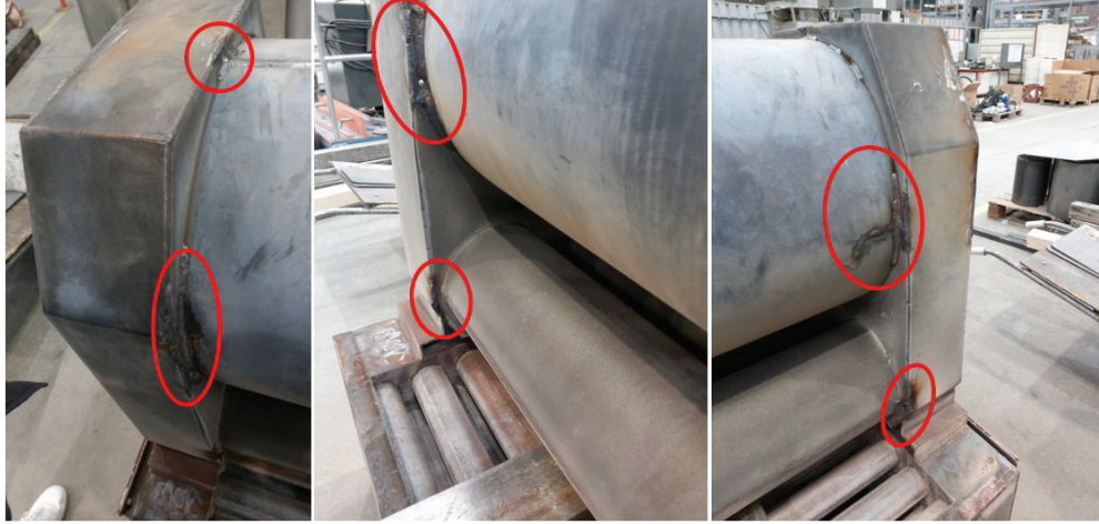
Figure 1.6. Some crack examples on the heat exchanger / ELECTRON Company Internal Report
