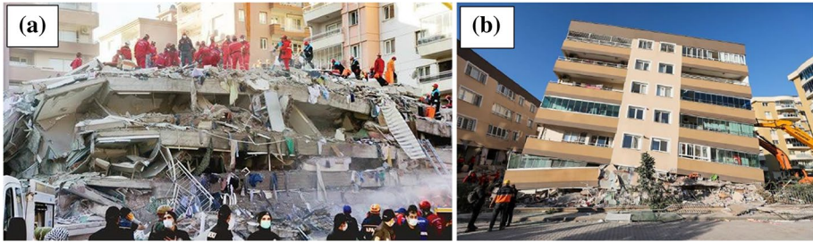
Fig. 15 a Pancake collapse, b Ground floor failure ( https://www.aa.com.tr/tr/pg/foto-galeri/izmir-depremi/0 )
