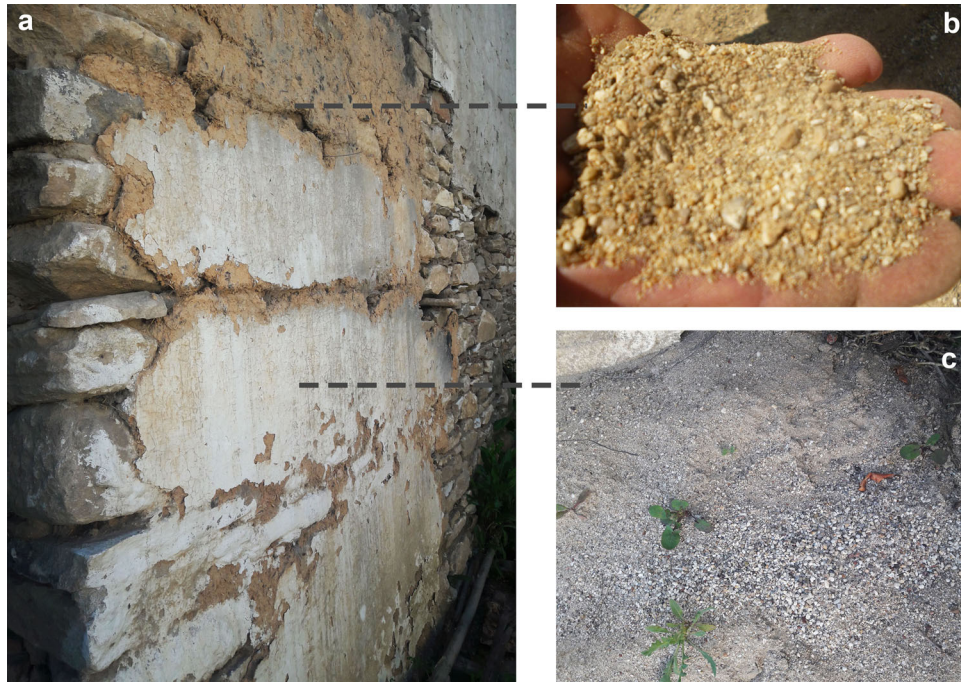
Figure 24. (a) Double-layer plaster on the wall, (b) yellow soil for the mud plaster, (c) fine sand for the lime plaster.
