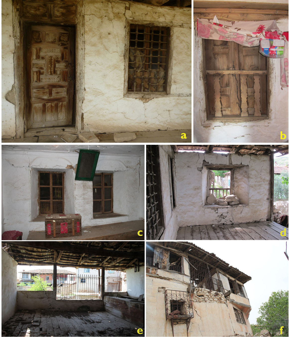
Figure 20. (a) Single-leaf wooden door and lokma parmaklık in the window opening, (b) wooden shutter and balustrade in the window of a room, (c) double-glazed casement windows in a room of RG's house, (d) wooden shutter and balustrade in a sofa window, (e) iron railing in iwan of HÇ's house, (f) iron railing in iwan and window in Gölde Evi.
