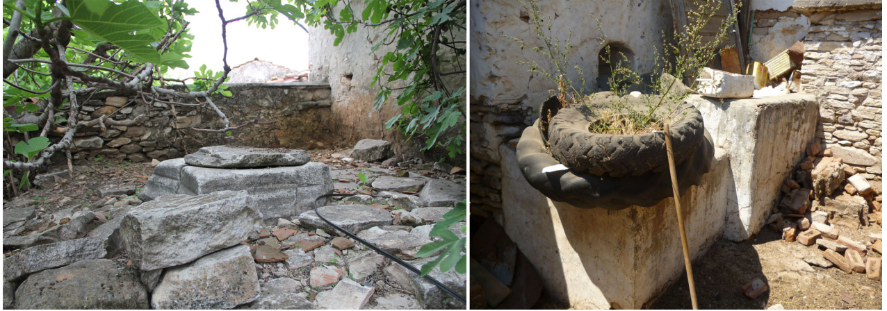
Figure 10. A well to store rainwater in the courtyard of a house (left) and an apilimi attached to the courtyard wall of another house (right).
