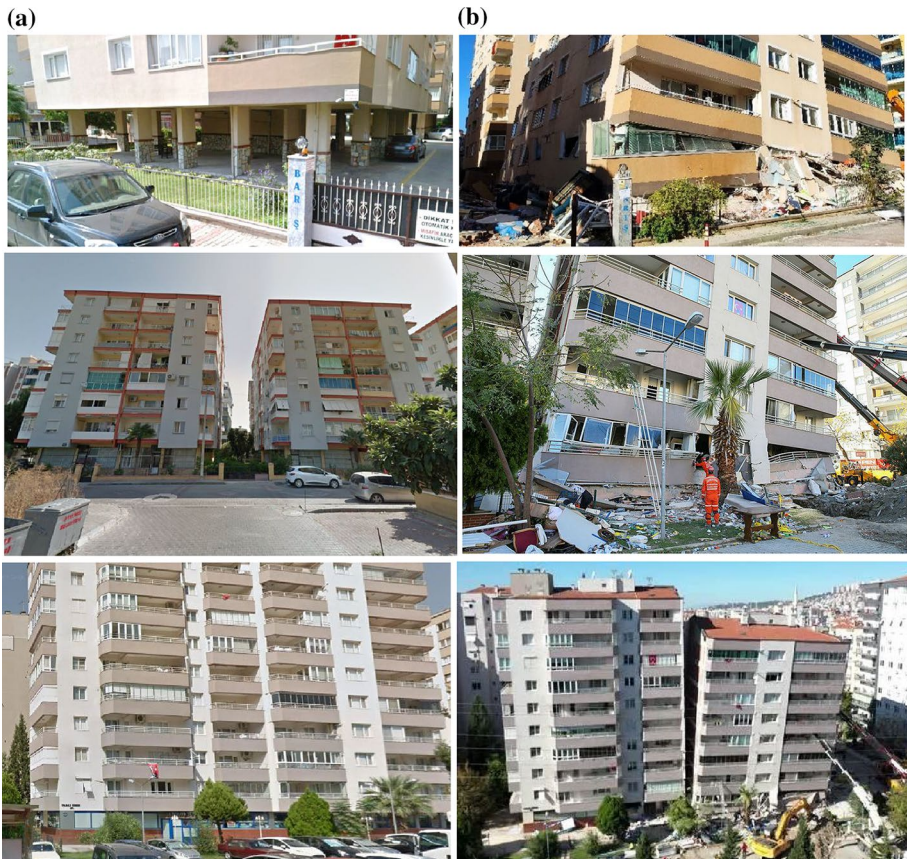
Fig. 7 Failure due to soft/weak story. a Before the earthquake (left), b after the earthquake (right)
