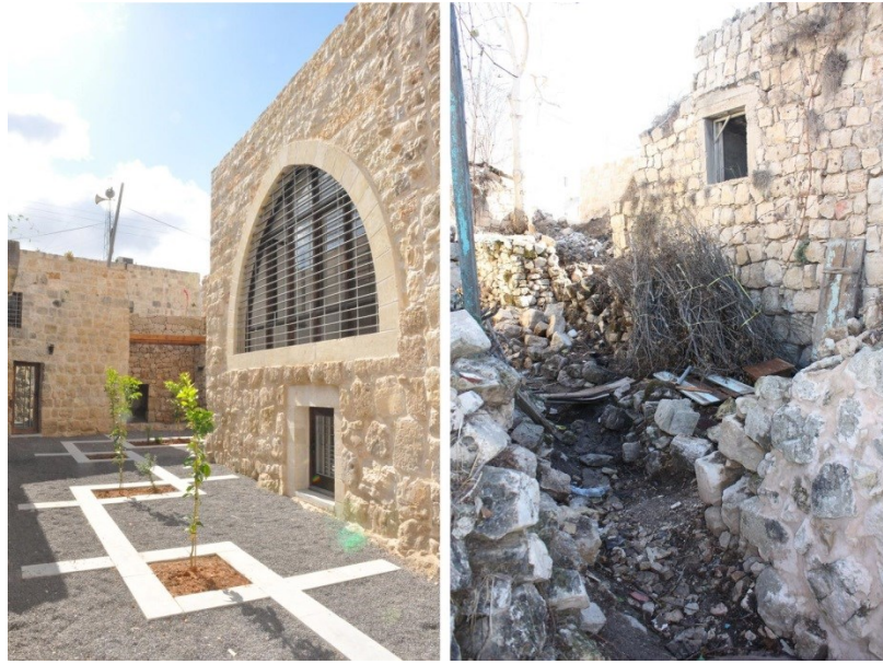
Figure 53. Birzeit Municipality guest house. Before (right) and after (left) restoration. (Source: Archnet)
