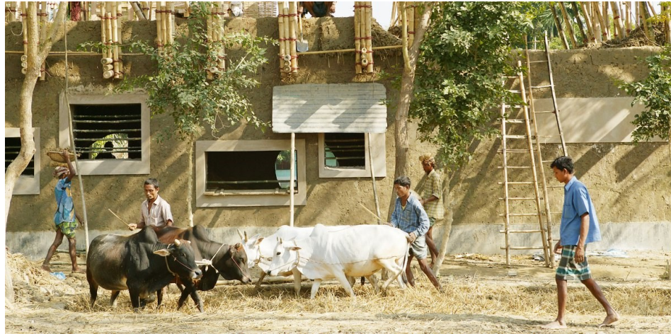
Figure 22. An image from the construction stage. 125
