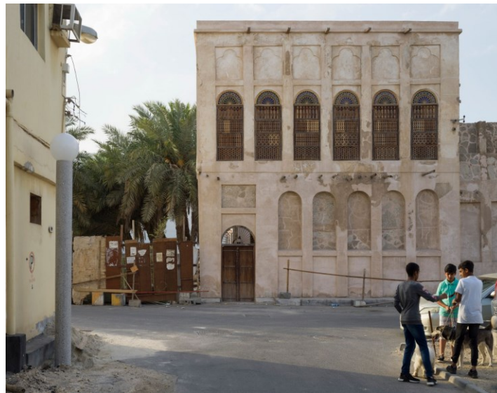
Figure 58. Renovated facade of Fakhro House. (Source: Archnet)
