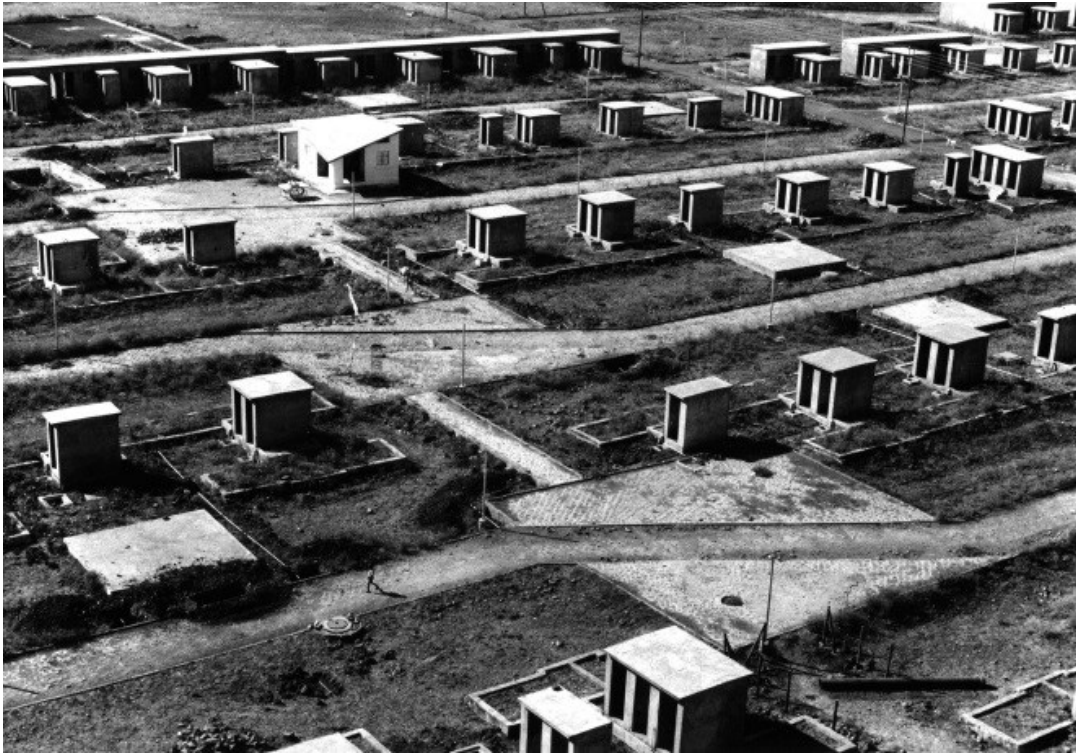
Figure 46. Each plot is provided with a plinth, a toilet at the back and an electrical connection: architecture as system and process rather than finished structure (Source: Vastushilpa Foundation)
