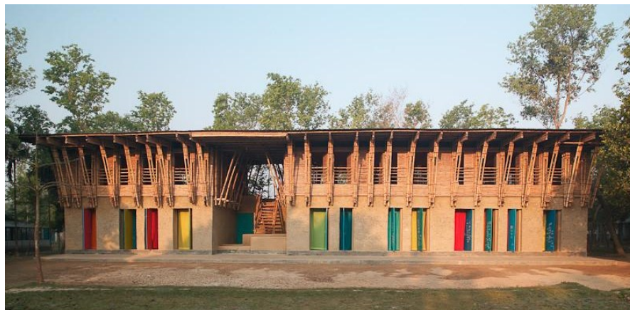
Figure 19. Meti School Elevation. (Source: Arhnet)
