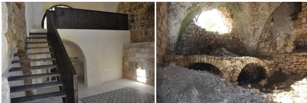
Figure 54. Birzeit University Guest House Before (right) and after (left) restoration. (Source: Archnet)
