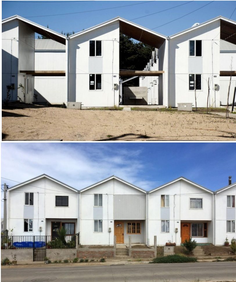
Figure 16. Villa Verde Houses project in Chile's coastal town Constitución, half houses in 2010 (above) and full houses in 2013 (below). (Source: https://www.archdaily.com/450958/elemental-s-half-finished-housing-typology-a-success-in-all-circumstances )
