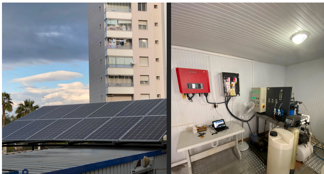
Fig. 6. Solar panels (left), RO system powered by PV module (right).
