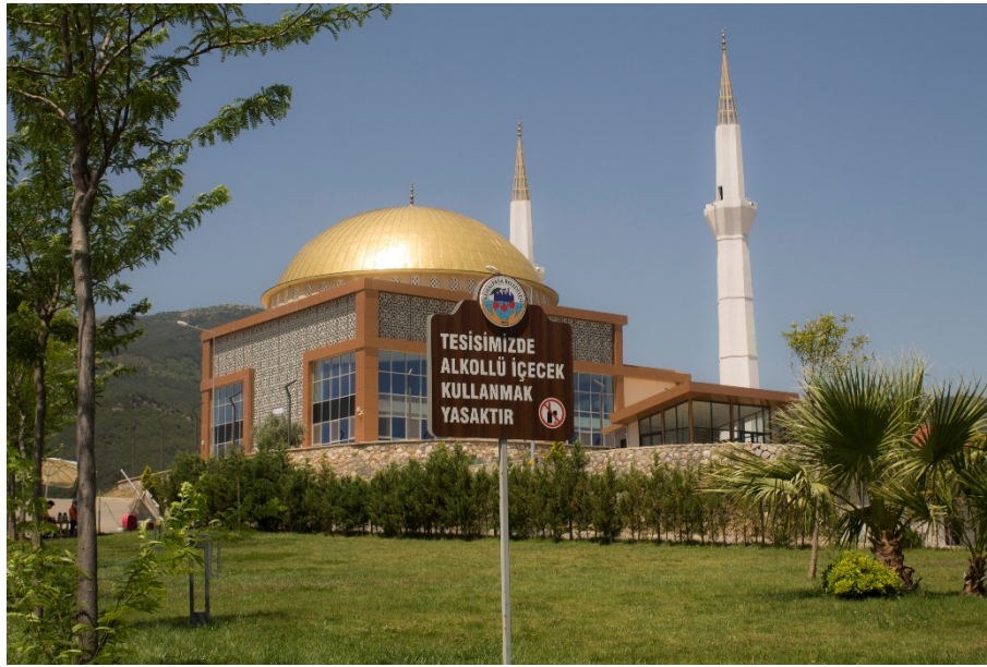
Figure 31. Visual of Warning Sign (Field Survey, June 2021)
