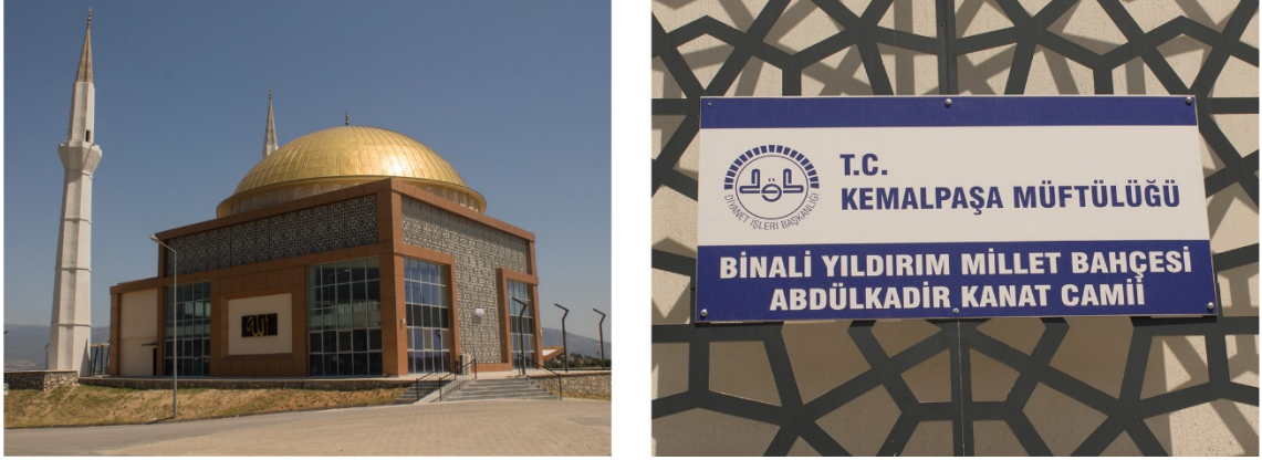
Figure 29. Kemalpaşa Nation Garden Mosque and Its Escutcheon (Field Survey, June 2021)
