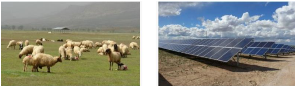
Figure 2. 17. SPP Project in Elmalı-Antalya
