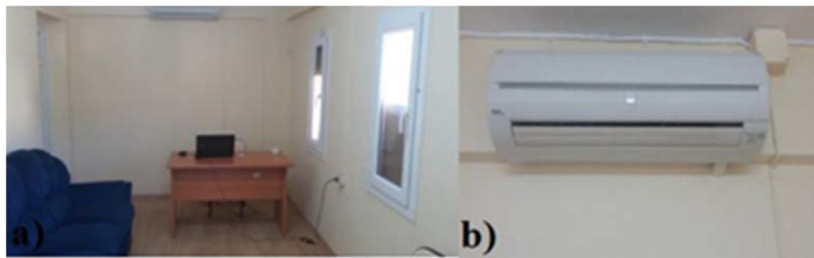
Fig. 4. a) Inner view of the case building, b) Split type air-conditioner used in the case building.
