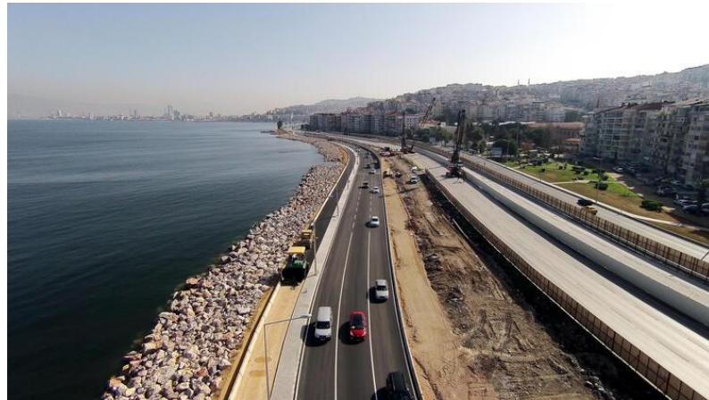
Figure 30. Construction of underpass in Mustafa Kemal Coastal Boulevard (Source: YA, 25.12.2015)
