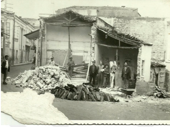
Figure 101. Around Big Bridge (Source: Kemal Ergun's Archive)
