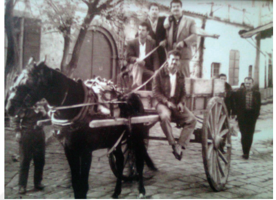
Figure 102. Around Big Bridge (Source: Kemal Ergun's Archive)
