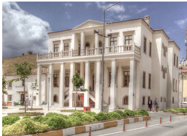
Figure 92. Town Hall after restoration (Source: Urla Municipality)
