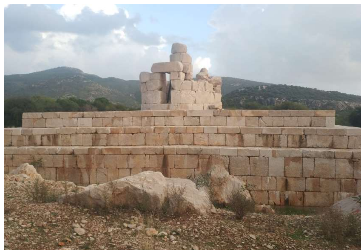
Figure 5.1: The current situation of the lighthouse
