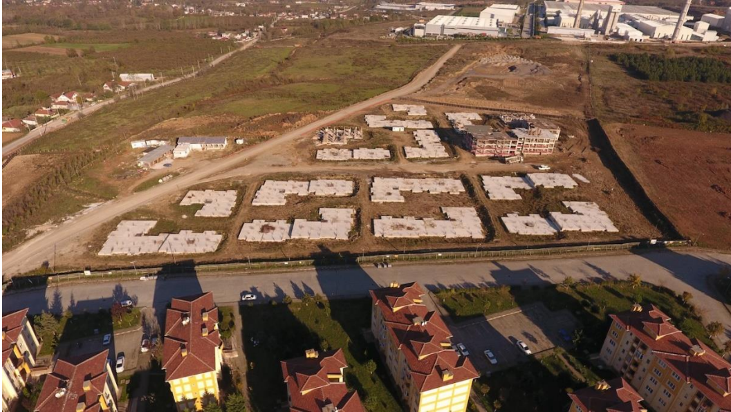
Figure 4.15. Düzce Hope Homes project, view from drone in 2017. (Source: Düzce Hope Homes Archive 2019)
