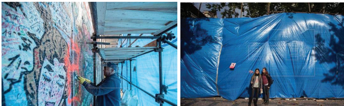
Figure 105. Reconstruction Works of Lennon Wall (Source: efe.com photographed by Divisek, 2019)
