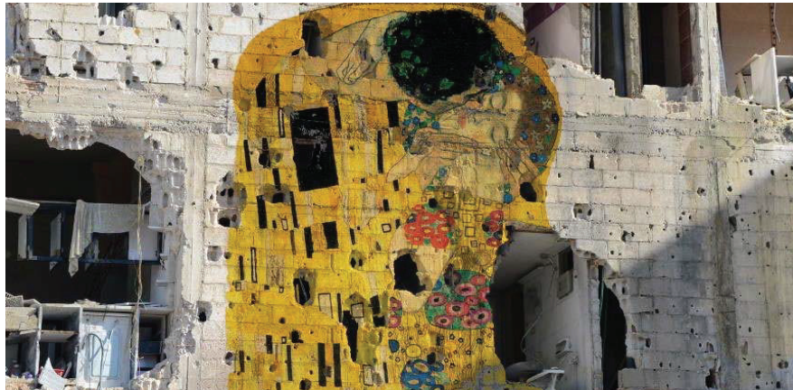
Figure 50. Artist Tammam Azzam's Artwork, Crumbling and Bullet-torn Surface of a Building in Damask, Awareness of the Gravity of Civil War. (Source: https://www.widewalls.ch/urban-art-the-tale-of-inspiration/ )
