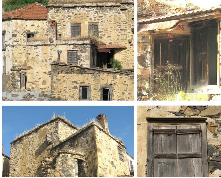
Figure 4. 52. View of stone facade and wood joinery. 184
