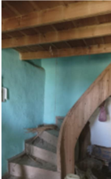
Figure 4. 43. View of inner timber stairs.
