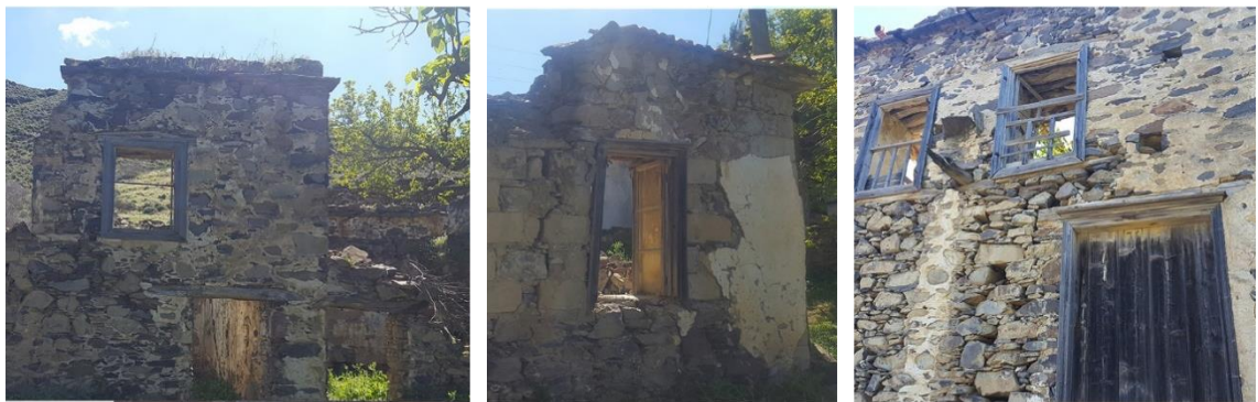
Figure 4. 40. Views of windows and doors in exterior.
