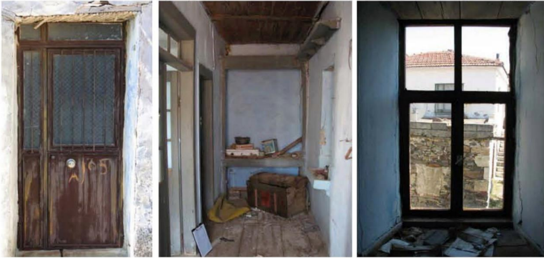
Figure 4.46.1 Entrance door. Figure 4.46.2 View of floor. Figure4.46.3 Southeast window. 178
