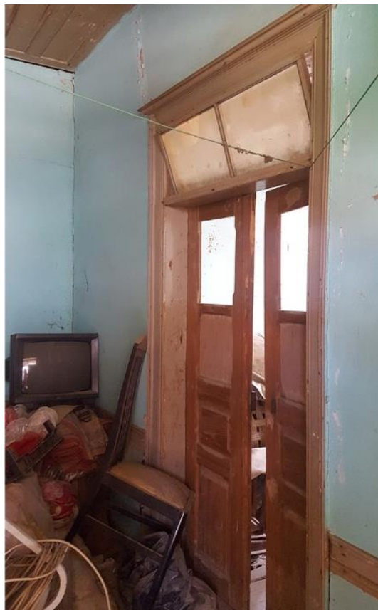
Figure 4. 31. View of interior side.
