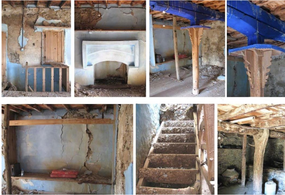
Figure 4. 53. Floor systems carrier beam, stove, and furnace. 185
