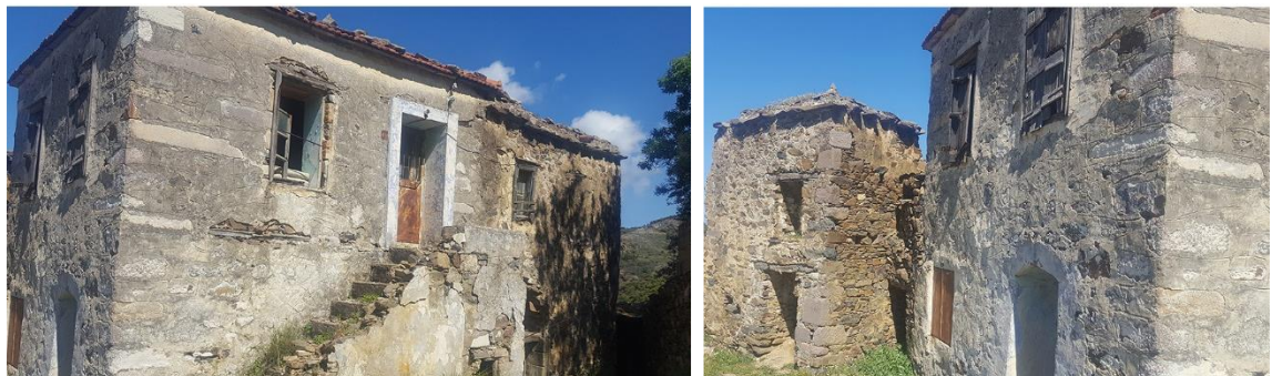
Figure 4. 41. Views of two-story village houses.
