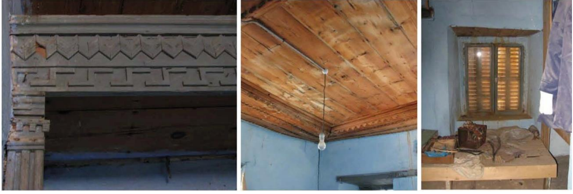
Figure 4.47.1 Frame of alcove. Figure 4.47.2 Ceiling covering. Figure 4.47.3 Ground floor window. 179
