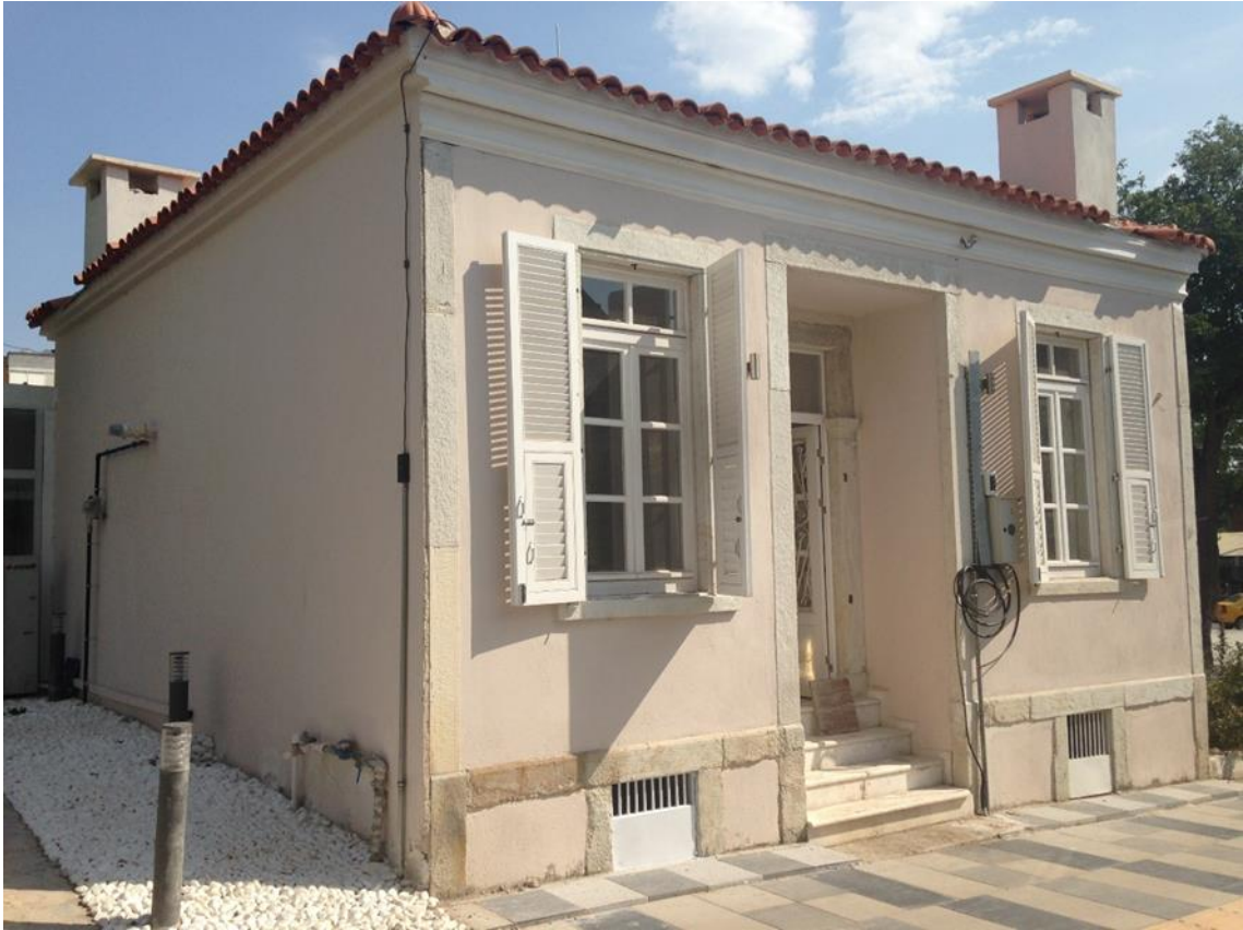
Figure 3.16. The north-west facade of the house in Buca
