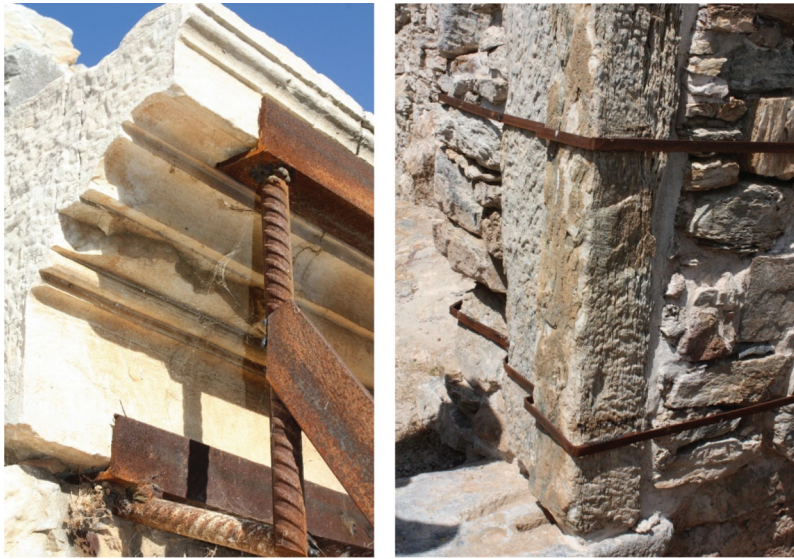
Figure 4. Rusting problem in a Roman (left) and Byzantine (right) ruin, Antiochia ad Cragum, Antalya, Turkey.
