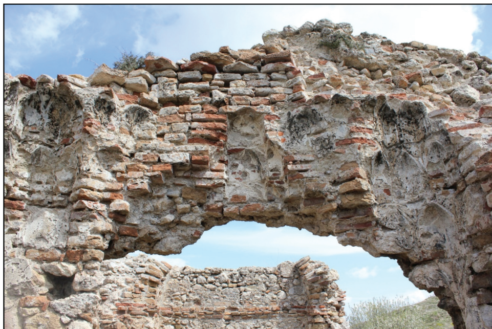
Figure 10. Dome remain as viewed from south.
