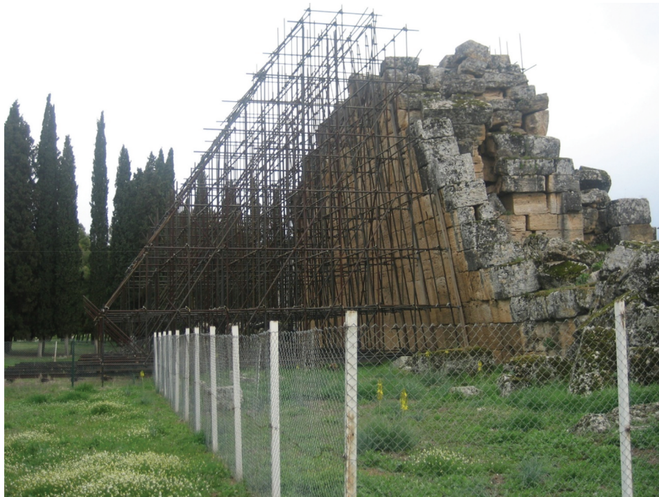
Figure 5. Supporting of the wall, the Basilica Bath in Hierapolis, Denizli, Turkey.
