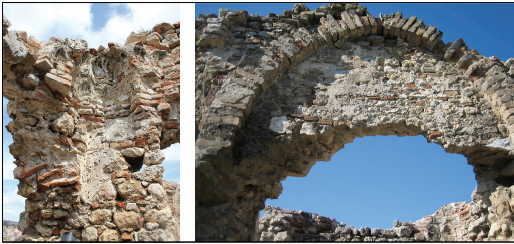
Figure 11. Squinch remain as viewed from southeast (left), arch remain as viewed from north (right).
