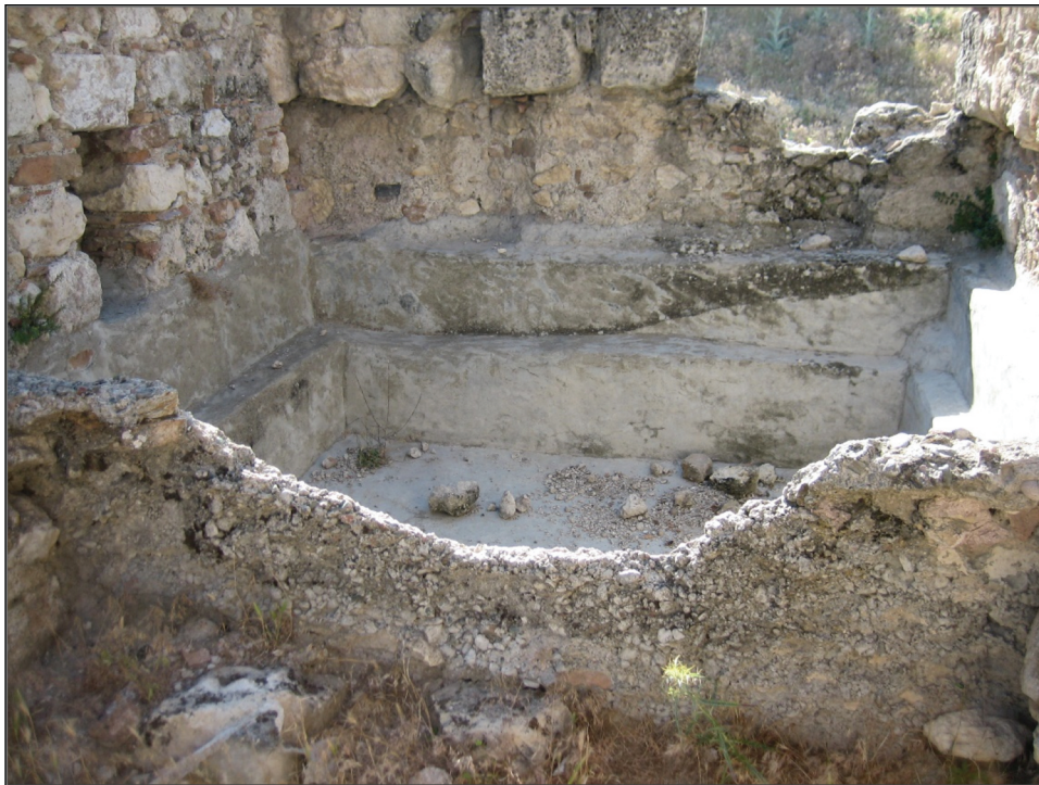
Figure 12. Load-bearing walls: rough-cut stone at both surfaces, rubble stone and lime mortar in between (left), rough-cut stone with cement mortar.
