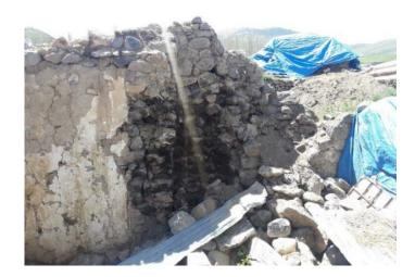
Figure 3.100. The ruins of the fireplace on the south wall of the machine house. (Photograph: Author, 2019).
