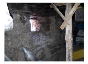
Figure 4.13. Wooden posts supporting the warehouse roof. (Photograph: Author, 2019)
