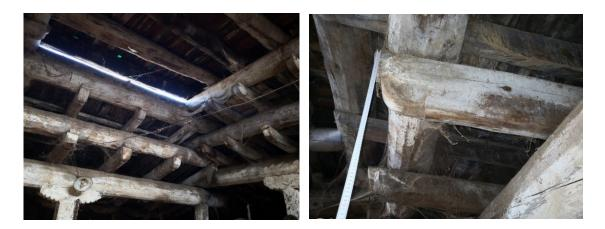
Figure 3.93. Corbelled ceiling and skylight and wooden joist sharpened in the form of hammerhead its ends (Photograph: Author, 2019).
