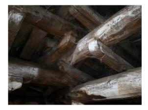
Figure 3.95. The corner mergence of hammerhead joists. (Photograph: Author, 2019)
