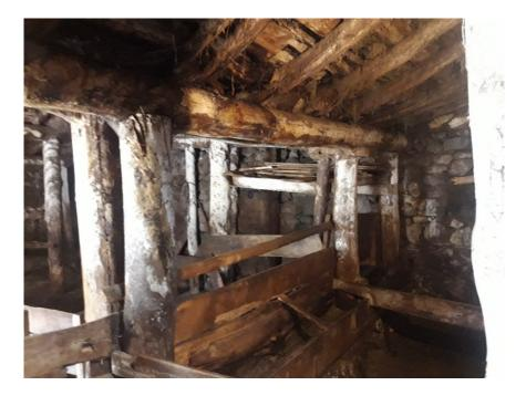
Figure 3.79. Serial of wooden posts separating the northern and southern parts. (Photograph: Author, 2019)
