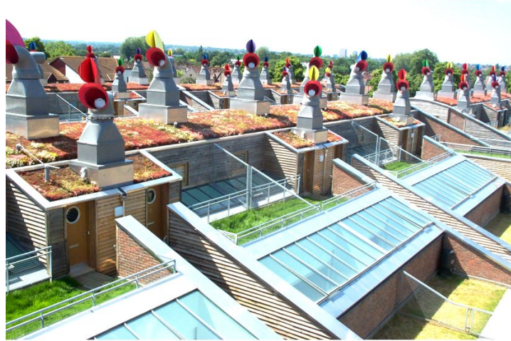
Figure 3.17. Rainwater harvesting terraces (Source: Lazarus, 2003: 25)
