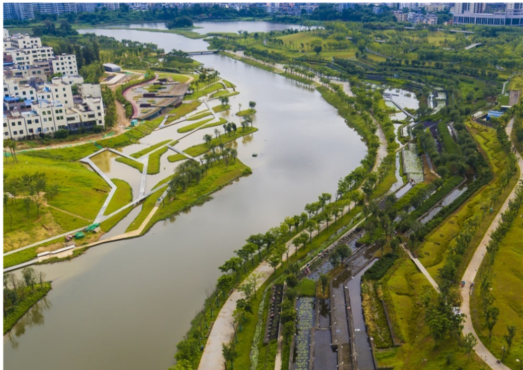
Figure 3.10. Part of the region after the project is completed (Source: Turenscape, 2019)
