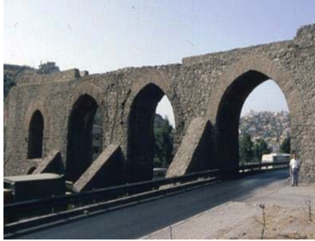
Figure 4.2. Vezir Waterway (Source: IZSU, 2017:6)
