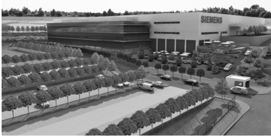
Figure 3.23. Siemens Gebze Facility (Source: Yaman, 2009: 1094)
