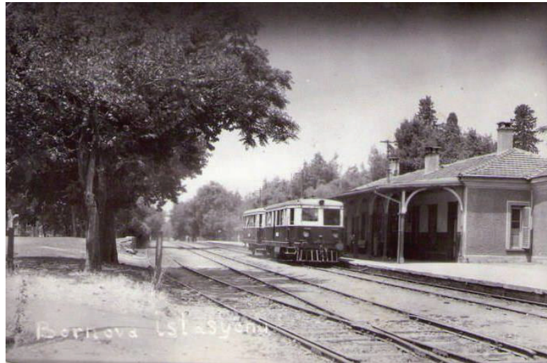
Figure 4.24. Train Station in Bornova in beginning of 1900's (Source:www.levantineheritage.com)
