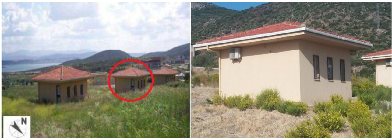
Fig. 3. The case building and the surroundings.
