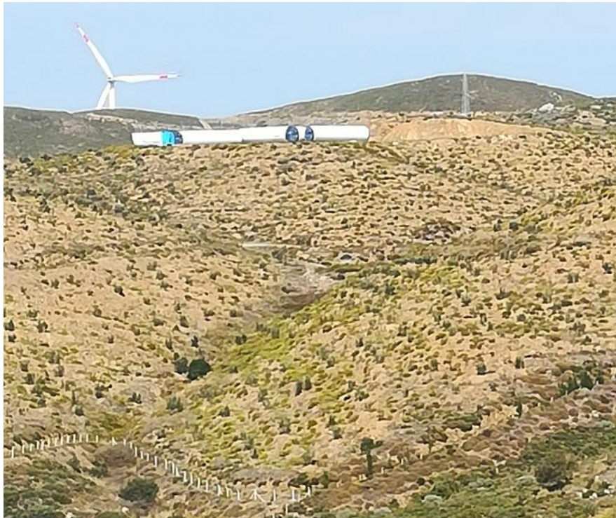
Figure 6. 9. Wind Turbines under Construction in Olive Groves (Field Survey, October 2018)
