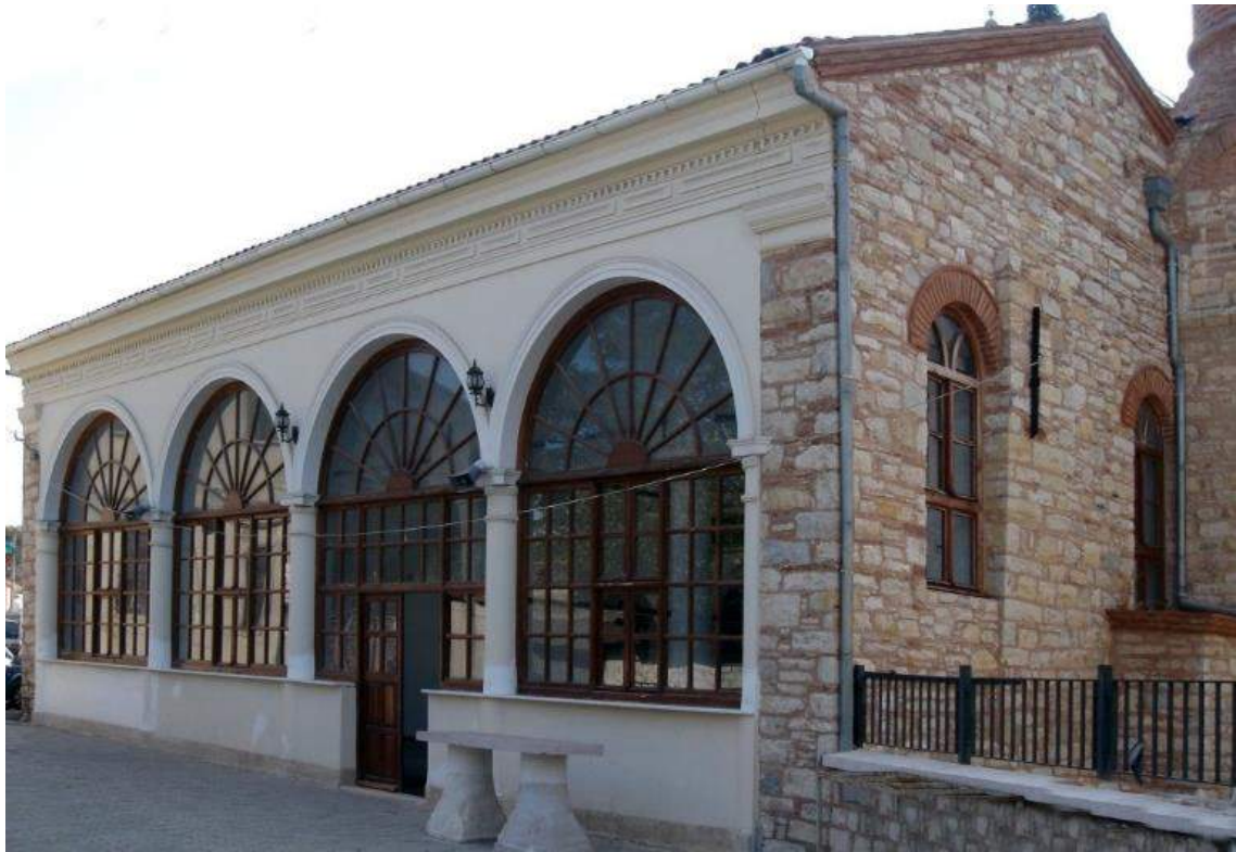
Figure 3.39. Last comers' hall as viewed from north (Source: RDPF Archive, 2006)
