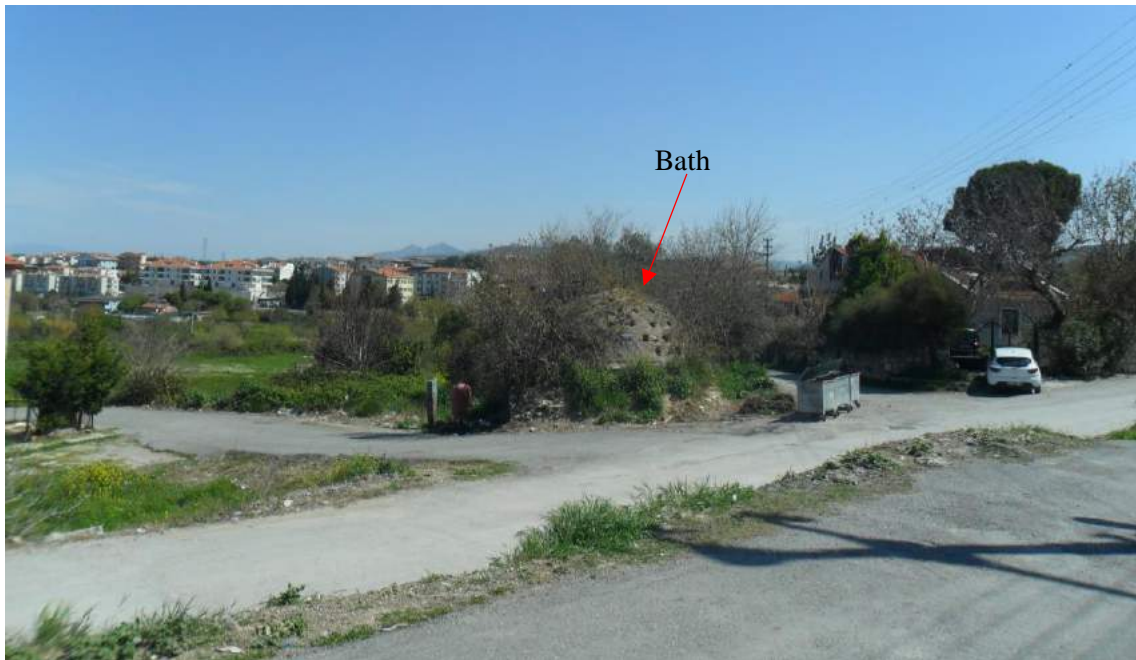
Figure 3.92. Rüstem Paşa Bath current situation as viewed from the northwest
