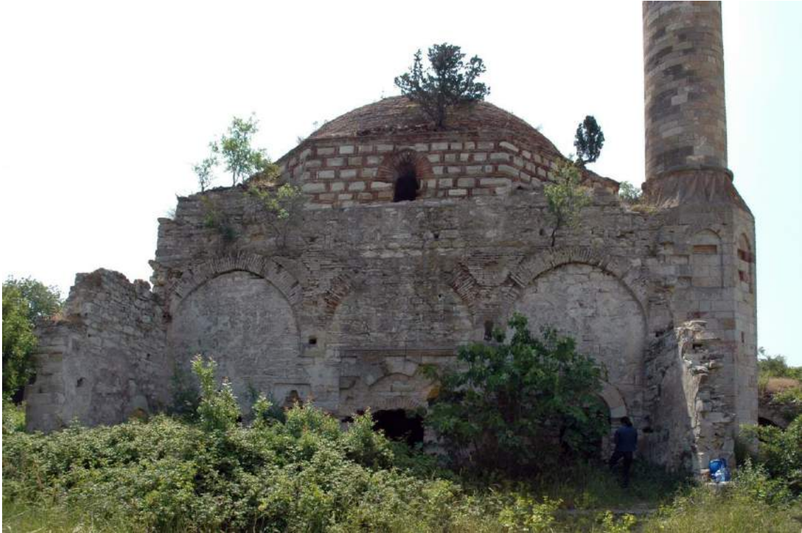
Figure 3.21. Last comers' hall before restoration process as viewed from the northwest (Source: RDPF Archive, 2006)
