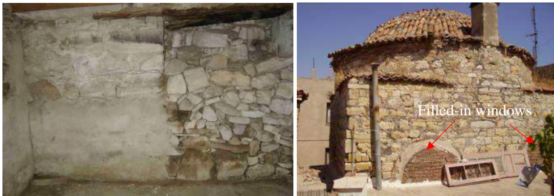
Figure 3.75. Kapan children's school before restoration implementation, interior of southwest wall (left), exterior of southeast wall (Source: Balcioglu, n.d.)
