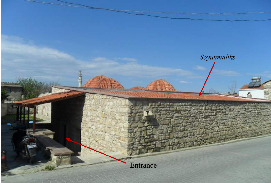
Figure 3.83. After restoration implementation as viewed from the east corner
