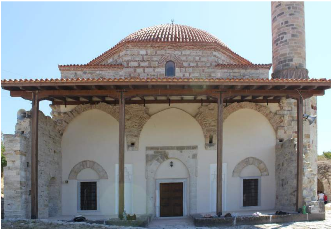
Figure 3.22. Last comers' hall after restoration process as viewed from the northwest
