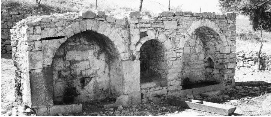
Figure 3.35. Kamanlı Bath Fountain as viewed from southeast (Source: RDPF Archive, 1980)
