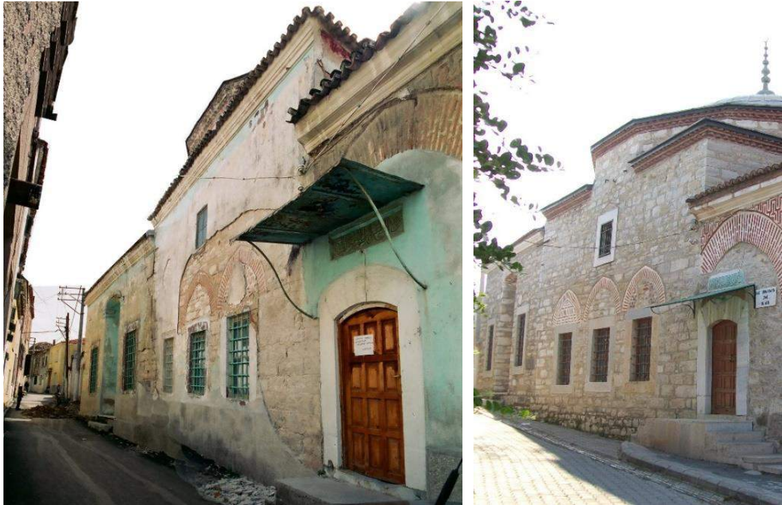
Figure 3.63. The Kapan Mosque before (left) and after restoration implementation as viewed from the west (Source: RDPF Archive, 1990)
