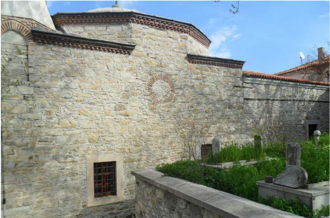
Figure 3.67. The Kapan graveyard after restoration process as viewed from the south
