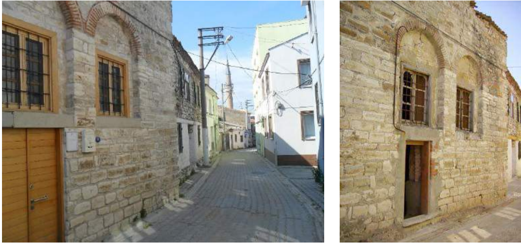
Figure 3.74. The Kapan school after (left) and before (right) restoration implementation as viewed from the northeast (Source: Conservation Board Archive, 2008)
