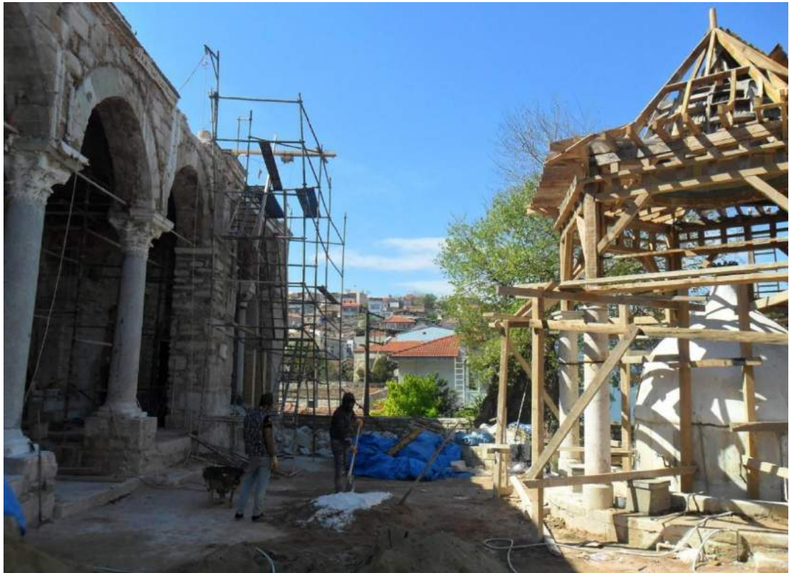
Figure 3.14. The courtyard as viewed from the northeast
