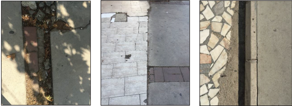
Figure 5.37. Damaged sidewalk materials in the case study area
