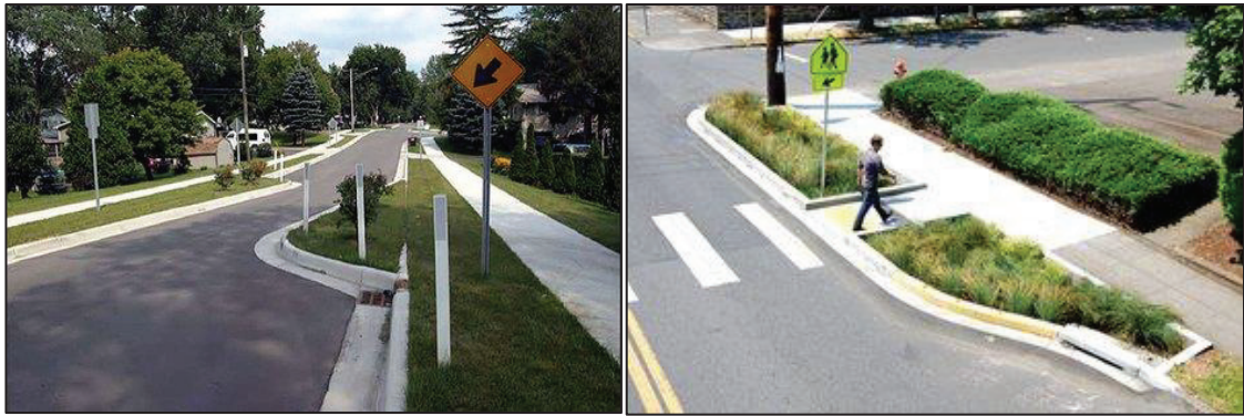
Figure 3.2. Traffic calming toolbox - examples of possible traffic calming treatments from right to left: choker and bulb-out/curb extension (Source: C. Gables, n.d.)
