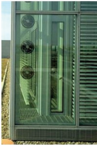
Figure 2.14. Headquarters of Götz Building shading device and cavity view (Source:Örkmez,2012)
