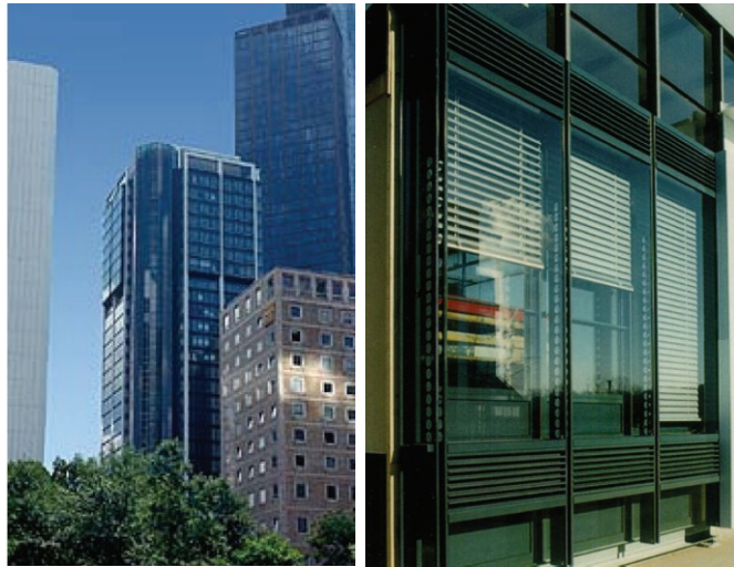
Figure 2.20. Eurotheum Tower building exterior view and blinds (Source:Ünal,2006).
