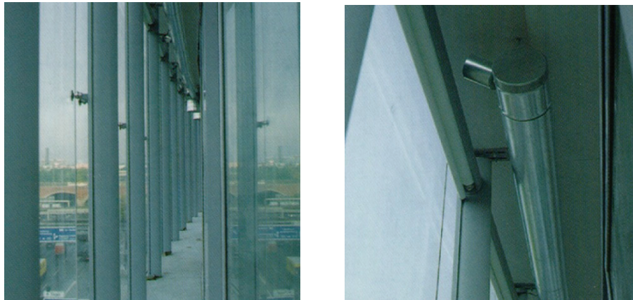
Figure 2.12. Halenseestrasse Building shading device and cavity view (Source:Örkmez, 2012).
