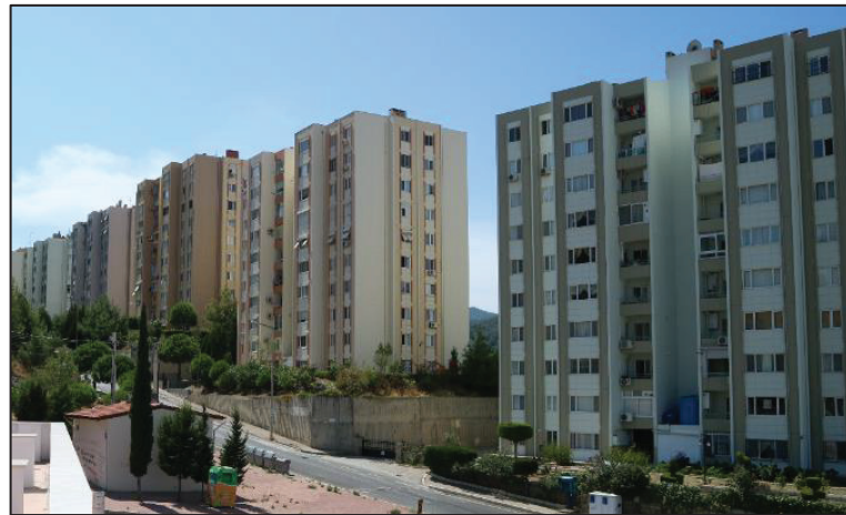
Figure 5.21. Narbel mass housing site (Source: Taken by the author during the field study, 2018)
