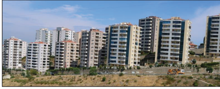
Figure 5.17. Multi-storey housing in İkinci İnönü Neighborhood (Source: Taken by the author during the field study, 2018)
