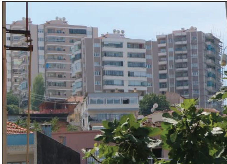
Figure 5.16. Detached multi-storey apartments in İkinci İnönü Neighborhood (Source: Taken by the author during the field study, 2018)
