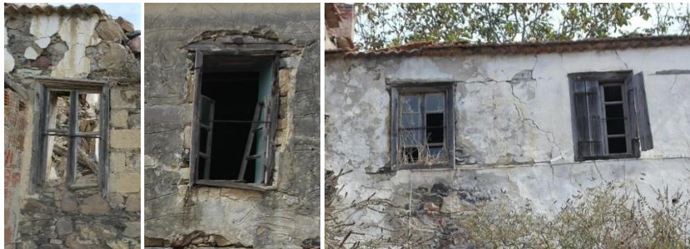
Figure 4.70. Double Casement Window Examples in Küçükbahçe (October 2016).
