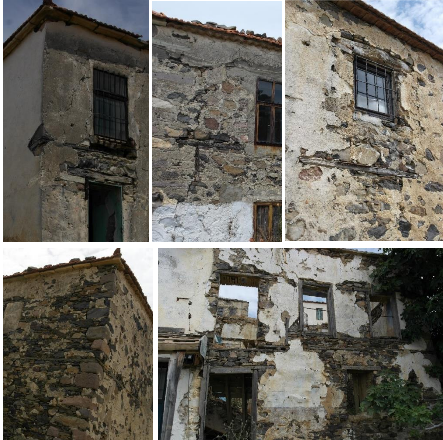
Figure 4.10. Lintel Usage in Küçükbahçe (May 2017).
