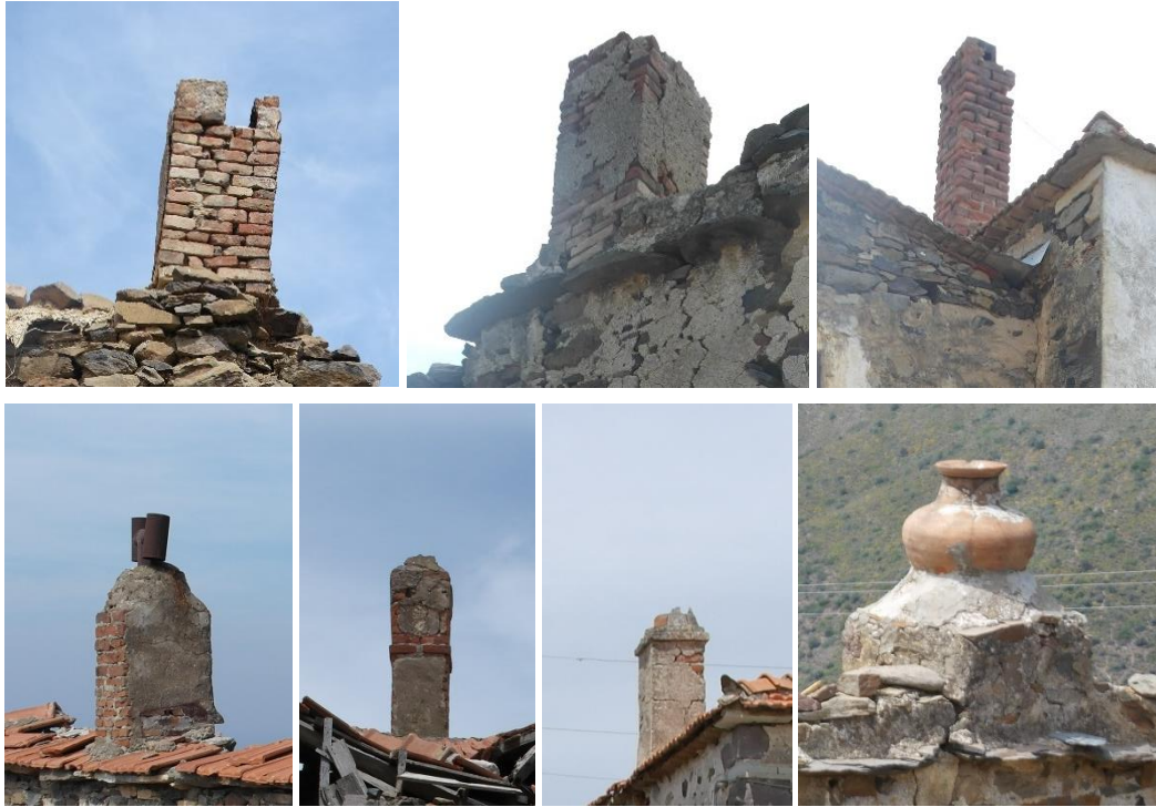
Figure 4.95. Chimney Examples in Küçükbahçe (April 2017).
