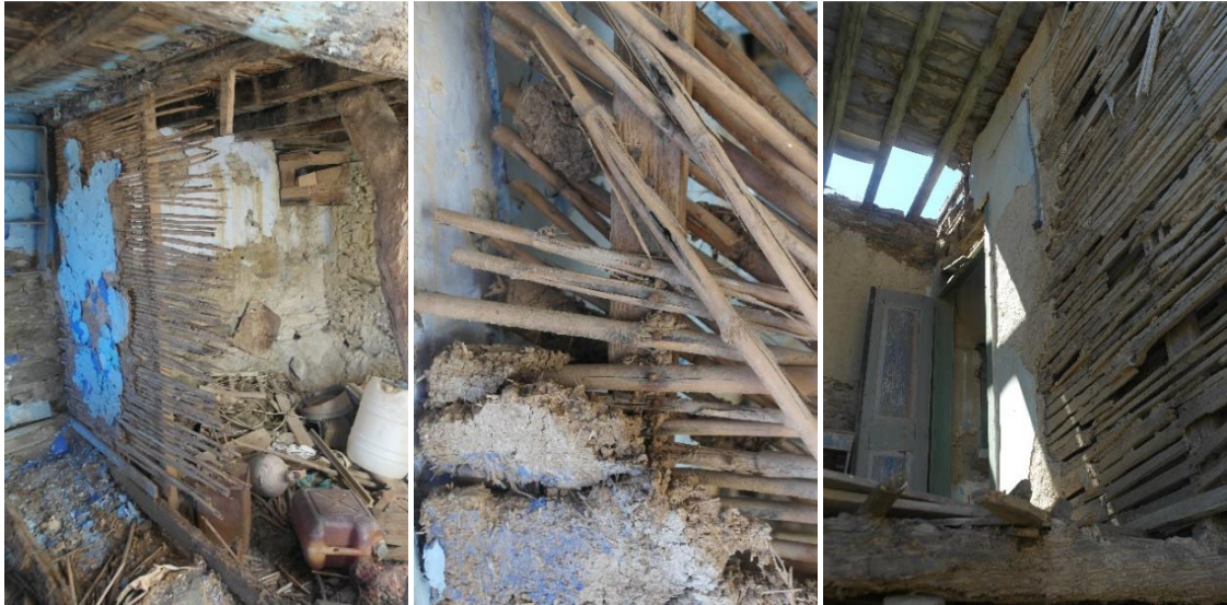
Figure 4.30. Timber Framed Wall Examples in Salman (May 2017).
