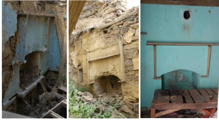
Figure 4.90. Fireplace Examples in Küçükbahçe (April 2017).
