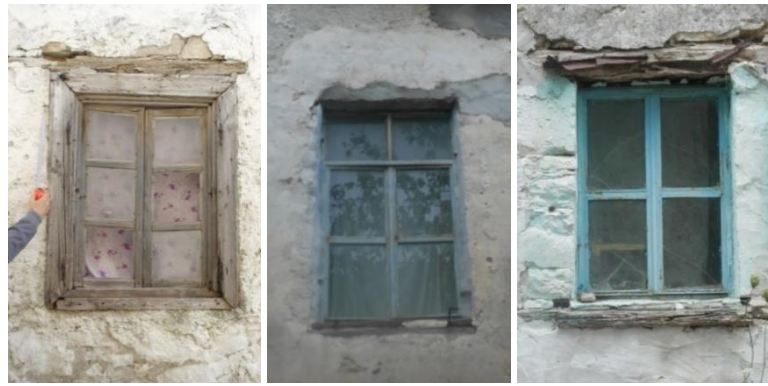
Figure 4.69. Double Casement Window Examples in Kösedere (June 2016).
