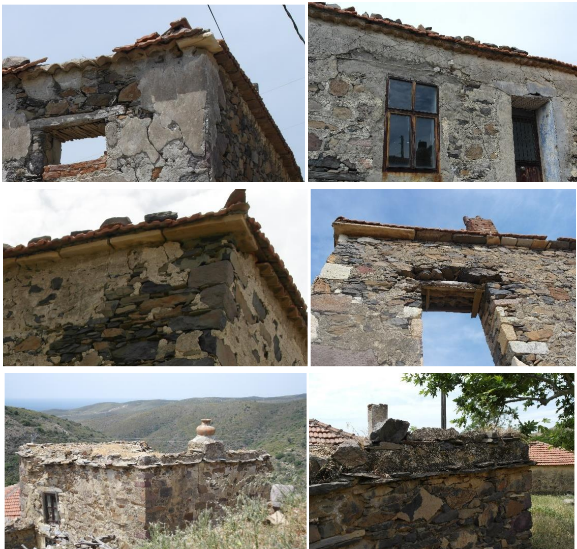
Figure 4.58. Tile and Stone Eave examples in Küçükbahçe (April 2017).
