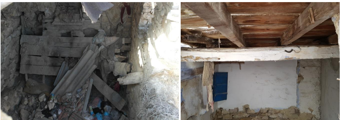
Figure 4.40. Floor Construction example (a) Eğlenhoca (b) İncecik (June 2017)
