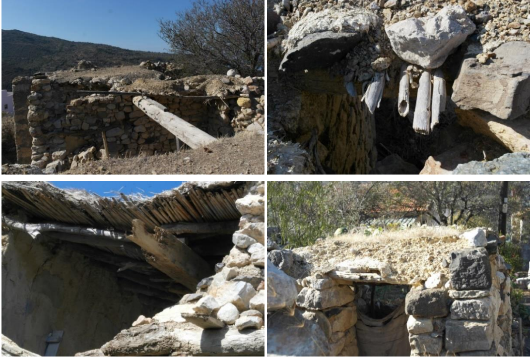
Figure 4.53. Fat roof examples in Bozköy (June 2016).
