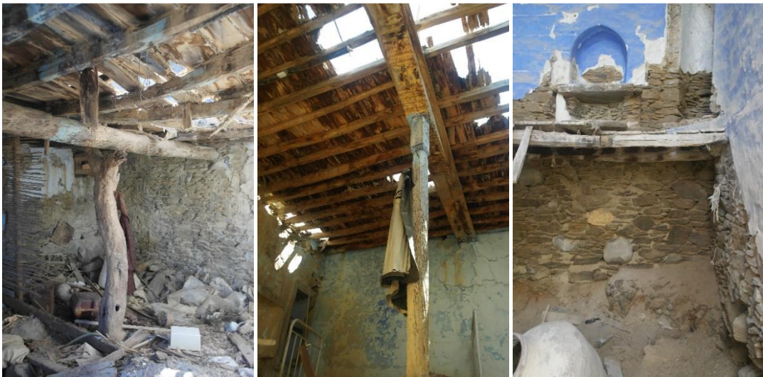
Figure 4.42. Floor Construction in Salman (May 2017).
