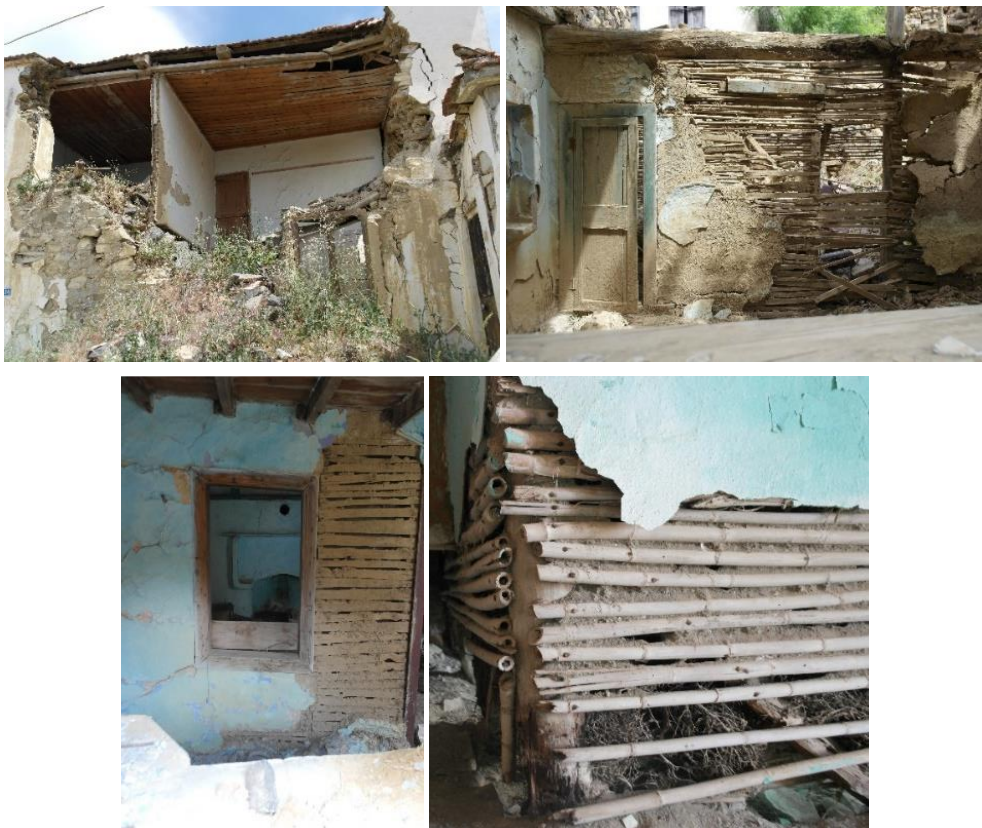
Figure 4.29. Timber Framed Wall Examples in Küçükbahçe (April 2017).
