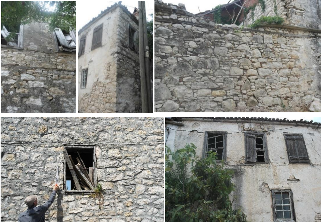
Figure 4.8. Lintel Usage in Kösedere (June 16).
