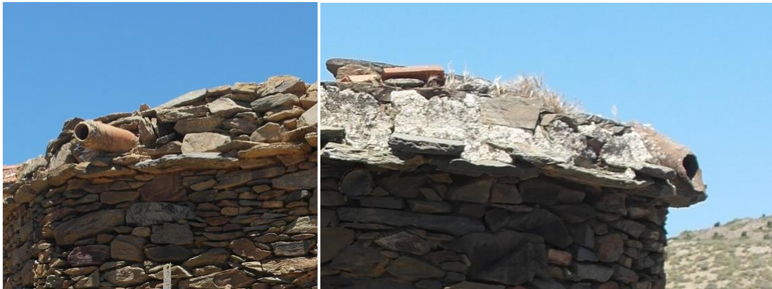
Figure 4.112. Waterspout Examples in Parlak (May 2017).
