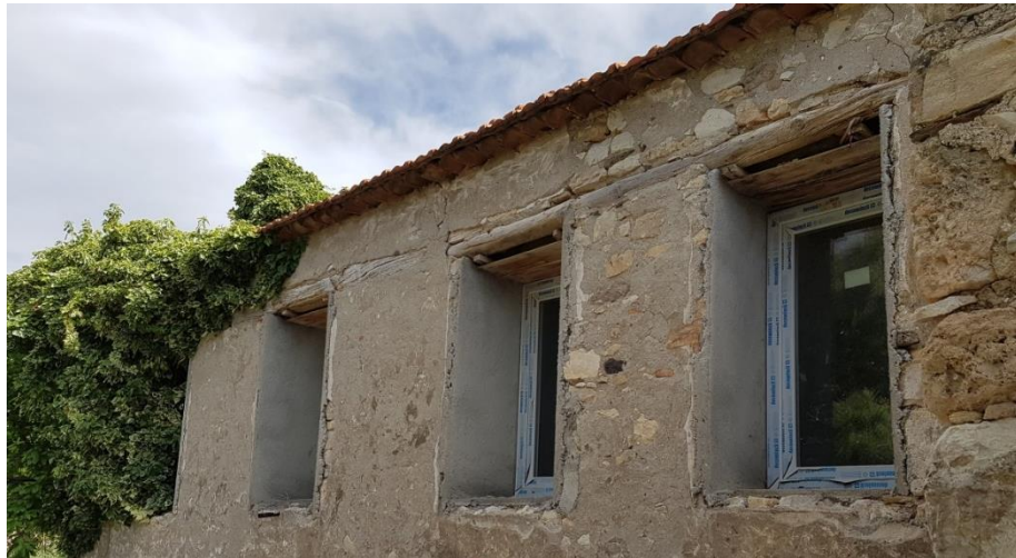
Figure 4.21. Spanning Openings in Tepeboz (April 2017).
