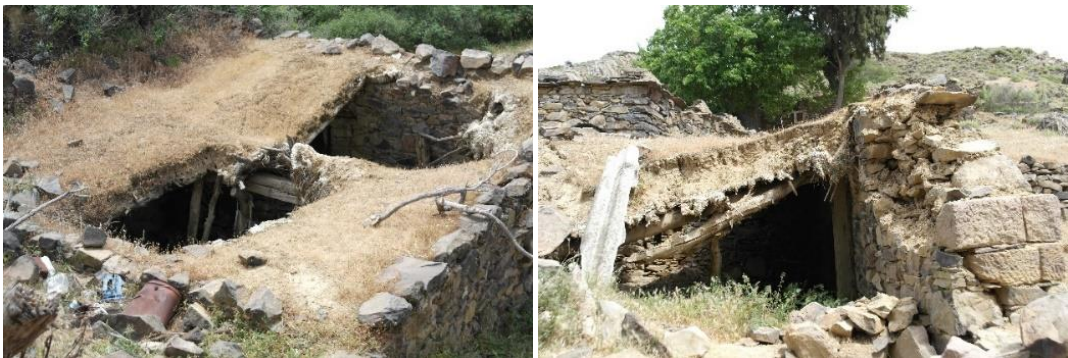
Figure 4.54. Flat Roof Examples in Küçükbahçe (April 2017).
