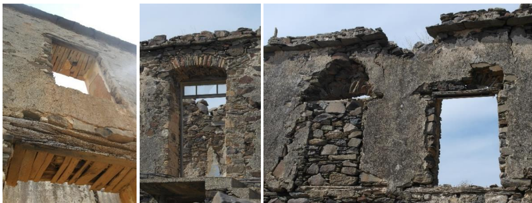
Figure 4.19. Spanning opening examples in Salman (October 2016).
