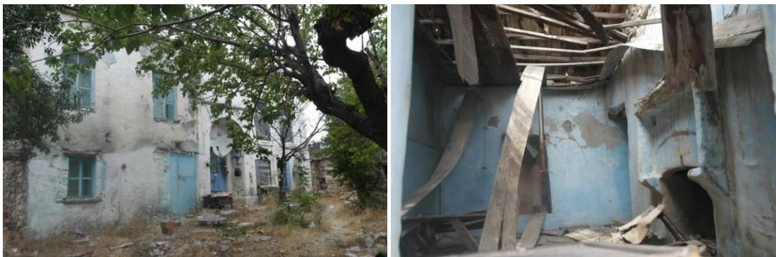
Figure 4.11. Plastered and Lime-washed Examples in Kösedere (June 2016).
