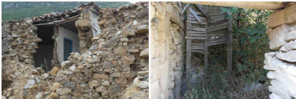
Figure 4.28. Timber Frame Wall in (a) Ambarseki (b) Tepeboz (June 2016).
