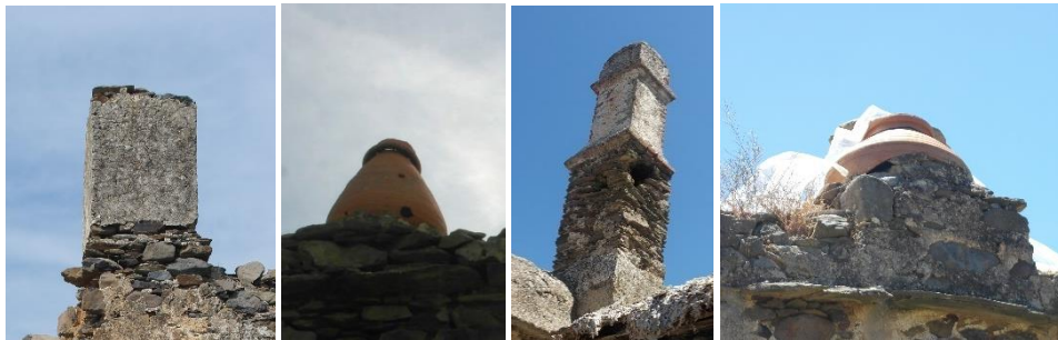
Figure 4.97. Chimney Examples in Salman (May 2017).
