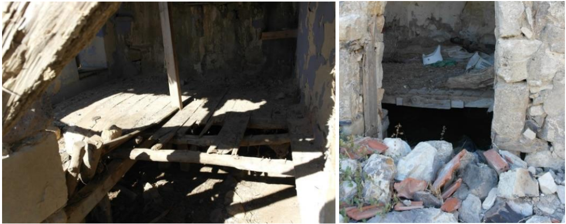
Figure 4.39. Floor Construction (a) Bozköy (b) Tepeboz (June 2016)
