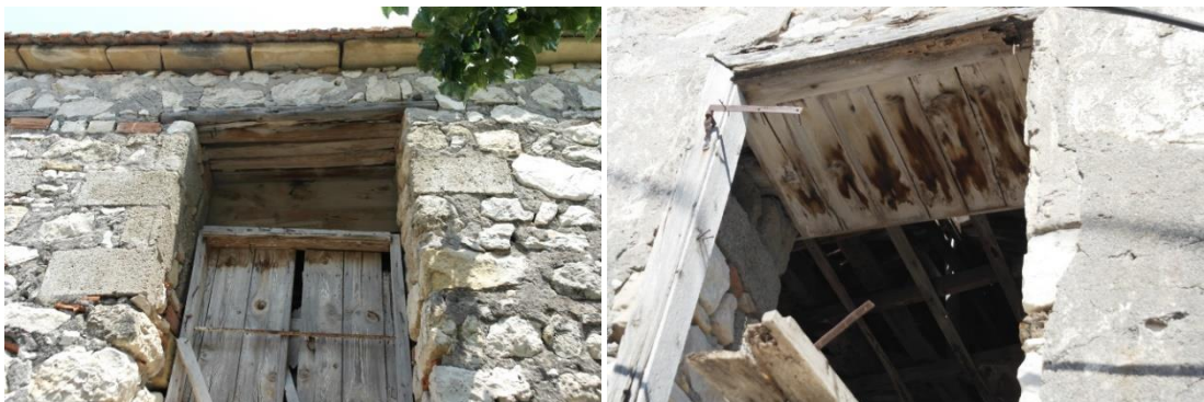
Figure 4.22. Spanning Openings in İncelik (April 2017).
