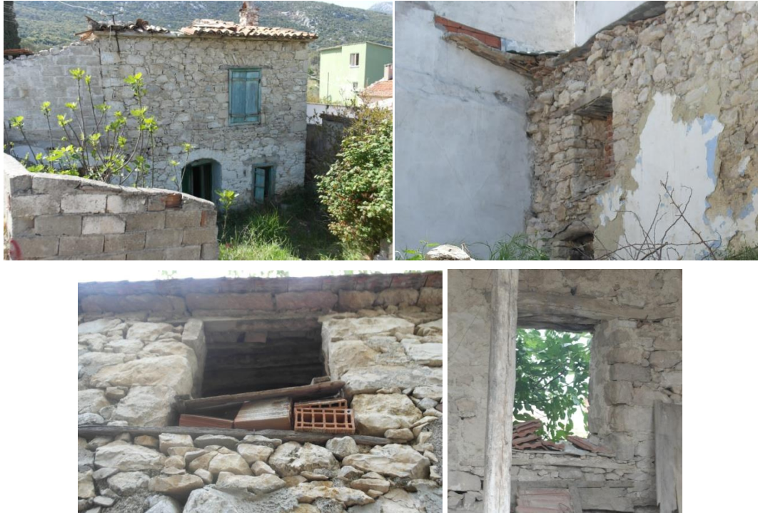
Figure 4.17. Spanning Openings in Kösedere (June 2016).
