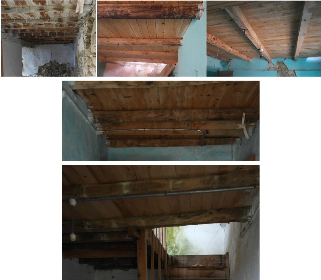
Figure 4.41. Floor Construction in Küçükbahçe (April 2017).
