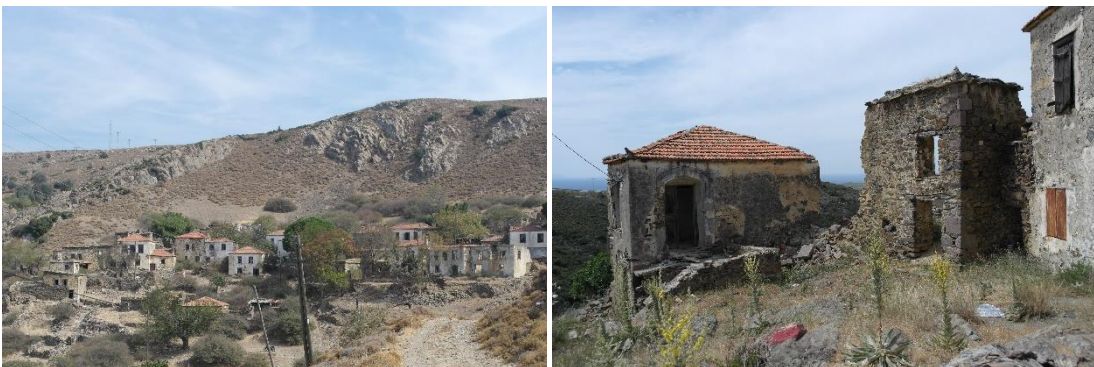
Figure 4.48. Hipped and Pitched Roof Examples in Küçükbahçe (April 2017)
