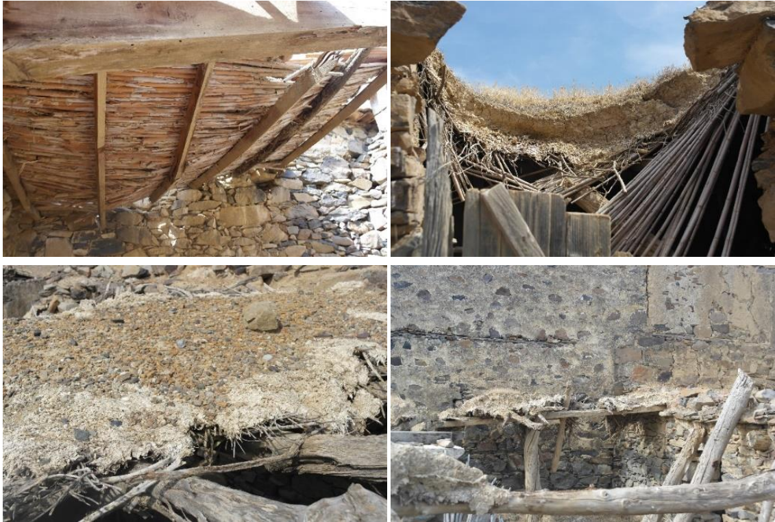
Figure 4.55. Flat Roof Examples in Küçükbahçe (April 2017).
