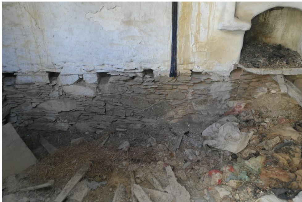
Figure 4.37. Raised Ground Flooring System Trace in Salman (May 2017).
