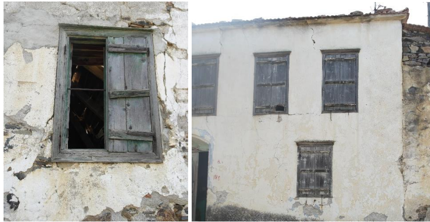
Figure 4.74. Shutter Examples in Küçükbahçe (October 2016).
