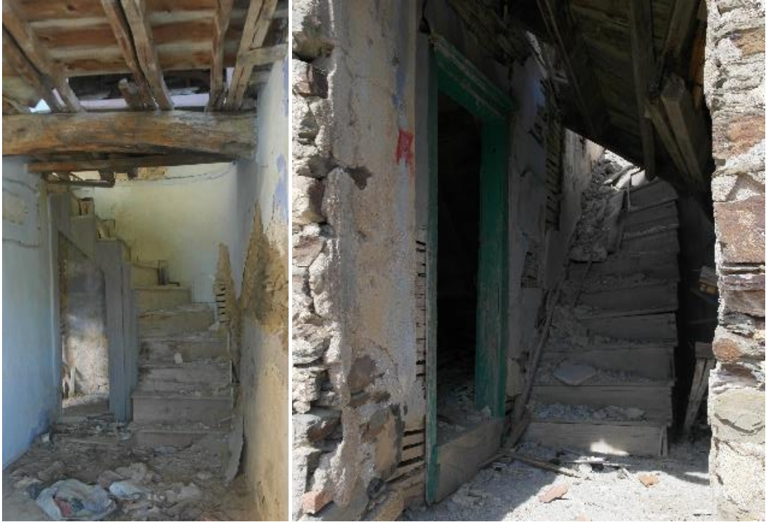
Figure 4.88. Timber Stair Examples in Salman (May 2017).
