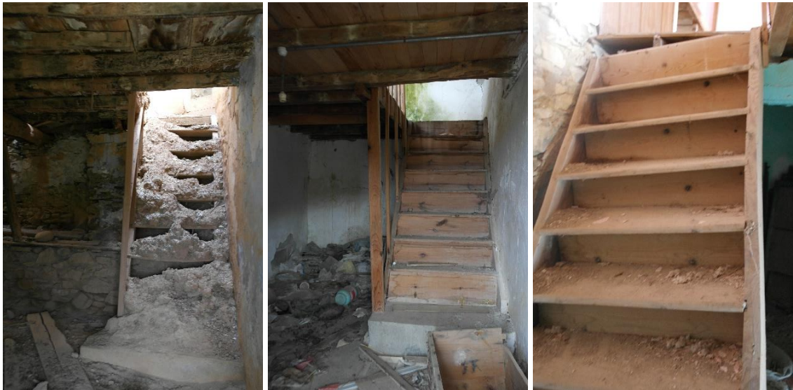
Figure 4.85. Timber Stair Examples in Küçükbahçe (June 2017).
