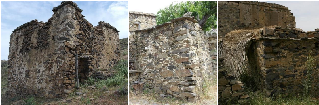
Figure 4.5. Overlapping Stones at the corners in Küçükbağçe (April 2017).
