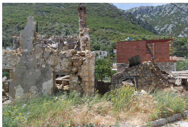
Figure 1.1. Disappearing structures in Ambarseki (May 2017).
