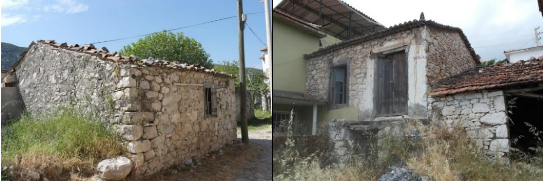
Figure 4.46. Examples of Pitched Roofs in Kösedere (June 2016).
