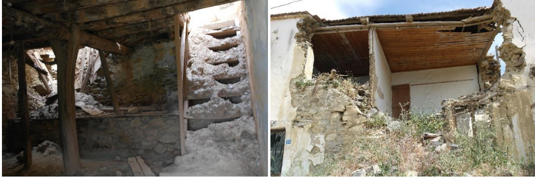
Figure 4.45. Ground Floor and First Floor Ceiling Structures in Küçükbahçe (April 2017).
