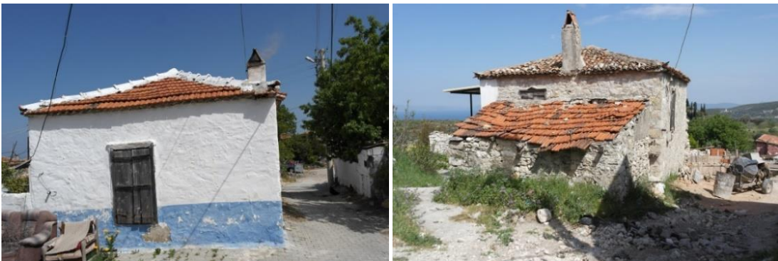
Figure 4.47. Examples of Hipped Roofs in Kösedere (June 2016).
