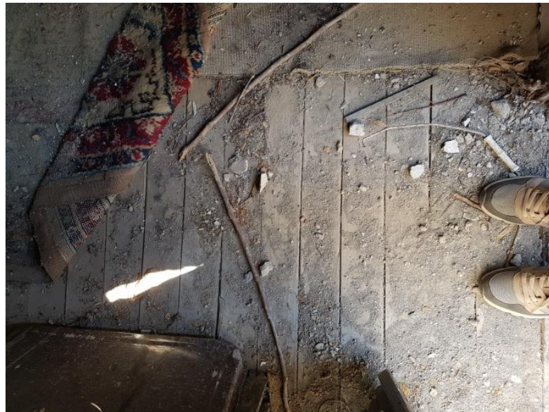
Figure 4.35. Wood Panel Covering Example on Ground Floor in İncik (June 2017).
