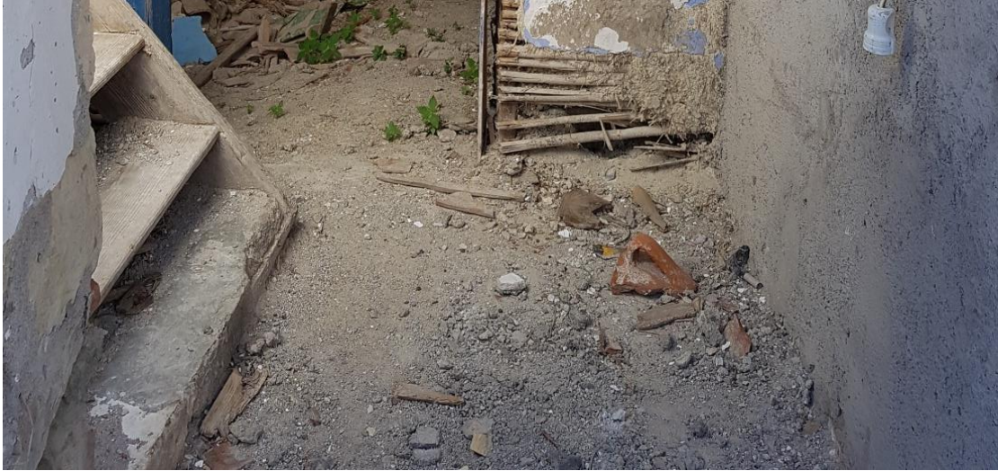
Figure 4.34. Pressed Earth Floor Pavement Example on Ground Floor in İncik (June 2017).
