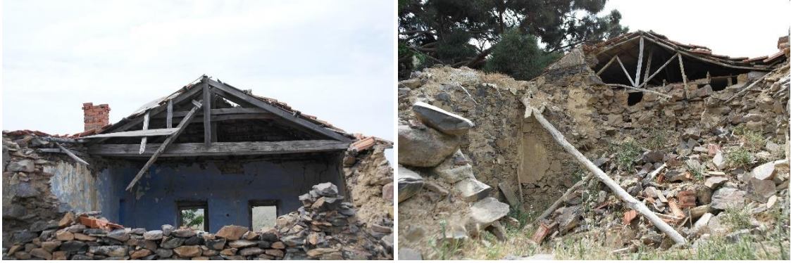
Figure 4.49. Hipped and Pitched Roof Examples in Küçükbahçe (April 2017).
