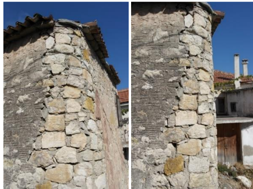
Figure 4.7. Chamfered Corner in Eğlenhoca (October 2016).
