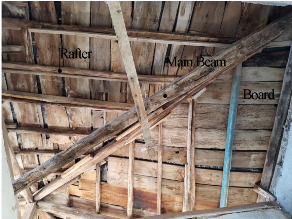
Figure 4.50. Hipped Roof Components in İncelik (June 2017).
