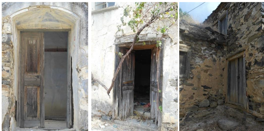
Figure 4.62. Entrance Doors Examples in Küçükbahçe (April 2017).
