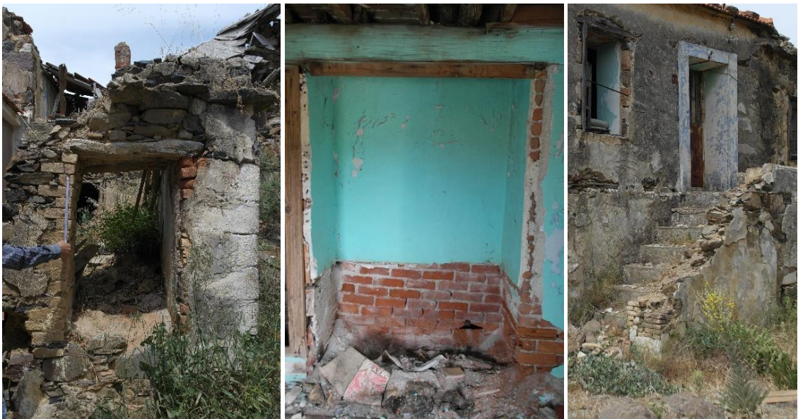
Figure 4.24. Brick usage examples in Küçükbahçe (April 2017).
