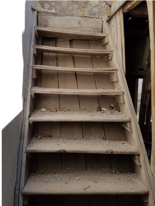
Figure 4.86. Timber Stair Example in İncik (June 2017)
