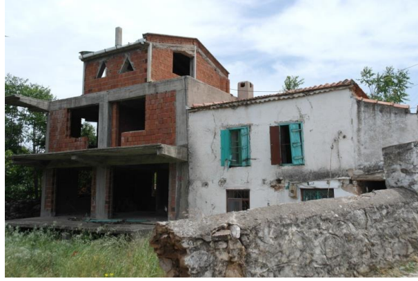
Figure 1.5. Old and new structure relation in Saip (May 2017).
