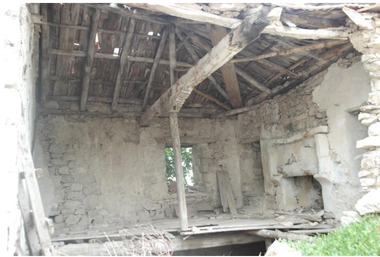
Figure 4.32. Wooden Post Carrying the Main Beam of the Roof in Kösedere (2016).
