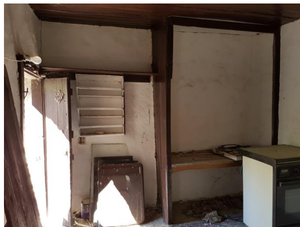
Figure 4.103. Example of Cupboard in İncelik; (June 2017).
