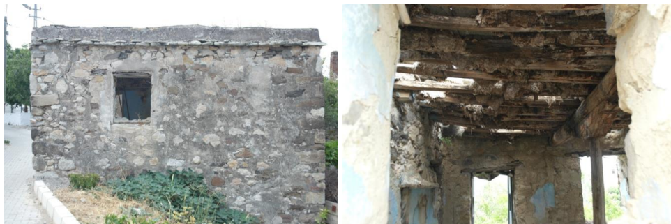
Figure 4.52. Flat roof examples in Saip (June 2016).
