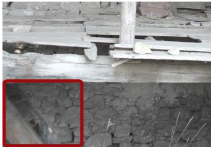
Figure 4.84. The Only Timber Stair Observed in Kösedere (June 2016).
