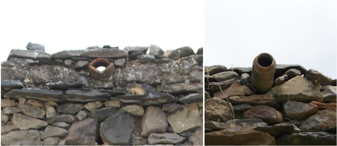
Figure 4.114. Waterspout Examples in Yayla (April 2017).
