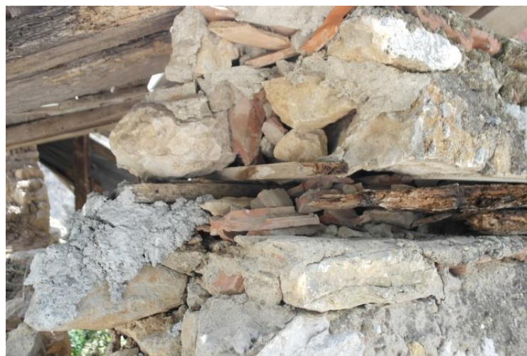
Figure 4.9. Lintel Overlapping at Corner in Ambarseki (April 17).
