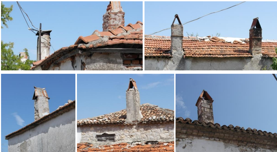
Figure 4.94. Chimney Examples in Kösedere (June 2016).
