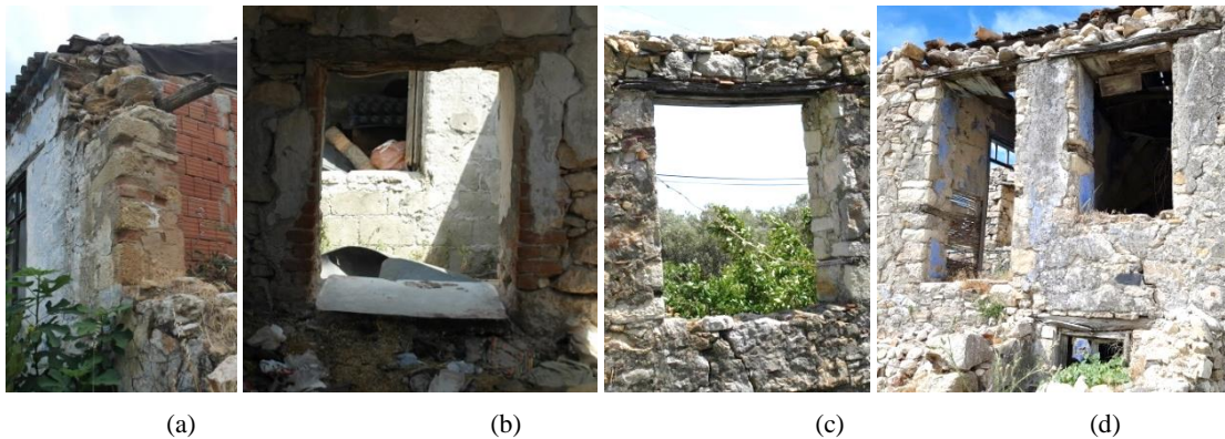
Figure 4.16. Brick and wood usage for openings in (a) Kösedere (b) Eğlenhoca (c) Ambarseki (d) Tepeboz (April 2017).
