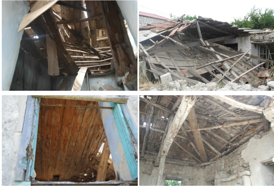
Figure 4.43. Ceiling Structure Examples in Kösedere (June 2016).
