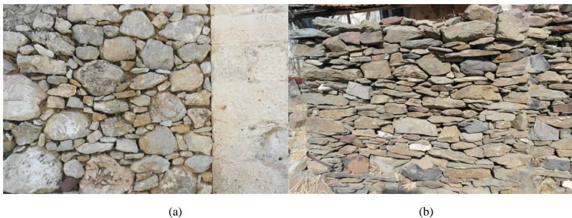
Figure 3.27. (a) White and yellowish color and round form stone from Ambarseki, (b) Thin, flat and gray-black color stone from Salman.
