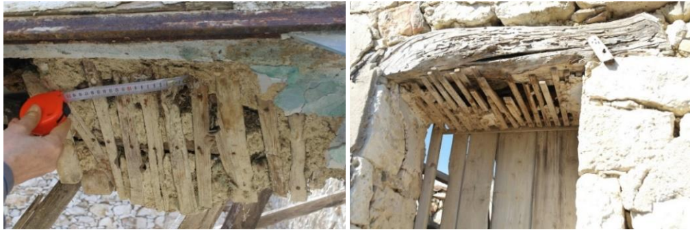
Figure 4.20. Spanning Openings in Eğlenhoca (March 2017).
