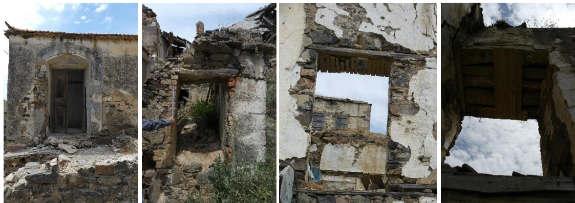
Figure 4.18. Spanning opening examples in Küçükbahçe (April 2017).
