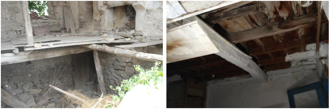
Figure 4.38. Floor Construction (a) Kösedere (June 2016) (b) İncecik (November 2016)
