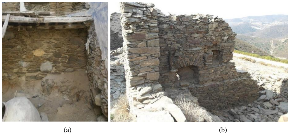
Figure 4.2. Stone masonry foundation (a) in Salman (By author, May 2017), (b) Sazak (October 2016).
