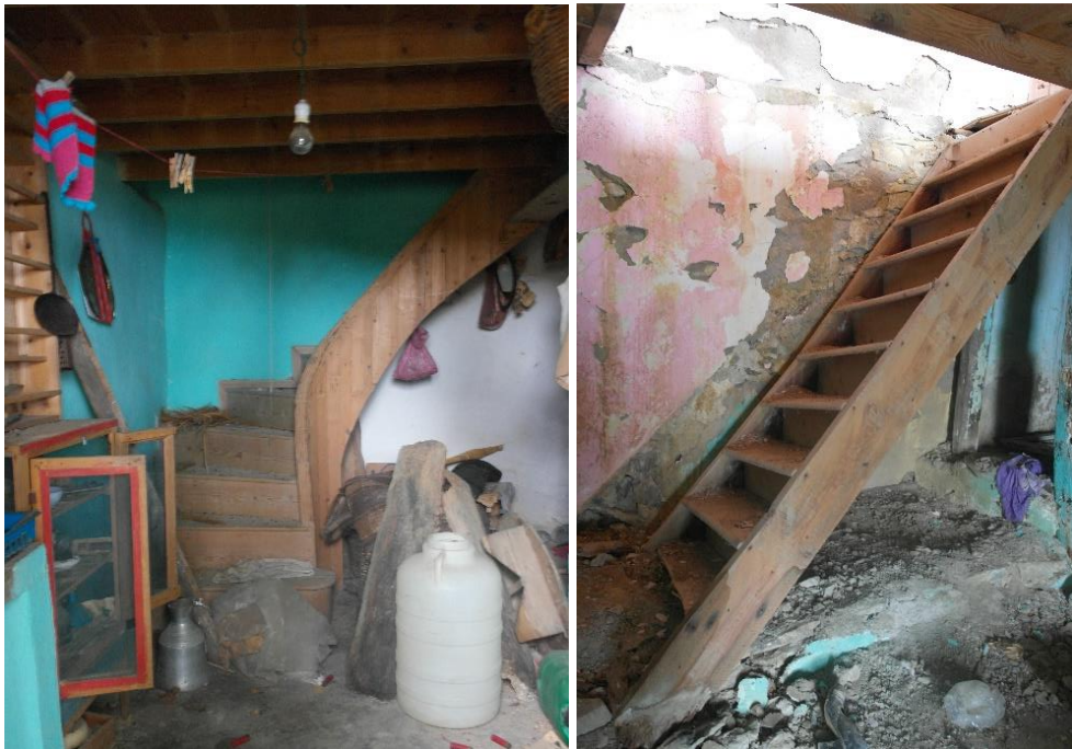
Figure 4.87. Timber Stair Examples in Küçükbahçe (November 2014)
