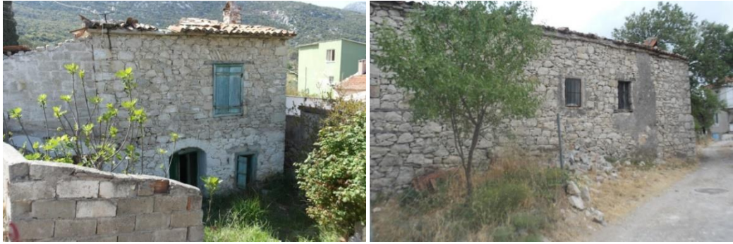
Figure 4.12. Non-Plaster and Lime-washed Examples in Kösedere (April 2017).
