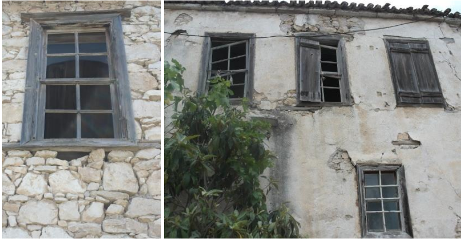
Figure 4.68. Sash Window Examples in Kösedere (June 2016).
