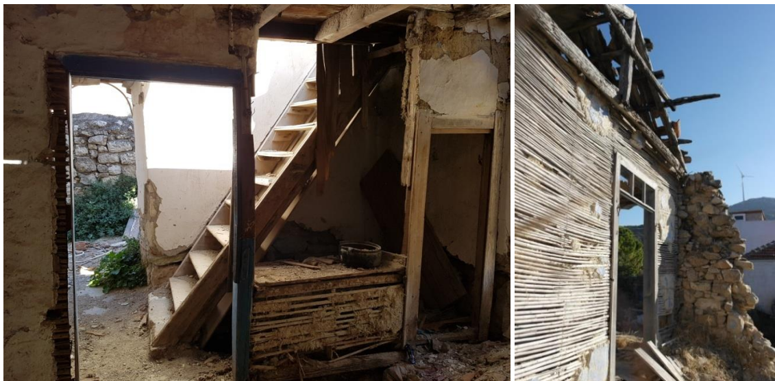
Figure 4.65. Doors in Timber Framed Wall (a) İncecik (b) Tepeboz (June 2016).
