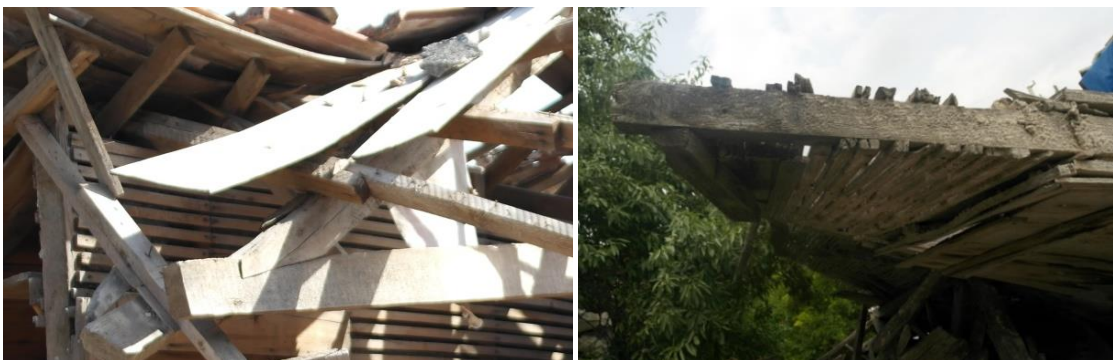
Figure 4.26. Timber Framed Wall Examples in Kösedere (June 2016).
