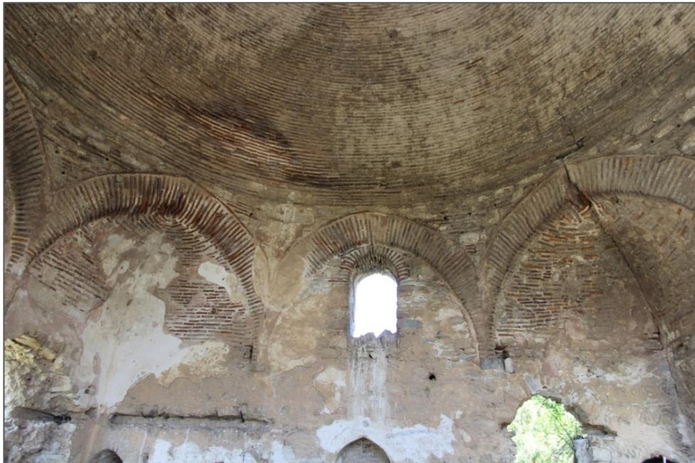
Figure 3.20. Squinches, arch and pendentives on transition zone of north wall
