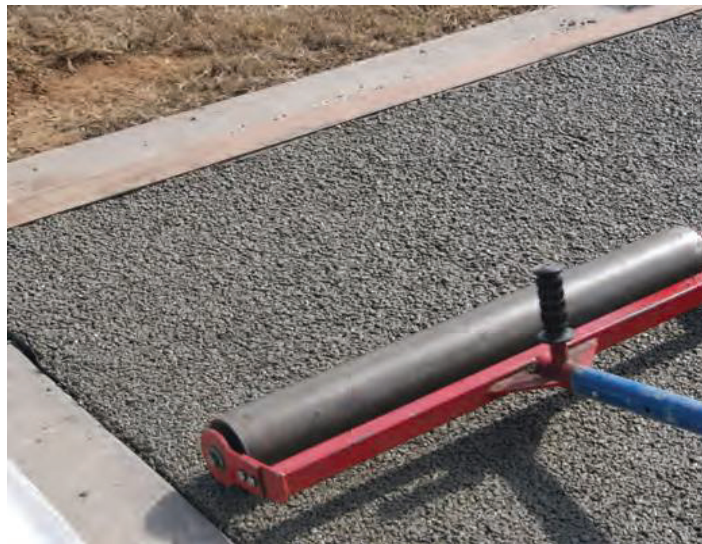
Figure 2.14 Compaction of pervious pavement (Source: [6])
