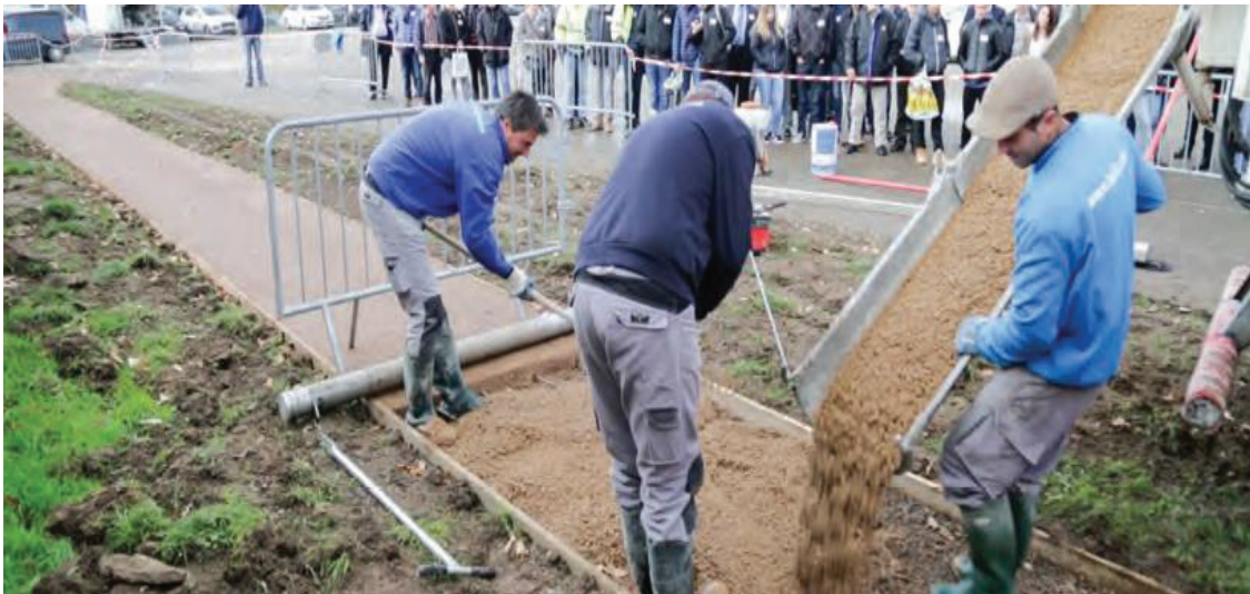
Figure 2.12 Placement of pervious concrete (Source: [6])
