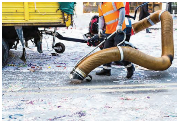
Figure 2.17 Cleaning of pervious concrete by vacuuming (Source: [6])
