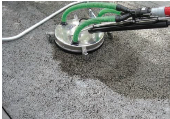
Figure 2.16 Cleaning of pervious concrete by vacuuming (Source: [6])
