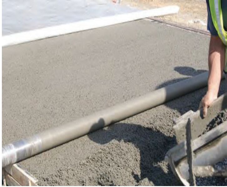
Figure 2.13 Compaction of pervious pavement (Source: [6])
