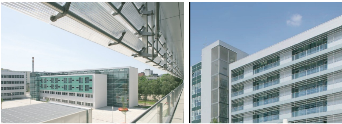
Figure 2.8. An example of movable prism system application in hospital building in Linz, Austria (Source: Siteco 2017)
