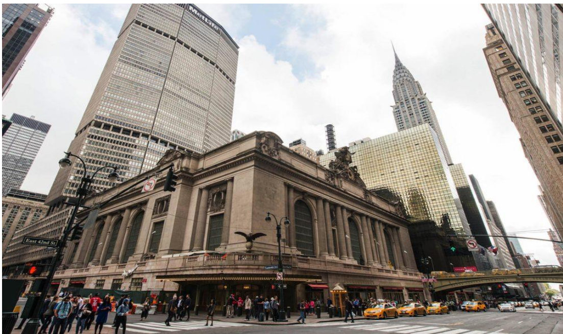
Figure 5.7. Grand Central Terminal in 2012
