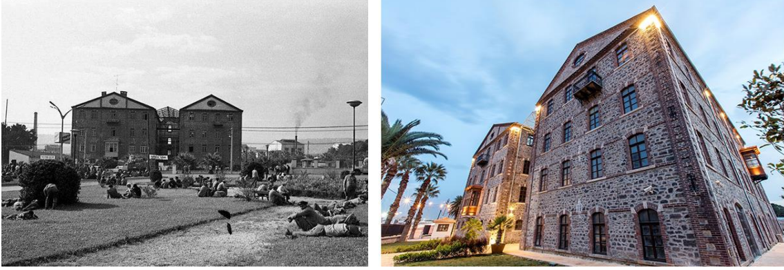
Figure 38. The historical photo (at the left) from Halkapınar Tuzakoğlu Flour Factory and the current photo (at the right) from Halkapınar Tuzakoğlu Flour Factory (Source. İzmirmag, 2019)
