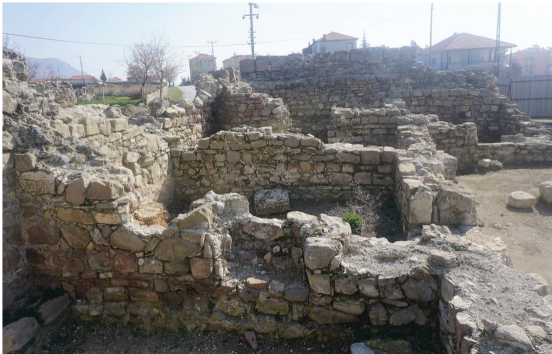
Figure 3.15. The interior walls of the service spaces at the north
