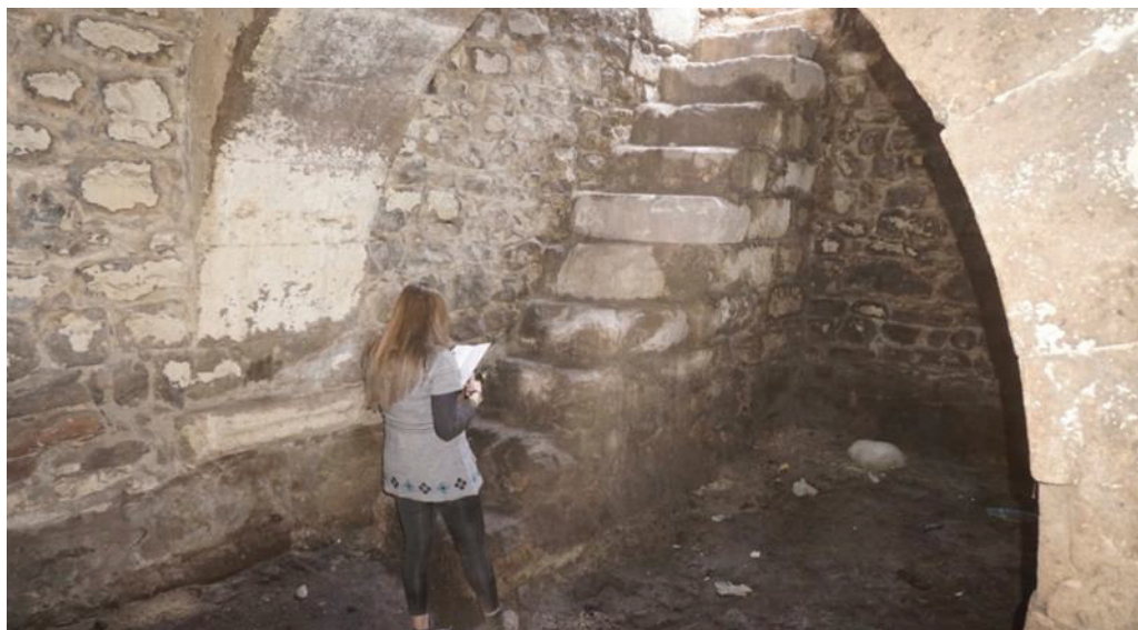
Figure 3.17. The staircase at the southeast corner of the shelter
