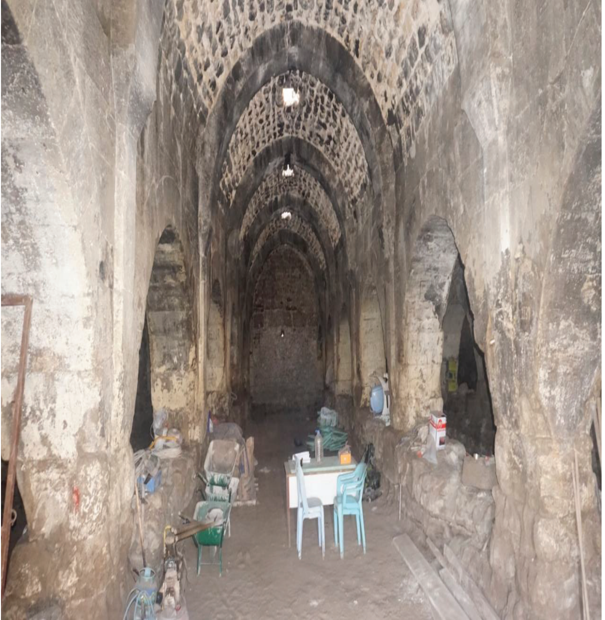
Figure 3.7. The central gallery as viewed from the east
