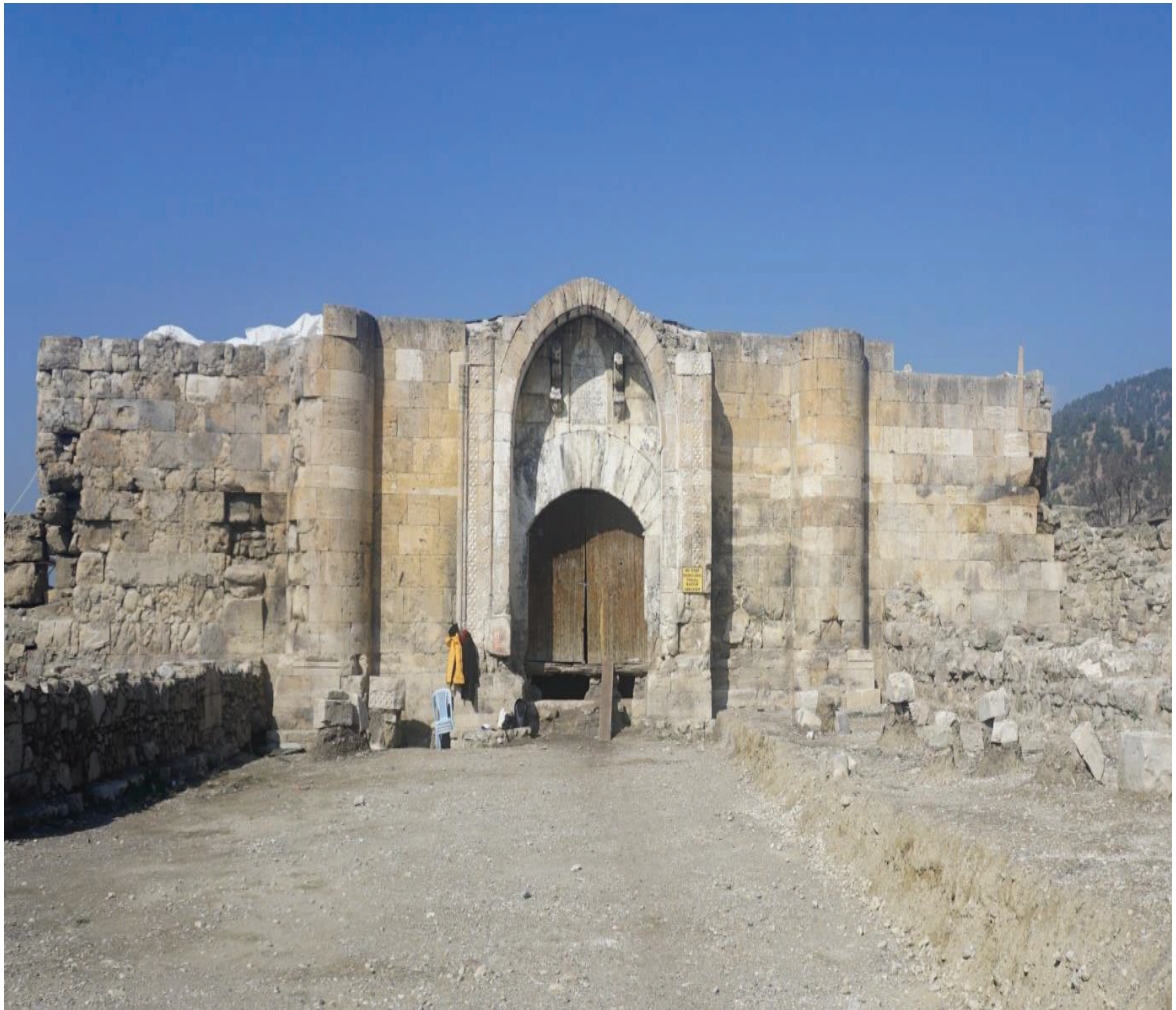
Figure 3.1. Çardak caravanserai in Denizli as viewed from the east
