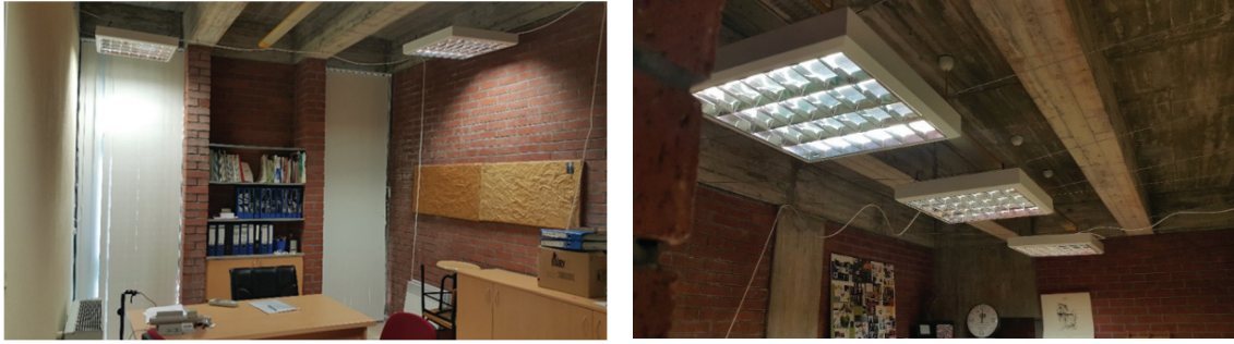
Figure 4.10. Installation of luminaires with fluorescent.
