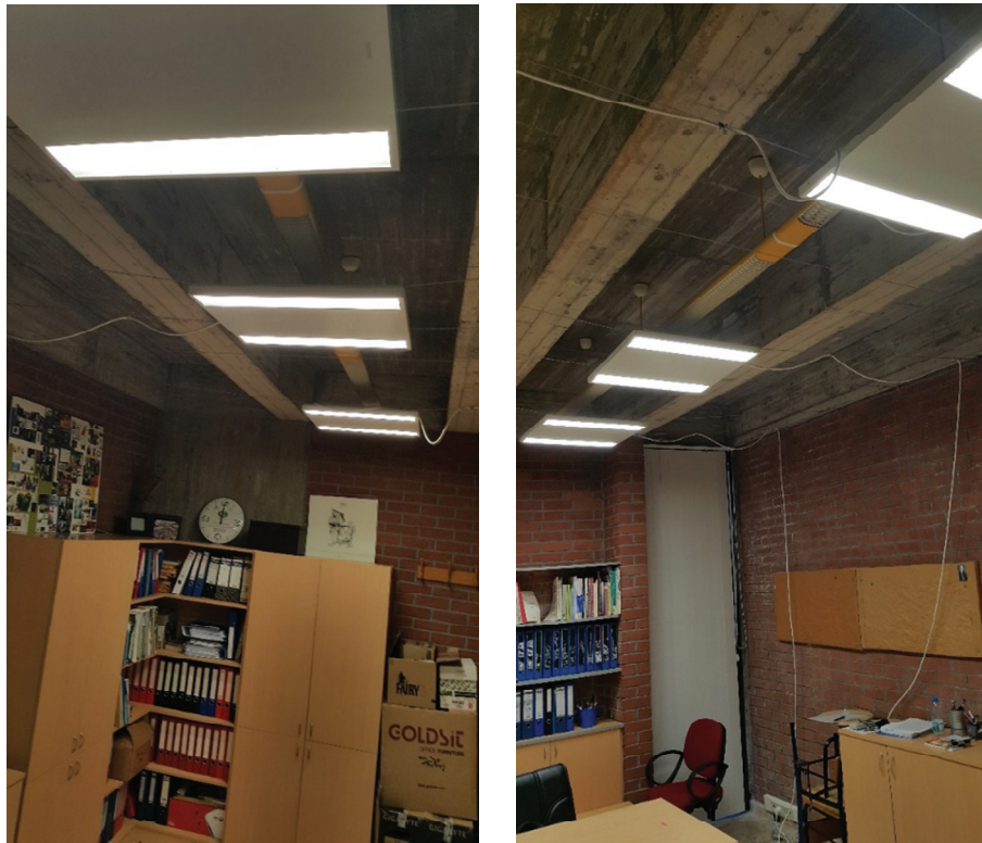
Figure 4.11. Installation of luminaires with LED.
