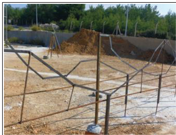
Figure 3.3 Metal Skeleton of Dam Site
