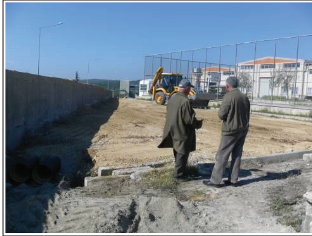
Figure 3.1 Construction of Model Site
