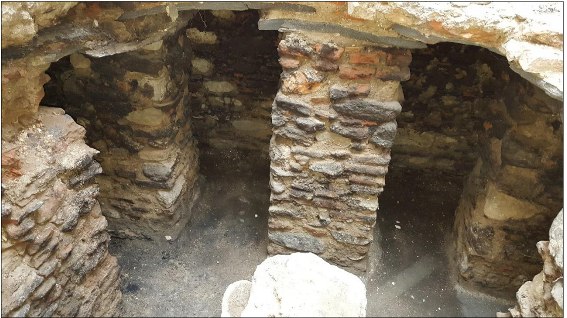
Figure A.62. Cehennemlik piers and the floor section (Source: Fatma Gürhan, July 2016)
