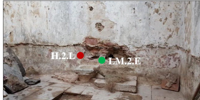
Figure 3.3. Locations where horasan plaster and lime mortar taken from the G02 Sıcaklık
