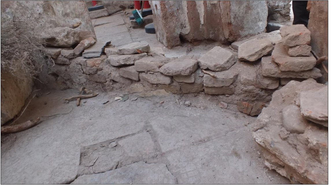
Figure A.64. The waste water channel formed with bricks between G02 Sıcaklık and G03 Sıcaklık (Source: Fatma Gürhan, November 2016)
