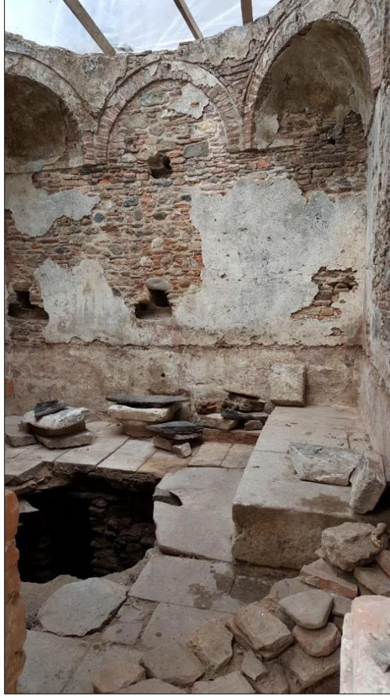
Figure 2.12. Eski Hamam G03 Sıcaklık (Source: Fatma Gürhan, December 2016)
