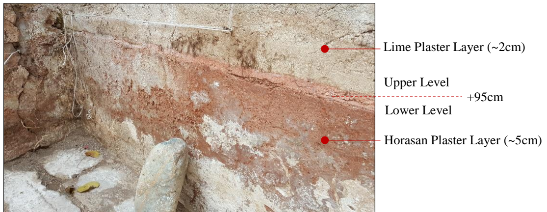
Figure 2.24. Plaster layers of the wall adjacent to the sıcaklık in the soyunmalık-ılıkık (15 th -16 th centuries)
