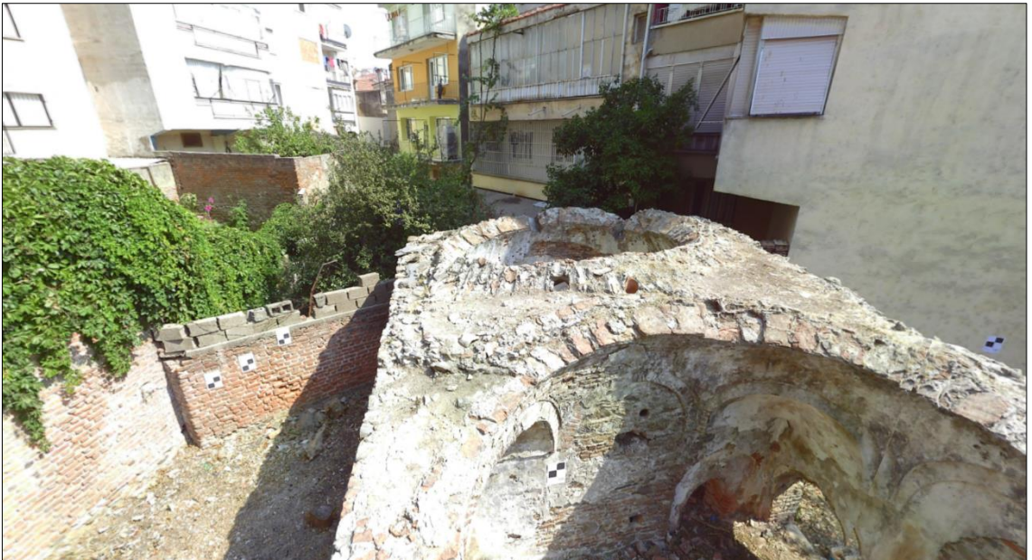
Figure A.68. The dome remain of the G03 Sıcaklık (Source: ANKA Architecture and Restoration Office archive, July 2016)
