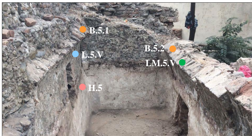
Figure 3.7. Locations where horasan plaster, lime plaster, building bricks and lime mortar taken from the G05 Hot Water Reservoir
