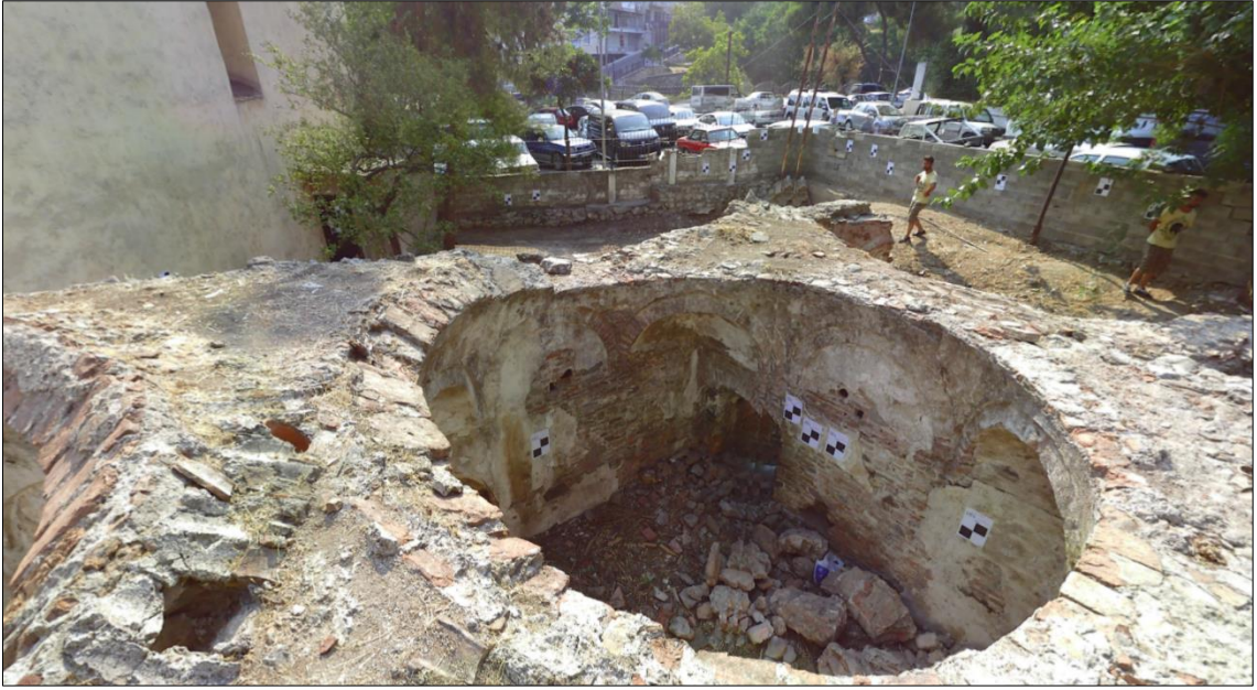
Figure A.67. The dome remain of the G03 Sıcaklık (Source: ANKA Architecture and Restoration Office archive, July 2016)
