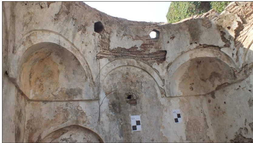
Figure A.50. The squinches and the pentagonal oculises (Source: Fatma Gürhan, July 2016)
