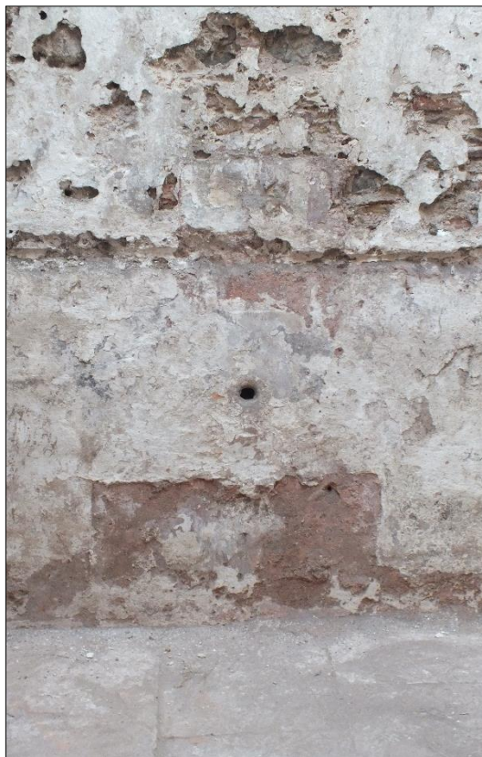
Figure A.48. Traces of the kurna and seki (Source: ANKA Architecture and Restoration Office archive, February 2017)
