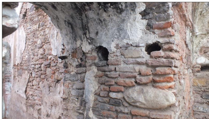
Figure A.66. The junction line between G03 Sıcaklık and G04 Sıcaklık and the interrupted terracotta pipes (Source: Mükerrerem Kürüm archive, May 2017)
