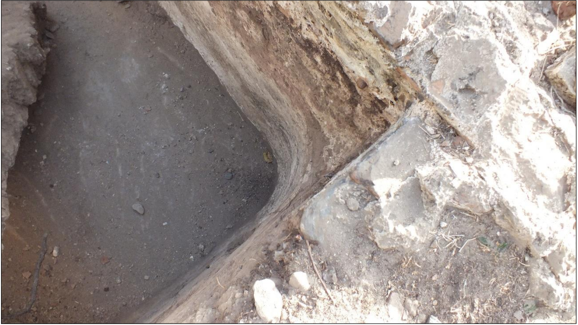
Figure A.81. Example of rounded corner with plaster (Source: ANKA Architecture and Restoration Office archive, October 2016)
