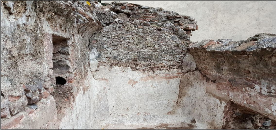
Figure A.79. The control window and the barrel vault remain (Source: Fatma Gürhan, December 2016)
