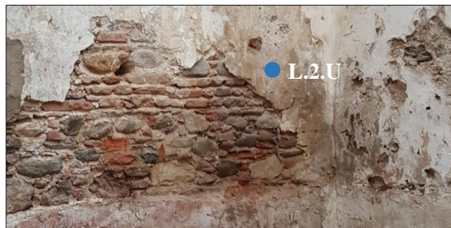
Figure 3.4. Location where lime plaster sample taken from the G02 Sıcaklık
