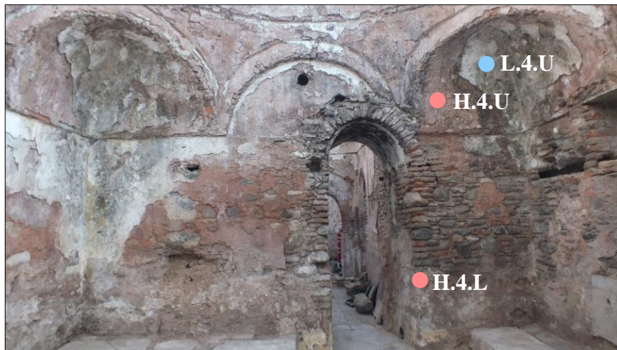
Figure 3.6. Locations where plaster samples taken from the G04 Sıcaklık
