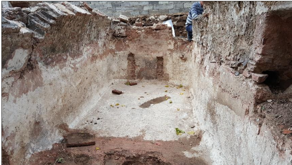
Figure 2.14. Eski Hamam G05 Hot Water Reservoir (Source: Fatma Gürhan, December 2016)
