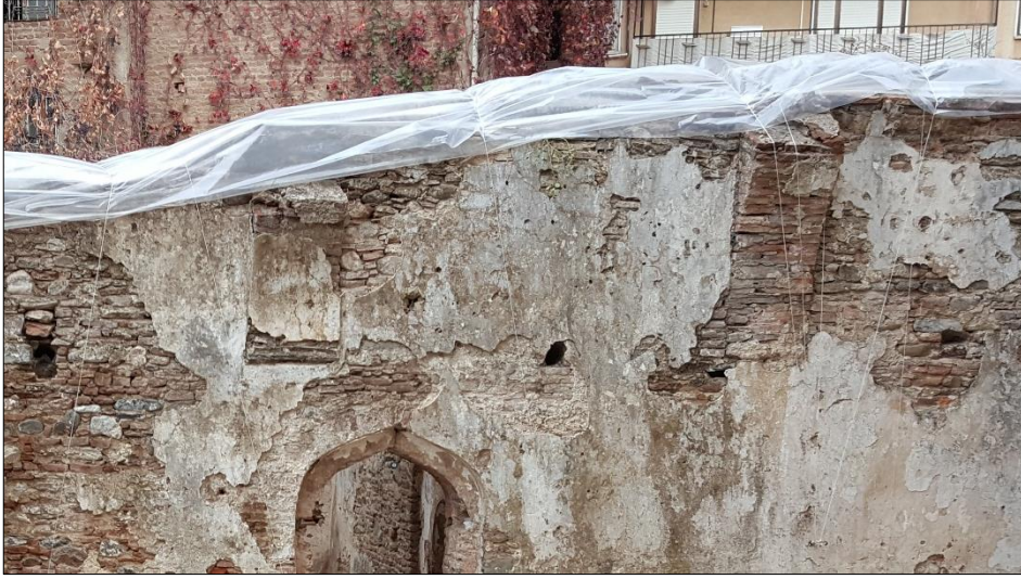
Figure A.37. The arch remains (Source: Fatma Gürhan, October 2016)
