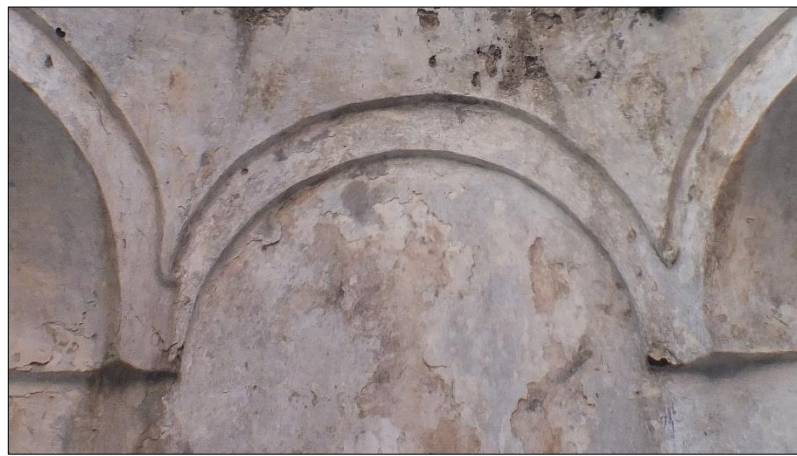
Figure A.52. The plaster motifs at the squinch finishes
