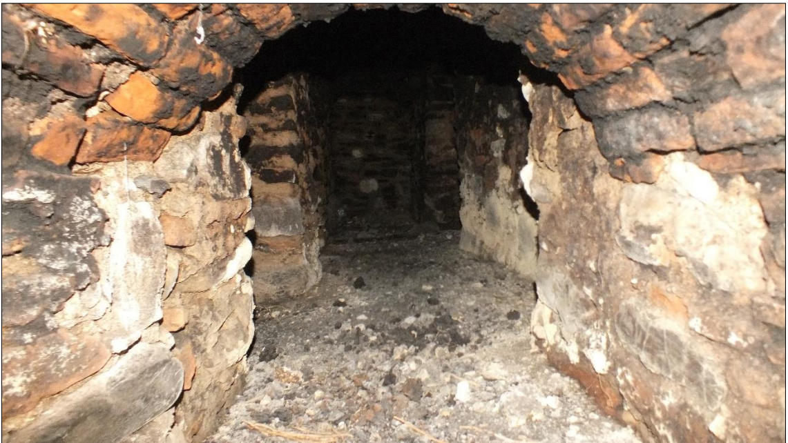
Figure A.55. Cehennemlik (Source: ANKA Architecture and Restoration Office archive, November 2016)
