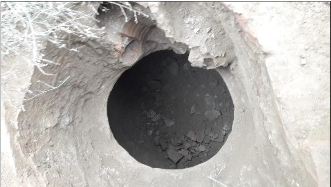
Figure A.88. The water reservoir of the fountain (Source: ANKA Architecture and Restoration Office archive, December 2016)
