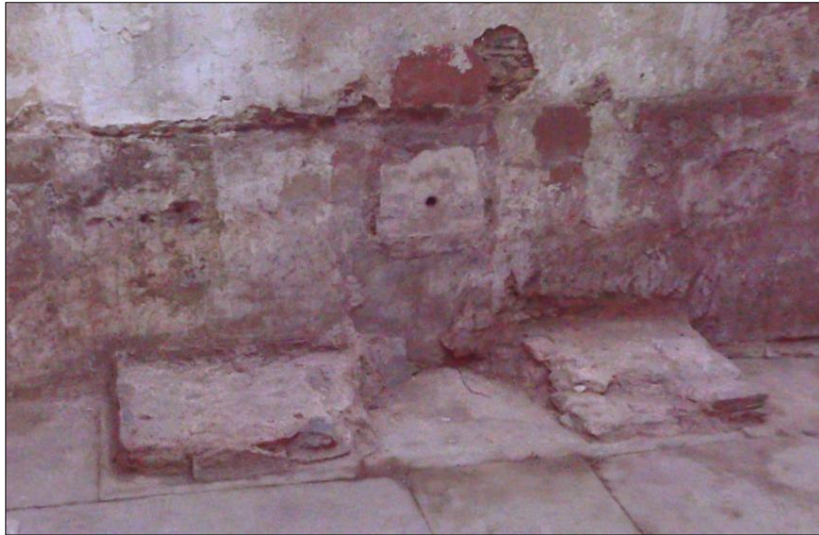
Figure A.47. Traces of the kurna and seki (Source: ANKA Architecture and Restoration Office archive, February 2017)
